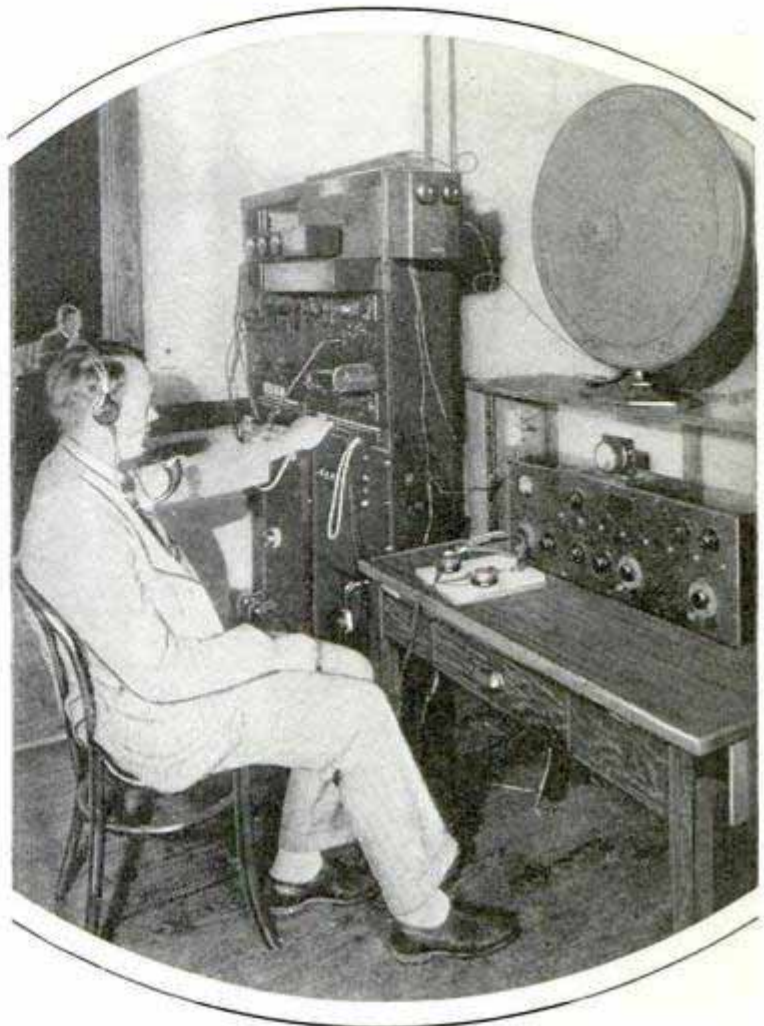
Terminal Equipment for Plane-to-Ground Transmitter at Airport Weather Station
