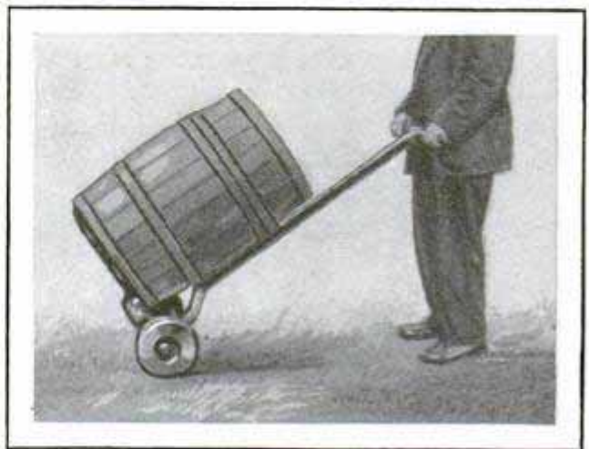
Old Lawnmower Converted into a Small Truck for Carrying Barrels
