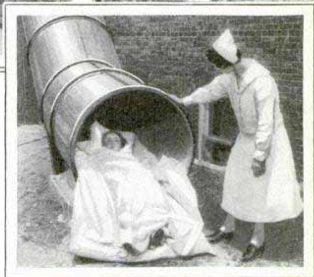
Tubular Fire Escape Which Protects from Fire, Water and Smoke; at Right, Hospital Patient Emerging from the Tube
