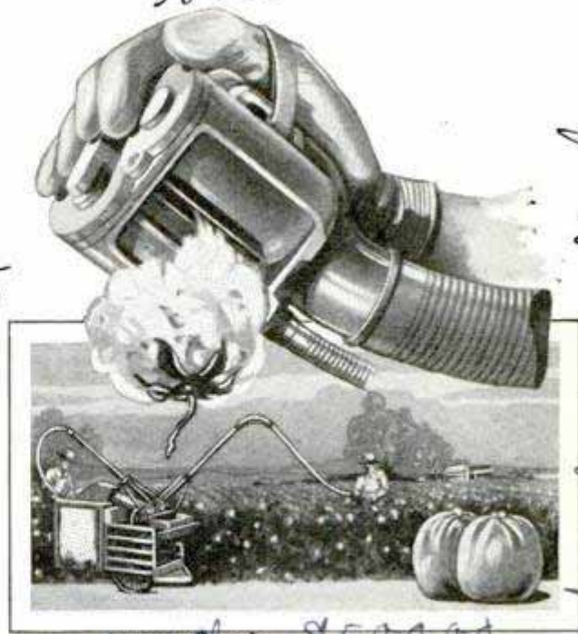
Cotton Picker Moved and Operated by One Man, and Close-Up of Picker Head
