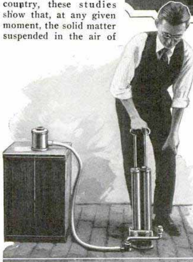
Making a Dust Count in Airplane over Washington, D. C., and Measuring Dust by "Paper Thimble"
