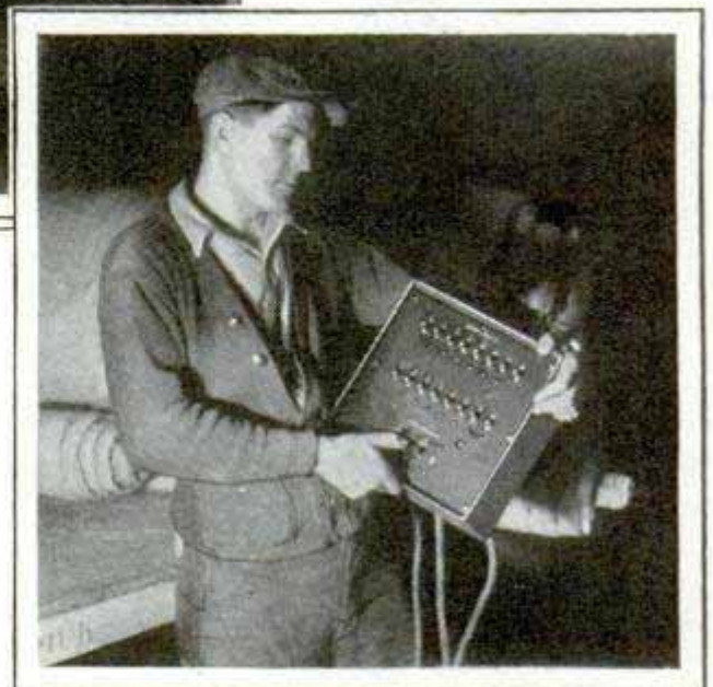
Views of the Light-Control Boards and the Portable Station for Raising and Lowering Stage Units
