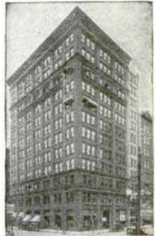
Our Pittsburgh Office Suite 514 Empire Building
