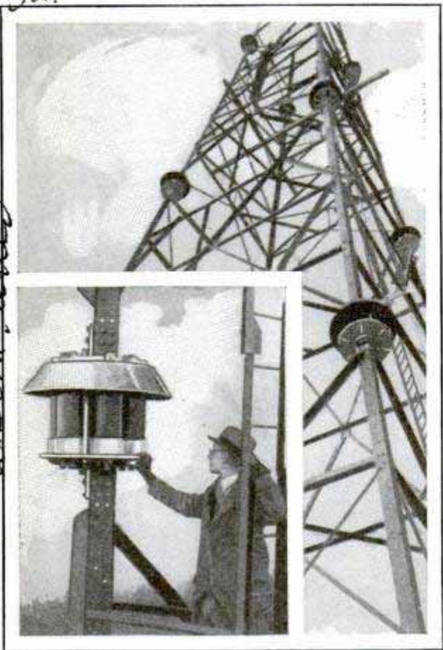
Radio Tower Built in Insulated Sections for Better Reception; Insert, One of the Insulators
