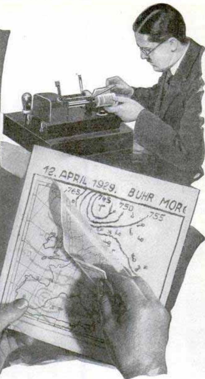
Left, Radio Weather Map as Received on Board "Graf Zeppelin" during Mediterranean Cruise; Right, "Fultograph" and Specimen British Weather Map It Broadcasts
