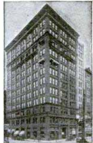
Our Pittsburgh Office Suite 514 Empire Building
