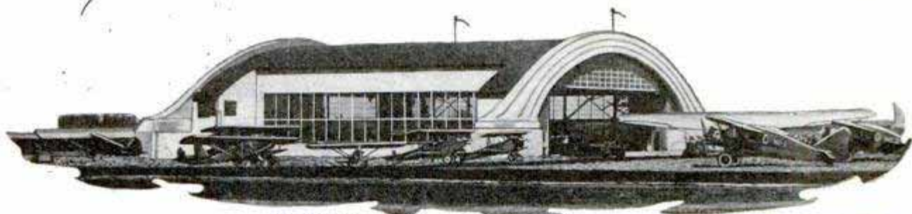
Steel and Concrete Hangar, Sky Harbor, Chicago
