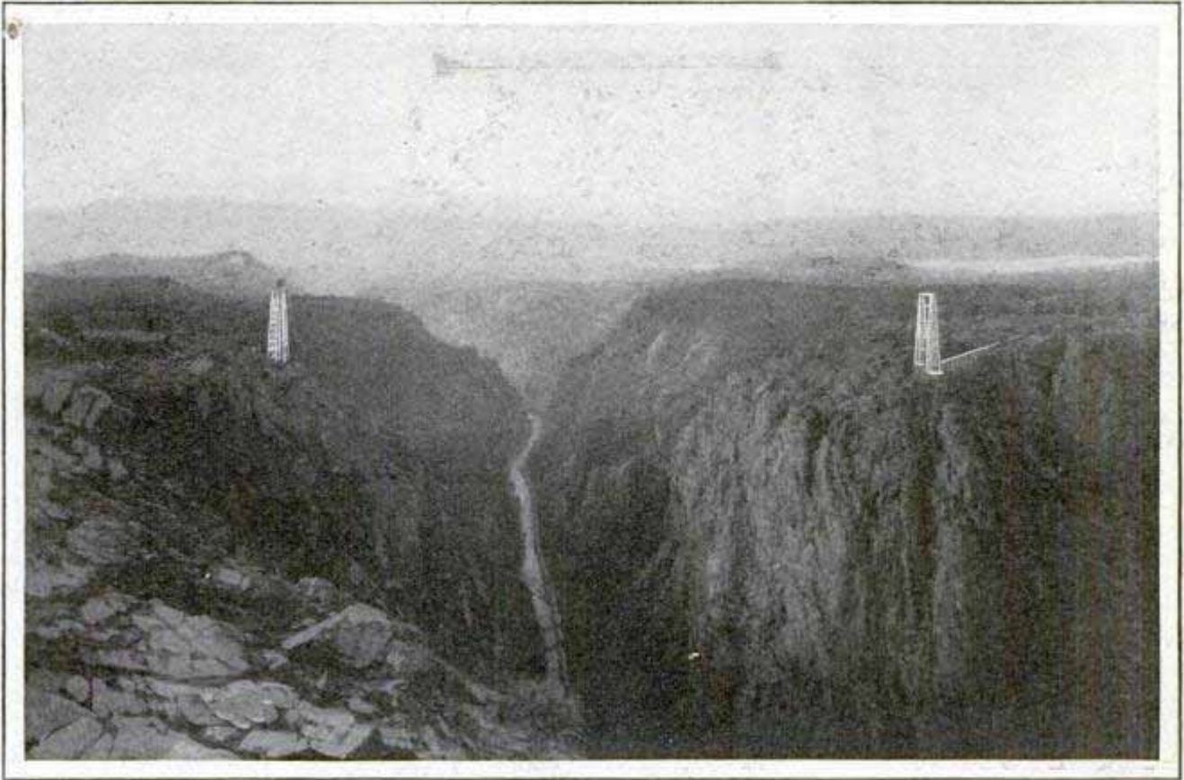
The Towers at Each Side of the Royal Gorge, on Which Will Rest the Highest Suspension Bridge in the World; It Will Be 1,052 Feet above the Arkansas River
