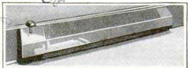
Floor-Level Radiator Installed, Showing How Closely It Fits to the Wall to Save Space
