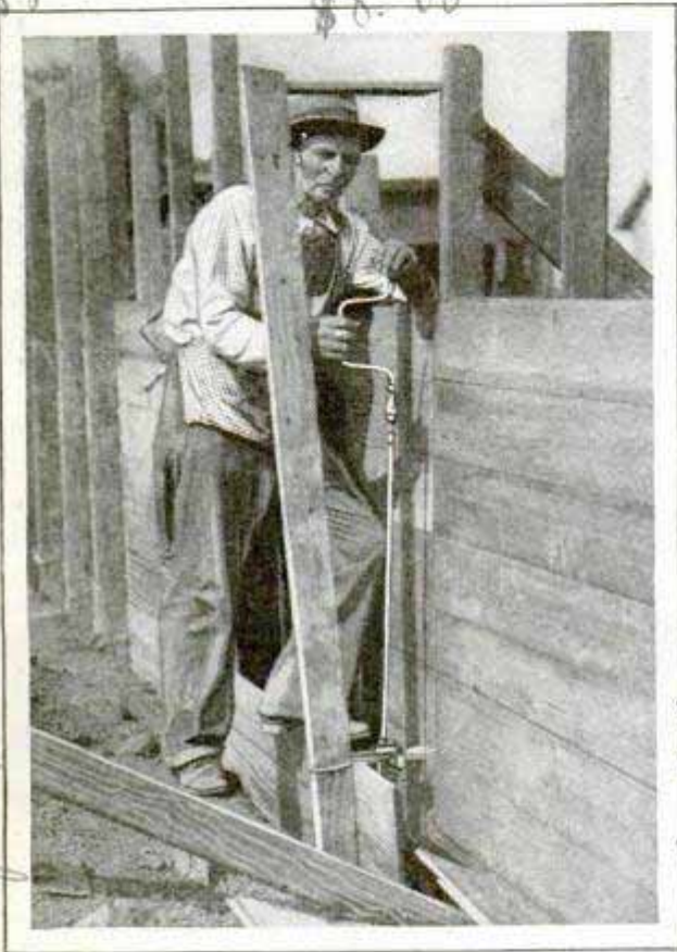
Wire Twister Operated like an Auger, to Tighten the Wires on Concrete Forms
