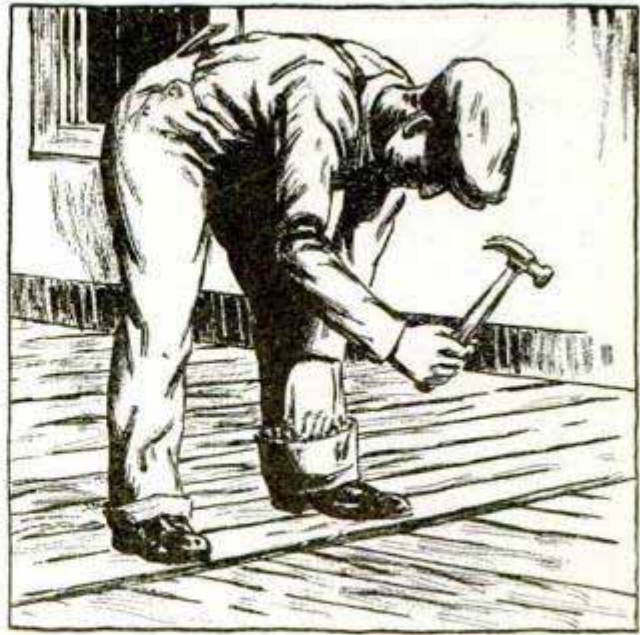
Extended Cuff on Carpenter's Trousers Makes Handy Nail Sack When Laying Flooring
