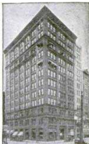
Our Pittsburgh Office Suite 514 Empire Building
