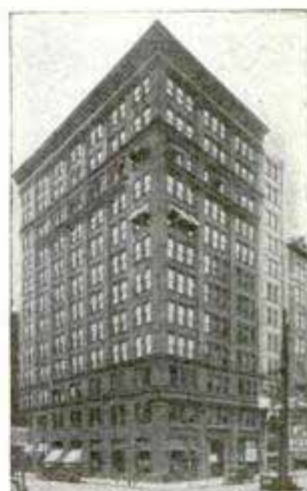
Our Pittsburgh Office Suite 514 Empire Building
