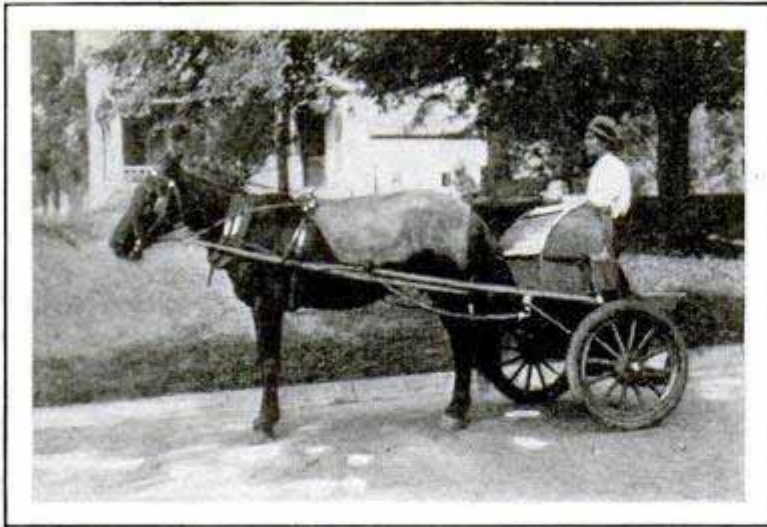
Cart Equipped with Old Auto Wheels and Casings Provides Comfort for the Driver
