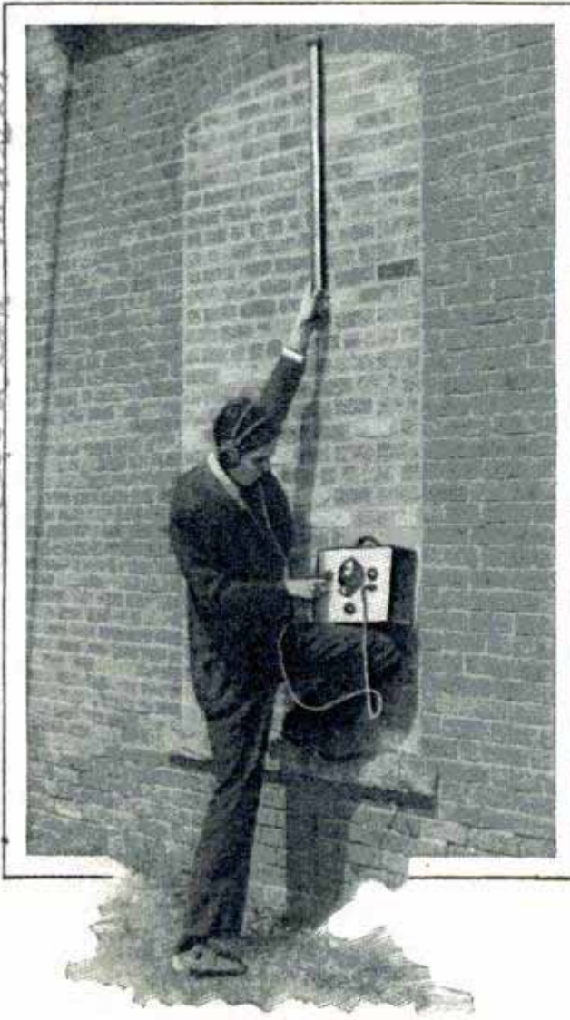
Tracking Down Radio Interference by Means of a Specially Designed Portable Receiver
