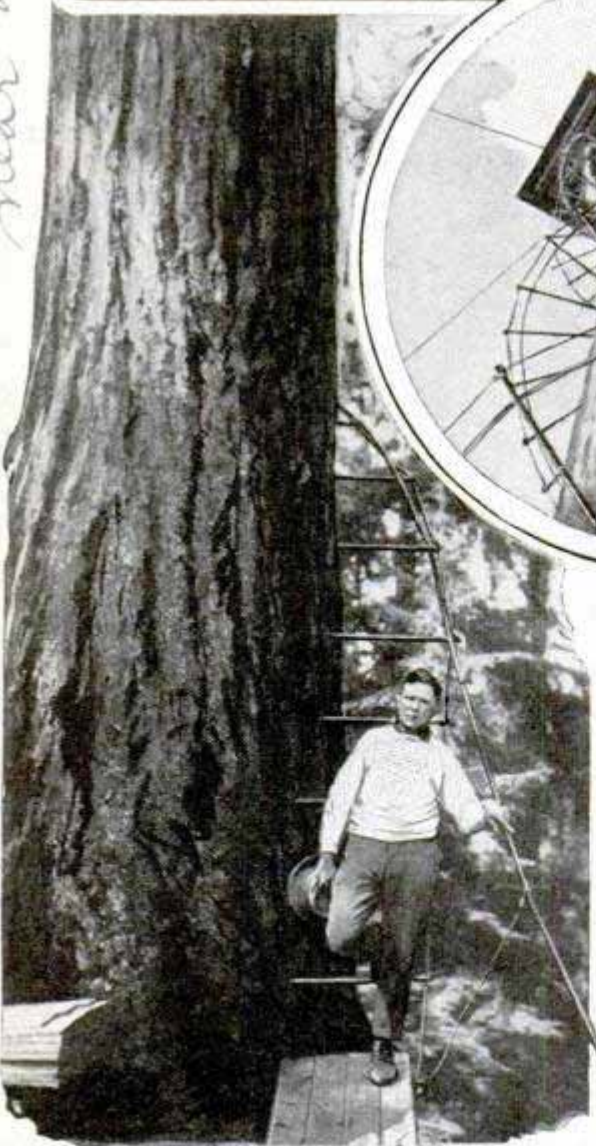
Miller at the Base of the Tree, Which Is Eight Feet in Diameter; Detail of the Ladder, a Spiral Series of Inch Steel Rods, Threaded with Steel Cable, and View of the Whole Lookout; the Tree Is Securely Guyed by Steel-Wire Ropes, Fastened Just below the House and Attached to Stumps near the Base; the Lookout Station Is Connected to a Fire Headquarters by Telephone; at the Observer's Command, a Speedy Gasoline Truck and Trailer, Loaded with Pumps, Hose and Tools, Are Dispatched to the Scene of a Blaze
