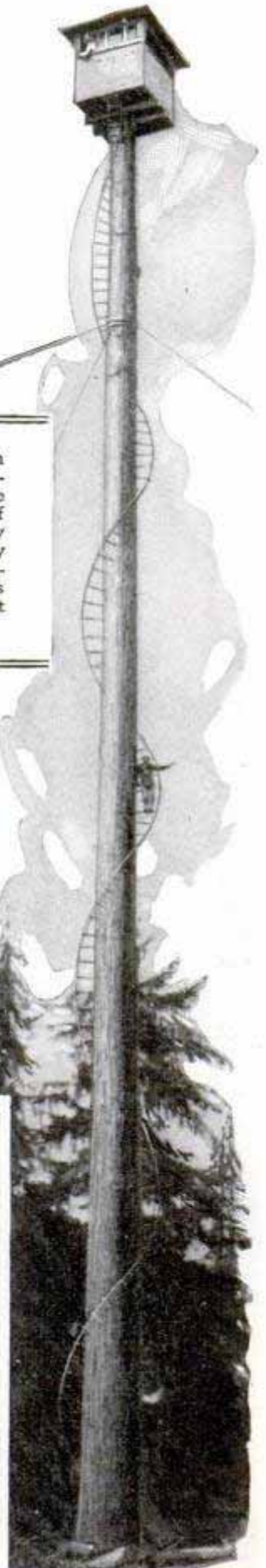
Miller at the Base of the Tree, Which Is Eight Feet in Diameter; Detail of the Ladder, a Spiral Series of Inch Steel Rods, Threaded with Steel Cable, and View of the Whole Lookout; the Tree Is Securely Guyed by Steel-Wire Ropes, Fastened Just below the House and Attached to Stumps near the Base; the Lookout Station Is Connected to a Fire Headquarters by Telephone; at the Observer's Command, a Speedy Gasoline Truck and Trailer, Loaded with Pumps, Hose and Tools, Are Dispatched to the Scene of a Blaze
