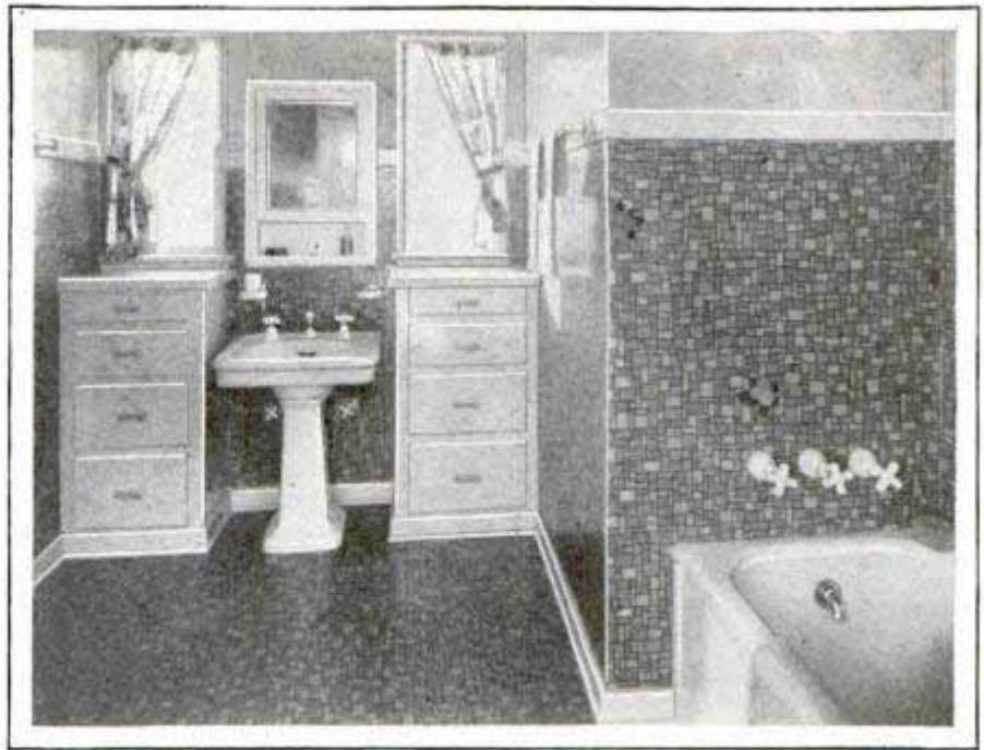
Inlaid Linoleum Used Instead of Tile for Wainscoting on Bathroom Wall; It Is Cheaper and Entirely Satisfactory
