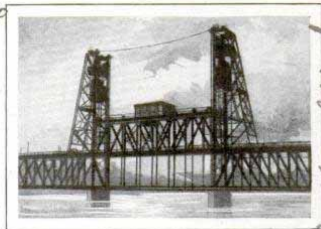
Twin-Deck Bridge at Portland, Oreg., So Arranged That Lower Level Can Be Raised Independently
