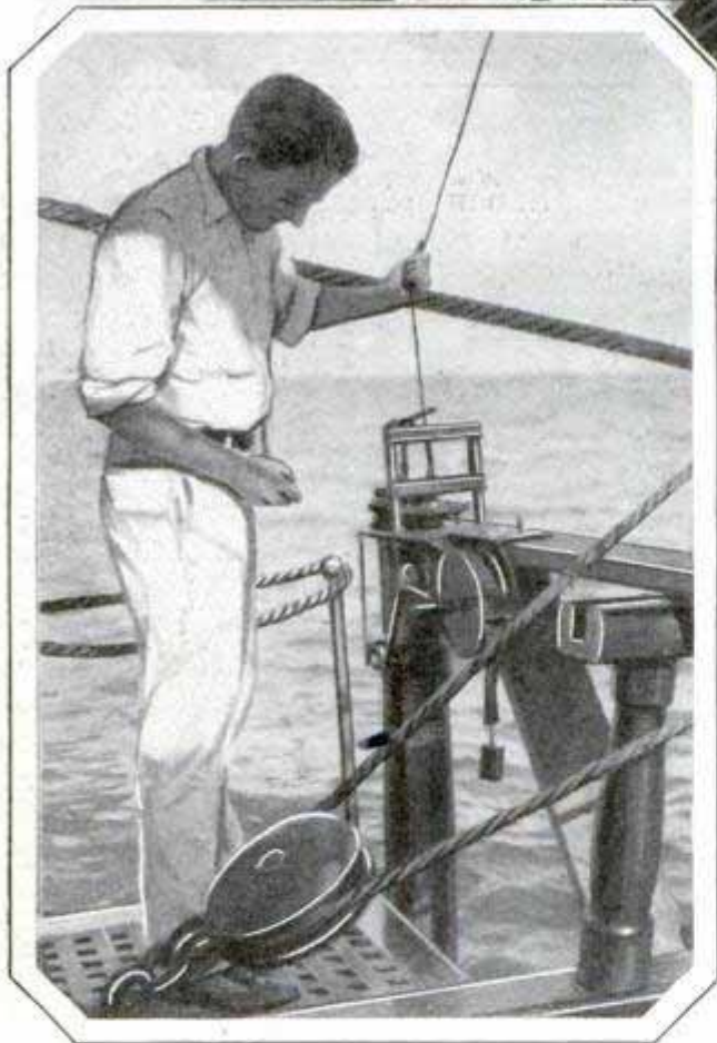
Captain Ault Inspecting the Non-Magnetic Electric Winch, Which Handles 20,000 Feet of Wire, and, Below, a Plankton Pump
