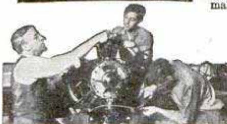
Students wiring and checking ignition on one of the late type Radial Aircraft Engines in our aviation electrical department
