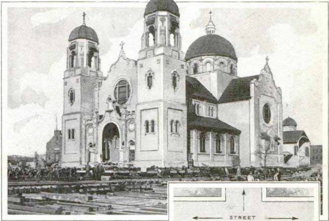
Chicago Church in Course of Being Moved across Street, and Diagram Showing Final Location
