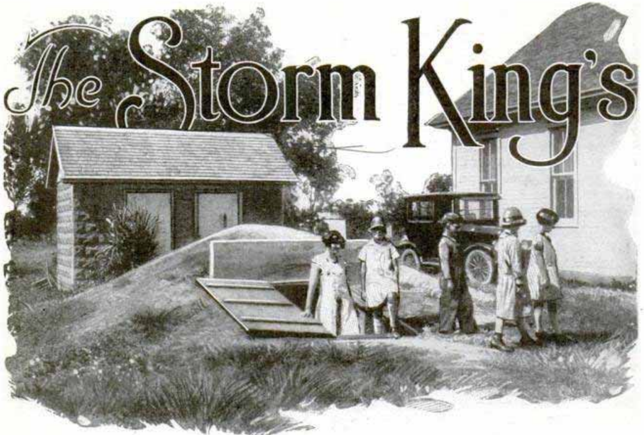
In Some of the Prairie States, Tornado Drill Is as Important as Fire Drill in the Schools; Here the Teacher Is Shepherding the Pupils Out of the Tornado Cellar
