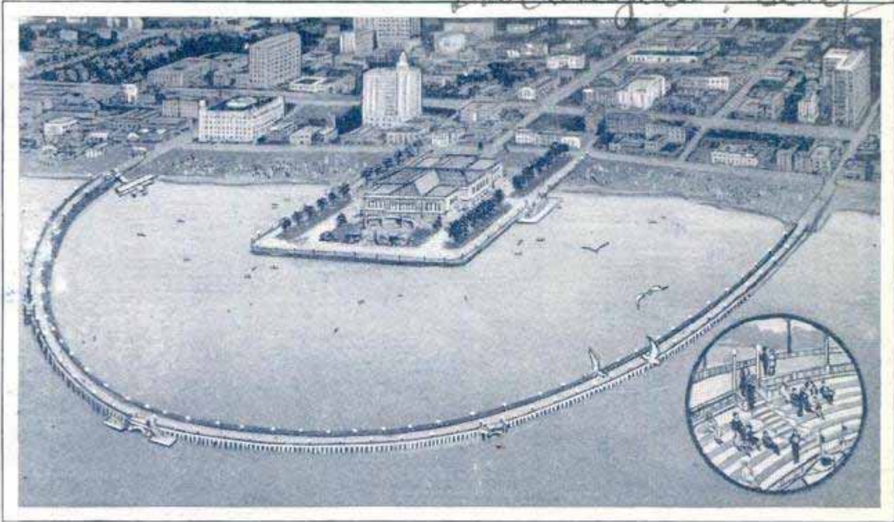
Tide Rips and Undertow, Which Often Prove Dangerous, Are Eliminated at a New California Beach, Which Has a Long Semicircular Sea Wall to Insure Still Water in the Pool
