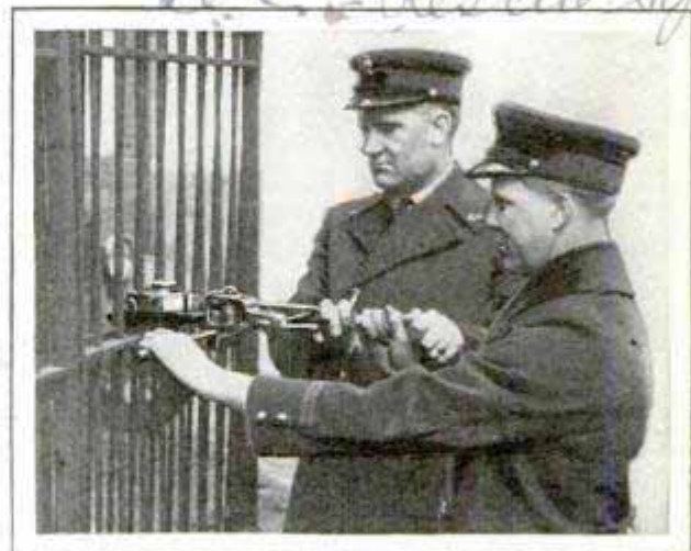
© U. & U. For Speedy Rescue Work; These Powerful Cutters Sever Steel Bars in a Few Seconds
