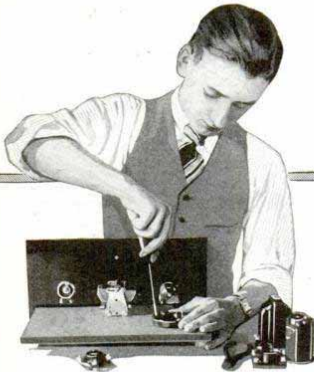
Above, Wood Subpanels Elevated by Wooden Cleats at Each End Allow Wiring to Be Hidden Below and Also Provide Room for Mounting By-Pass Condensers; the Front Panel Is Easily Mounted with Wood Screws without the Aid of Metal Brackets
