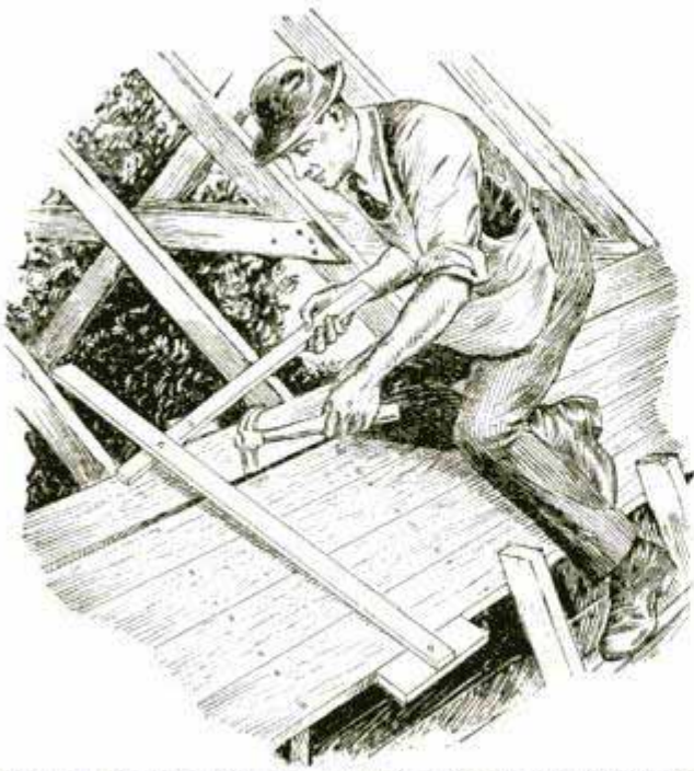
Warped Roofing Boards Can Readily Be Straightened by Means of This Device
