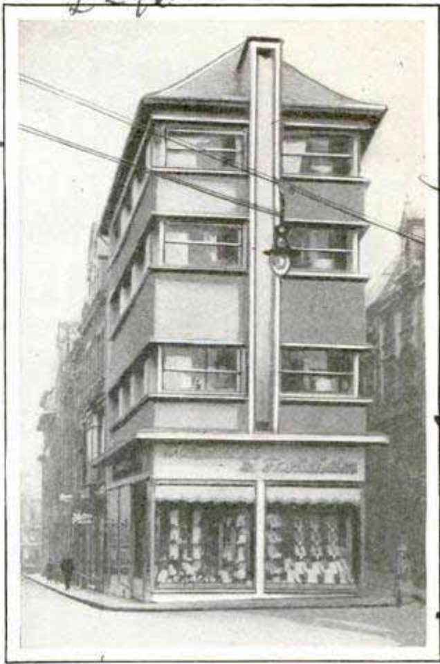
Front View of the All-Steel Building Erected in Essen, Germany; Note the "Groove" for Exterior Lighting
