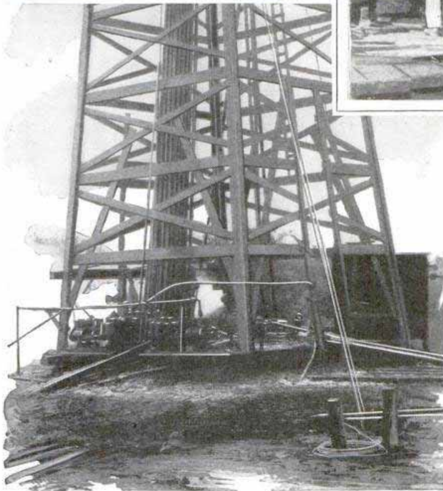
Lowering Sections of Drilling Pipe into a Well, Top, and, Bottom, a Close View of a Rotary Rig, Showing Stacked Pipe and the Mud Pumps
