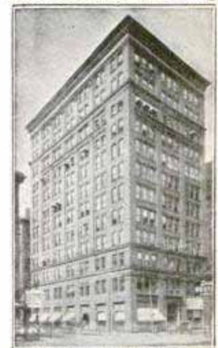
Our Pittsburgh Office Suite 514 Empire Building
