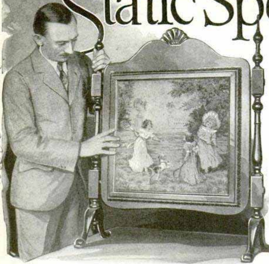
Colin Kyle, with His Electrostatic Speaker, Less Than an Inch Thick, Built into a Fire-Screen
