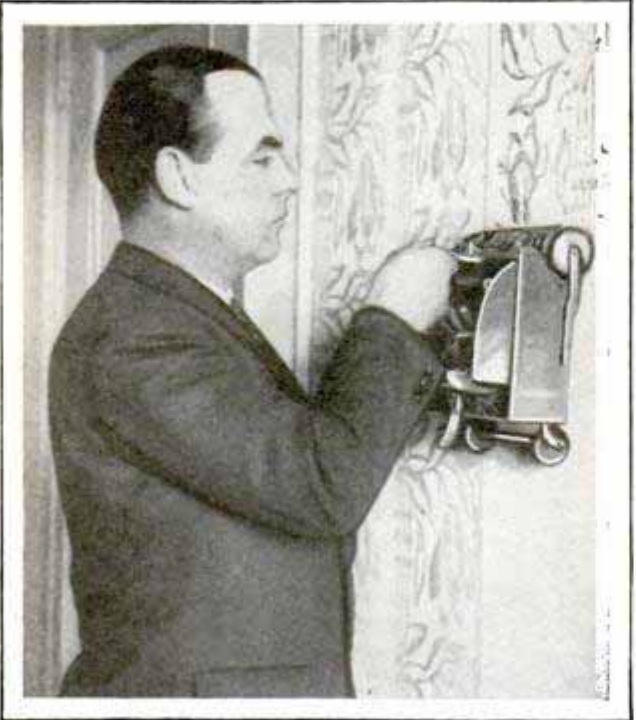
Automatic Decorating Tool, Working Like a Grainer, Which Paints Designs Rapidly on the Walls
