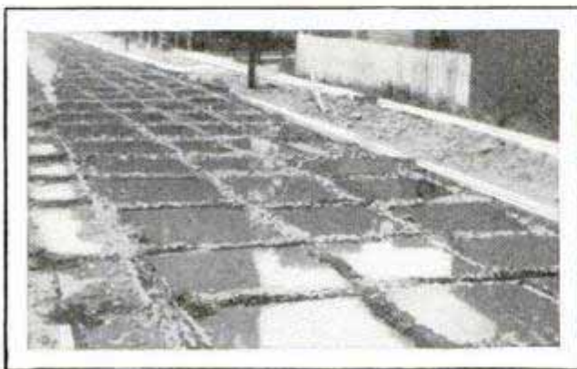
Concrete Pavement Kept from Drying Too Quickly by Small Water-Retaining Dikes
