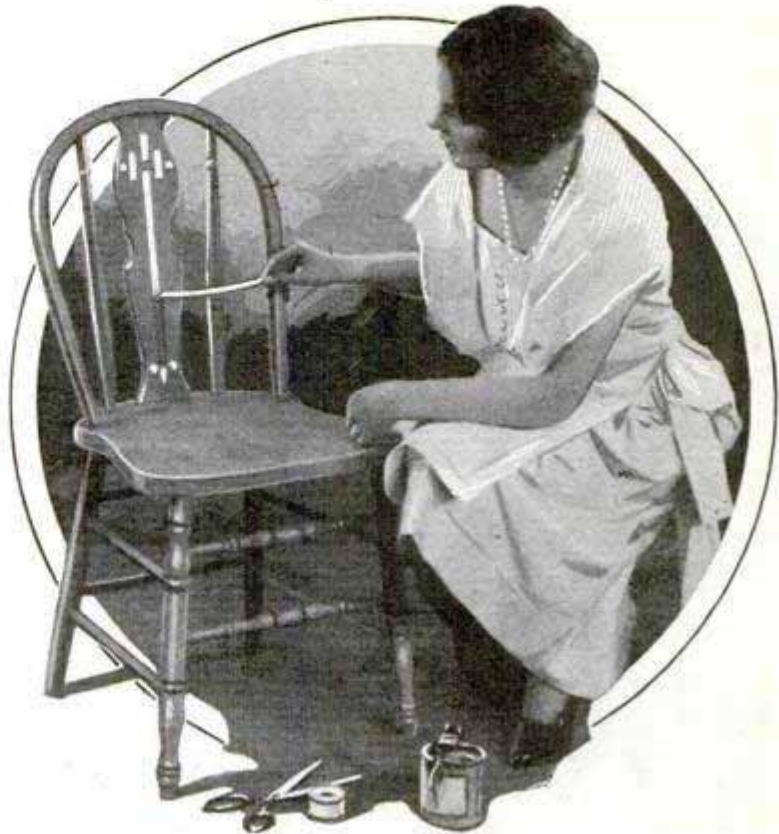
Strips of Ordinary Adhesive Tape Used as Stencil When Painting Furniture
