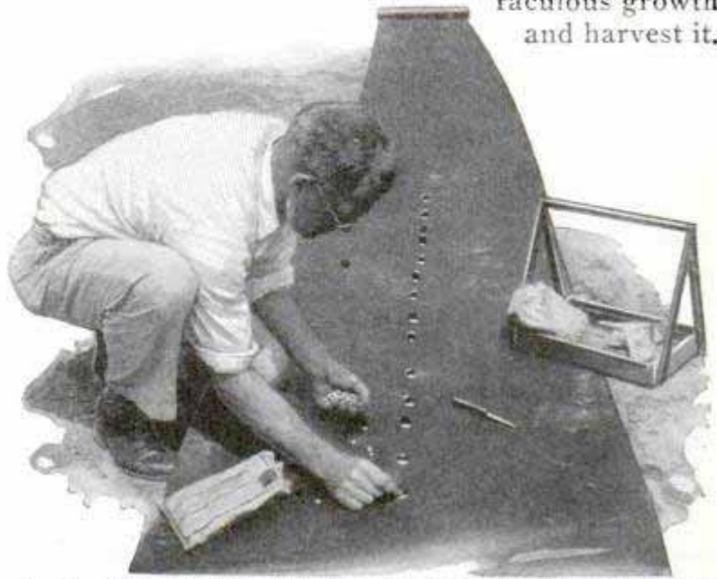
In the Patented Eckart System, the Seeds Are Planted through Holes Cut in the Paper Mulch
