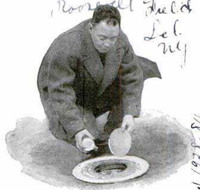
Landing-Field Lights in Small Wells Are Protected against Breakage and Serve as Wind Indicator
