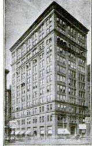
Our Pittsburgh Office Suite 514 Empire Building
