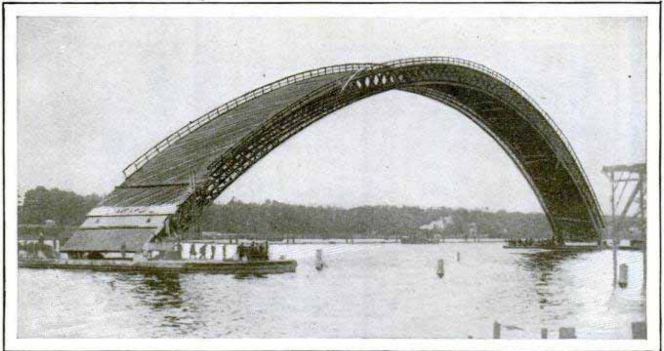
One of the Huge Spans of French Bridge Being Floated into Position; It Is Nearly 600 Feet Long, the Chief Link in the Structure, Which Reaches a Mile across the River Elorn at Brest
