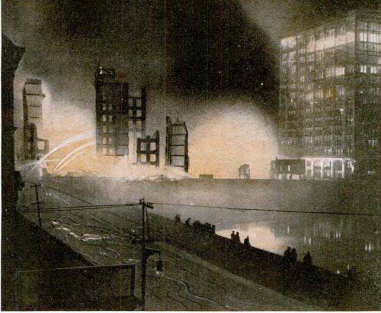
One of the Most Unusual Fires on Record; the Top Floors of the Fireproof Building on the Right Were Set Ablaze by Heated Air from the Conflagration across the Street
