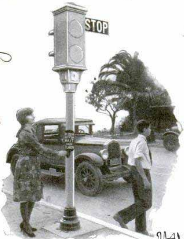
Pressing Button Raises the "Stop" Flag, Which Stays Up for Fifteen Seconds
