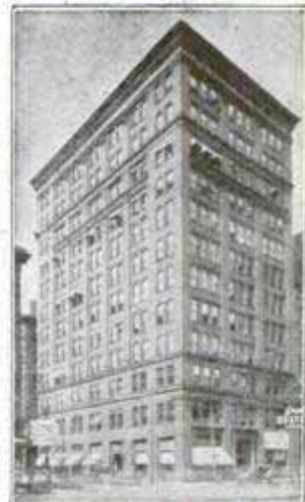
Our Pittsburgh Office Suite 514 Empire Building
