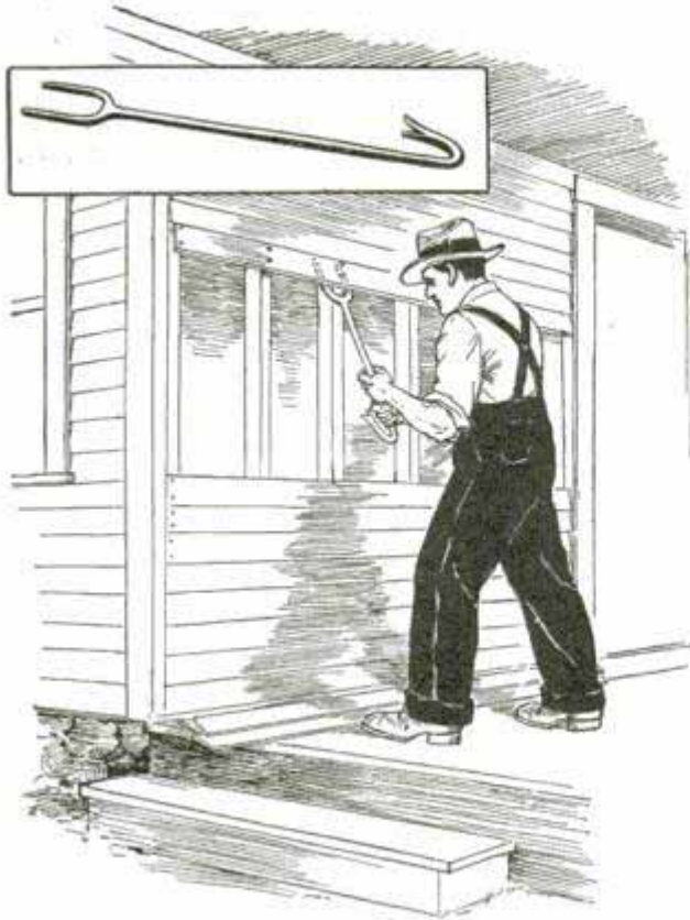
Improvement on an Ordinary Wrecking Bar to Facilitate Removing Siding
