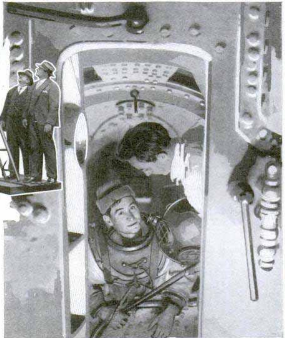
Diver Trying the Sea Door of the "Defender" and Preparing to Leave the Air Lock Which Admits to the Sea
