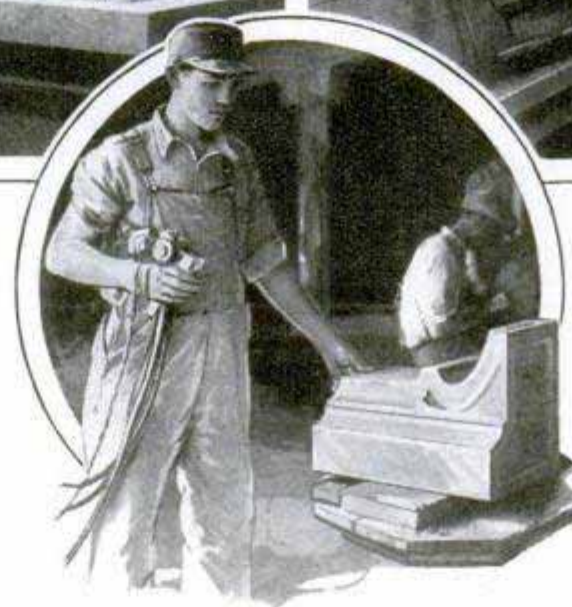
Model of Terra-Cotta Building, Showing the Shaded Effect of Different Colors; Preparing Clay Model for Large Piece, and Spraying Three Colors at Once
