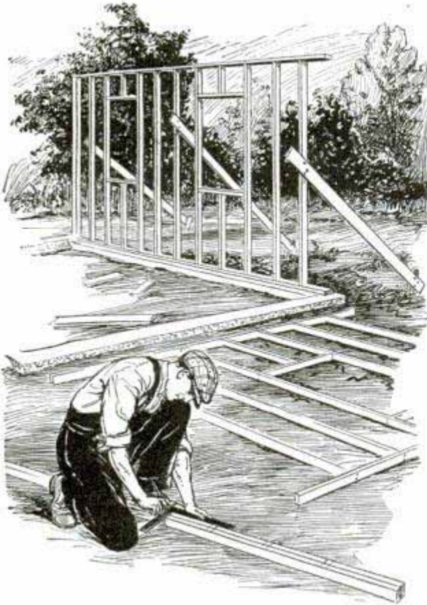
Nailing Studs to Plates on the Ground Saves Time and Much Unnecessary Labor
