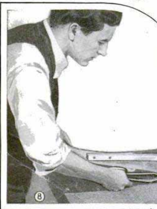
The Rawhide of the Traditional Snowshoe Is Replaced by Galvanized Screening, or So-Called "Hardware Cloth," Cut to Shape with Tin Snips and Tacked in Place
