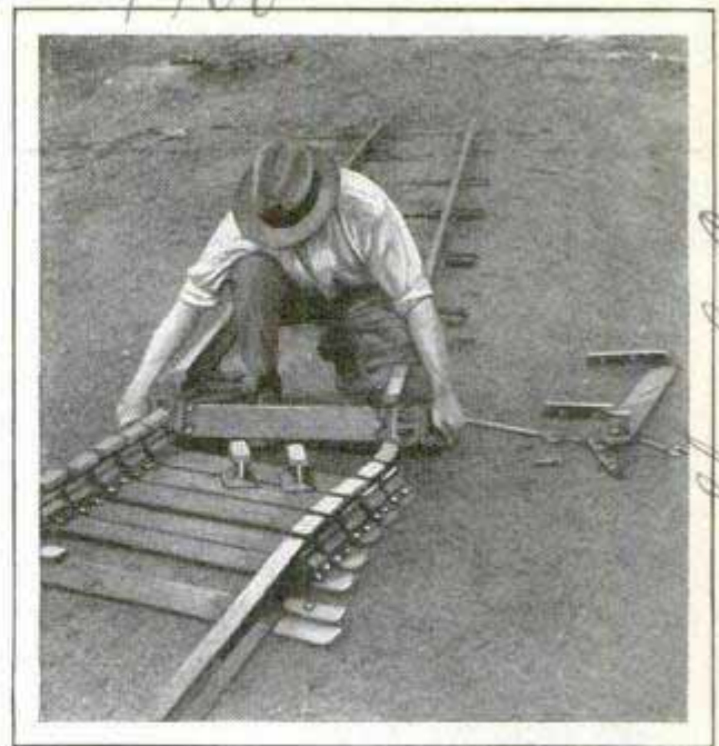
Work Track in Small Sections to Simplify the Removal of Rails or Laying a Curve
