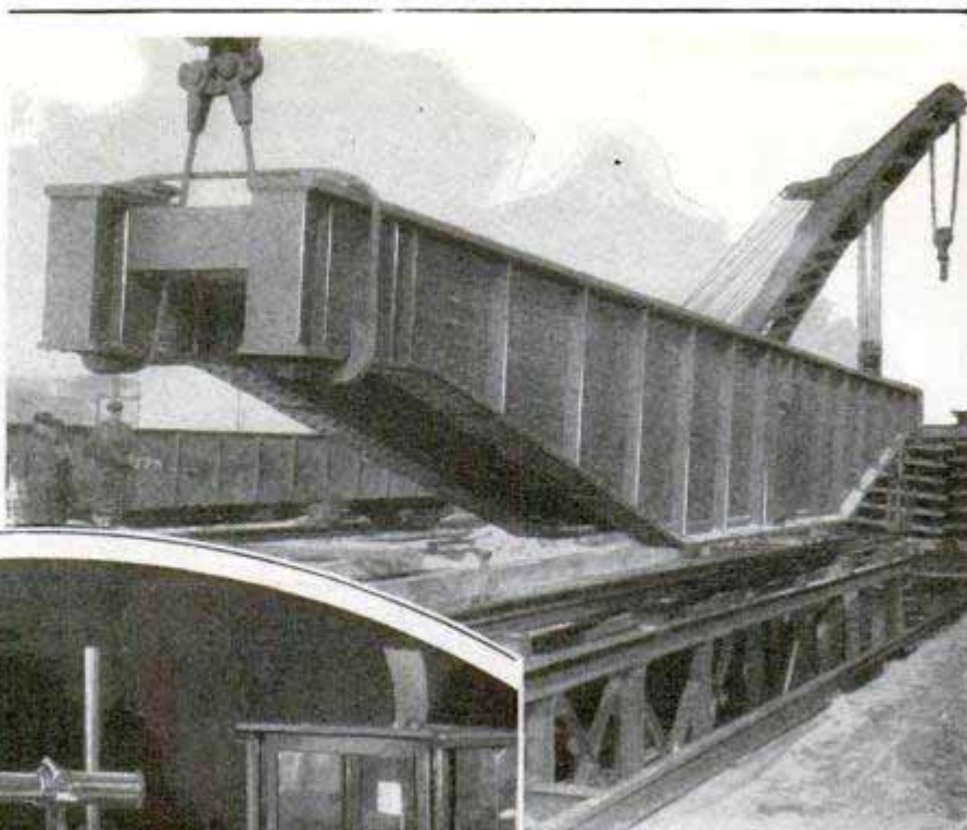
Lowering the Seventy-Five-Foot Fulcrum-Scale Bridge into a Scale Vault on the Pennsylvania Railroad; the Completed Scale Bridge, Including Rails and Ties, Weighs 143,000 Pounds; at Left, Examining at Close Range the Cabinet-Inclosed Precise Test Scale at the U. S. Bureau of Standards; This Machine Will Weigh Objects Down to the Thousandth Part of a Milligram; Some Laboratory Scales Weigh the Millionth of a Milligram
