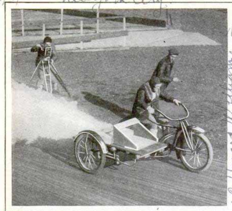
Testing Motorcycle Propelled on the Rocket Principle; Fuel Supply Is Carried in the Sidecar Rack
