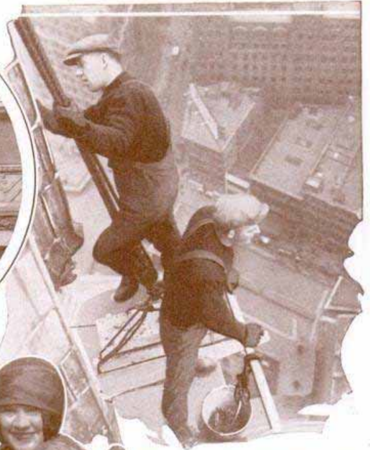
Pointing Up the Cracks in the World's Tallest Building; John Moore and Thomas Thom Were Snapped from a Tower Window of the Woolworth Building at Their Annual Task
