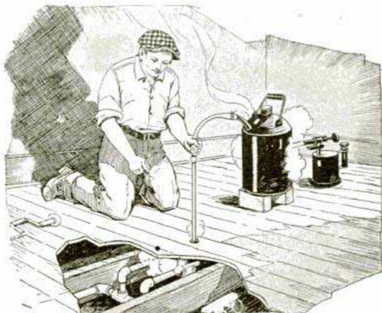
Frozen Water Pipes Thawed Out by Steam Admitted through Small Hole Drilled in Floor
