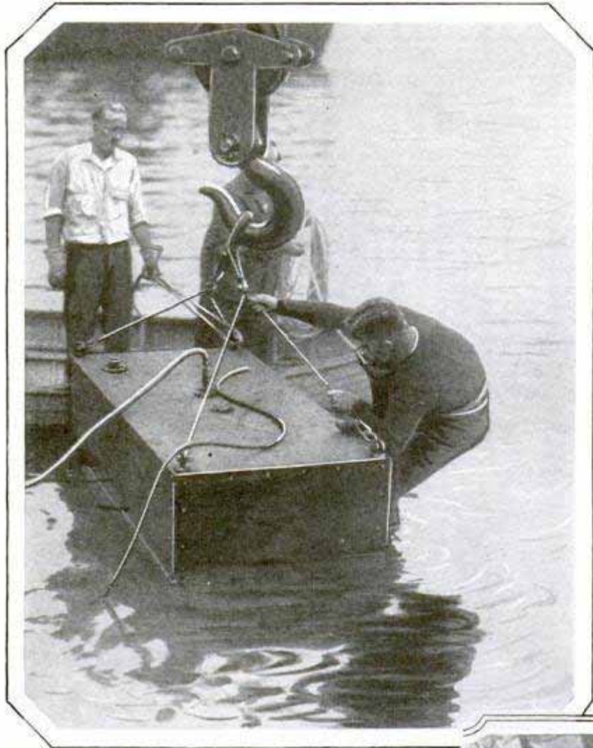
First Stage in Descent with the Diving Bell; Diver Climbing Inside for Lowering
