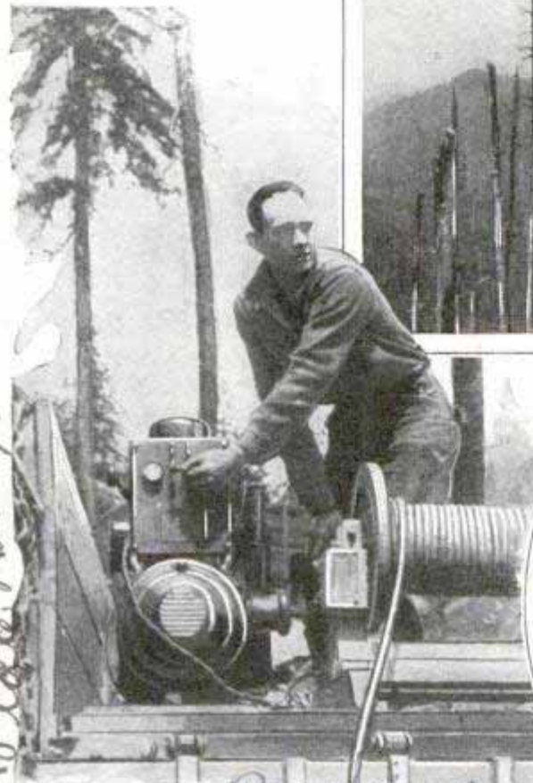
Trees Falling at Blast; Partial View of the Portable Electric Power Plant, Showing Switch being Thrown to Set Off Explosion, and Drilling a Hole for Explosive with a Motor-Driven Auger
