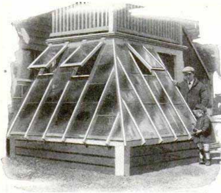
Cambridge School-Teacher Who Glazed In the Space under His Back Porch to Make a Greenhouse
