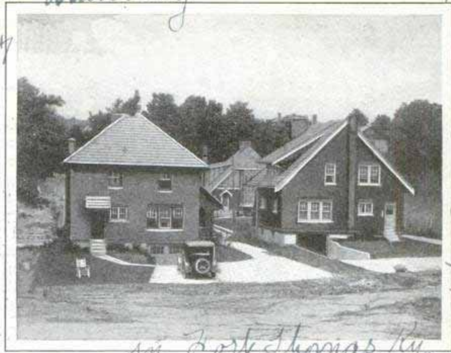
Typical Arrangement for the Basement Garage Which Insures a Warm Place for the Car and Saves Lots of Space
