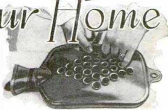
To Hold It in Position, This Hot-Water Bag Has Vacuum Cups That Keep the Bottle on the Body without the Use of Straps or Ties
