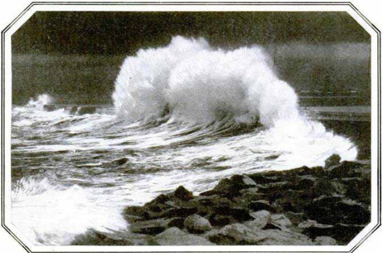
Rearing Dozens of Feet into the Air, Tons of Water Fall Back with a Mighty Crash; the Picture Shows a Huge Wave Striking the Sea Wall at Colombo, Ceylon, in the Far East
