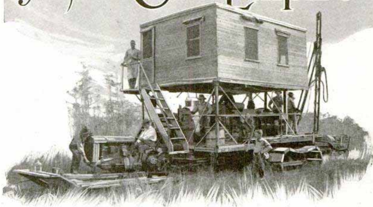
Combination Dynamite Drill, Stump Puller and Traveling Cook Shack. One of the Unique Tools Used to Build the Tamiami Highway through the Wilderness of the Everglades Jungle
