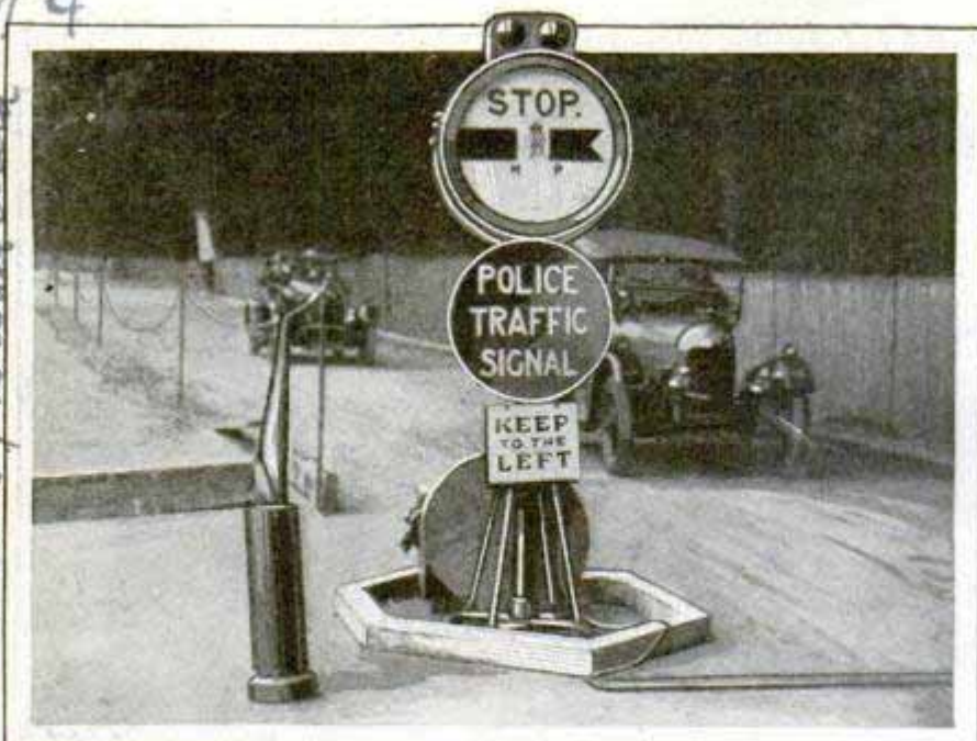
Traffic Light with Alarm Attachment Rung If Car Crosses the Line; the Signal Wire Is Seen at Right
