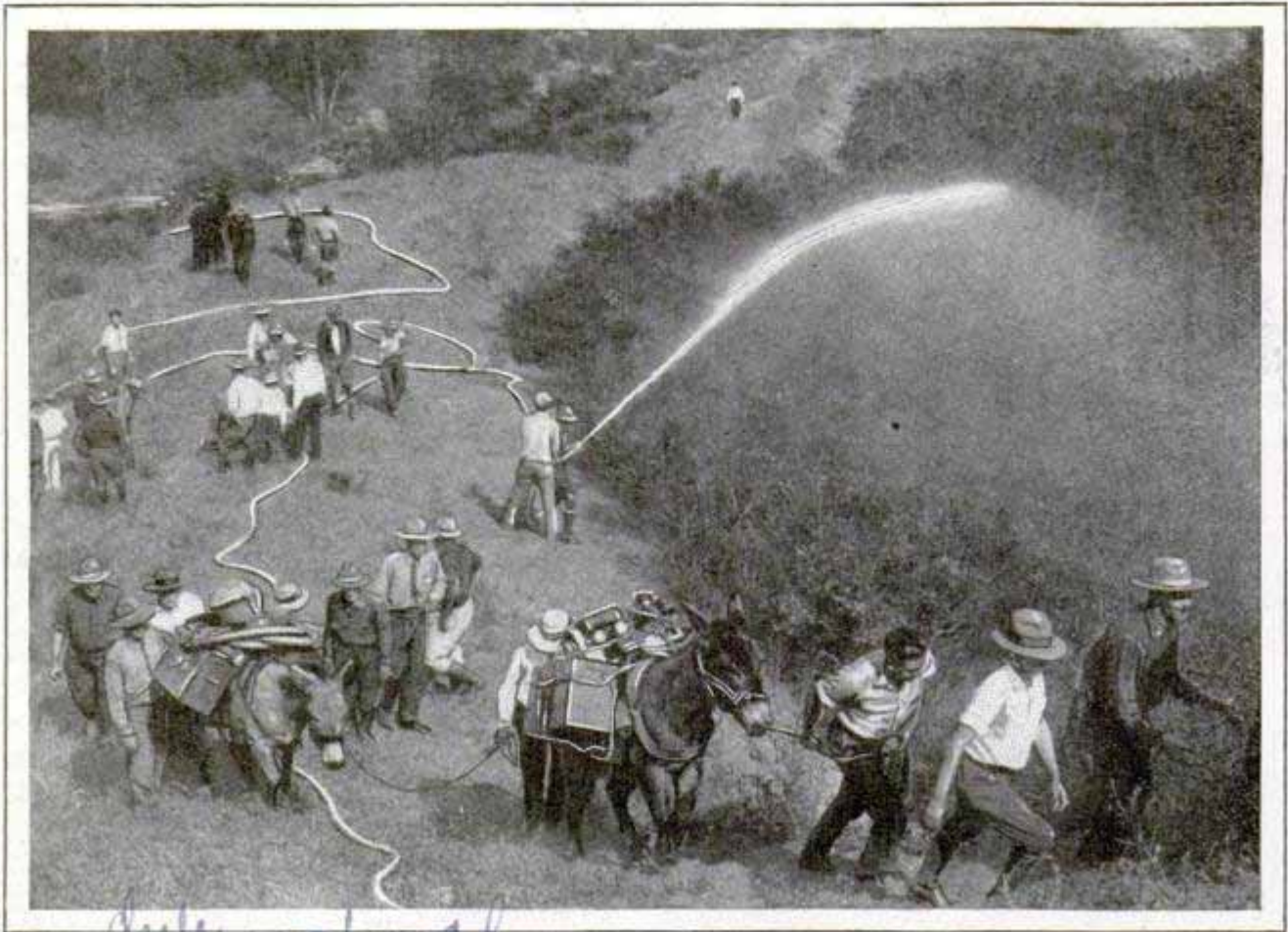
Testing the Portable Fire-Engine Units for Combating Blazes in Western Forests; a Burro Brigade in Action, to Show Efficiency of the Traveling Apparatus
