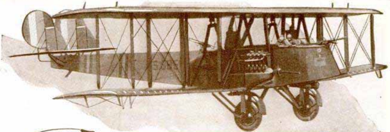
The Army's Latest Twin-Engine Curtiss Bomber; Instead of a Third Engine in the Nose It Carries a Machine Gunner There, While Another, behind the Pilot, Fires toward the Rear, and the Bomber Drops His Missiles through the Floor; Left, a 4,000-Pound Bomb
