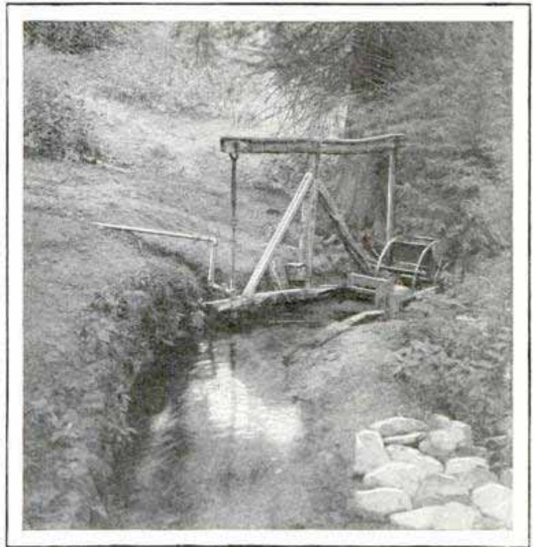
Small Waterwheel Installed in a Brook Operates a Pump Which Raises Water to a Near-By Reservoir
