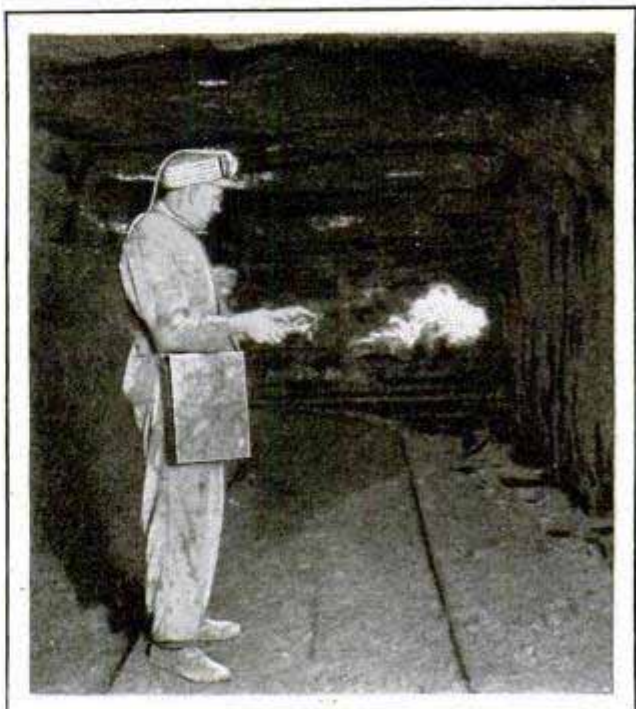
Studying Air Currents in Mine with the Aid of a Smoke Screen That Drifts with the Breeze
