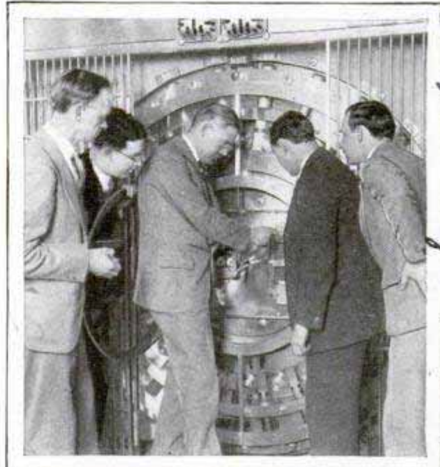
Interior View of Vault, Showing Handle That Unlocks Door from Inside
