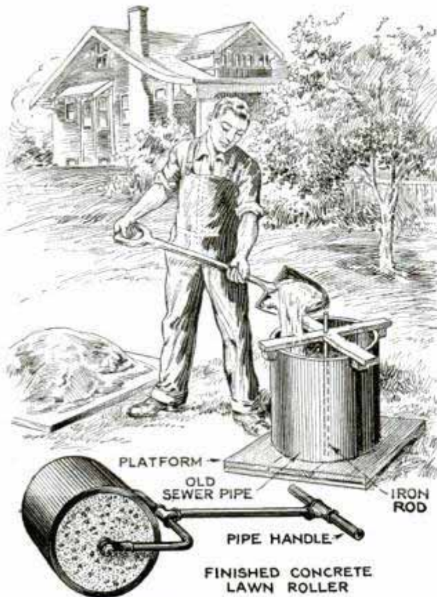
A Lawn Roller Made from a Sewer Tile Filled with Concrete and a Mounting of Pipe
