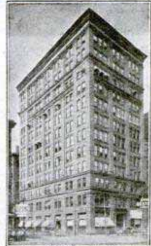
Our Pittsburgh Office Suite 514 Empire Building
