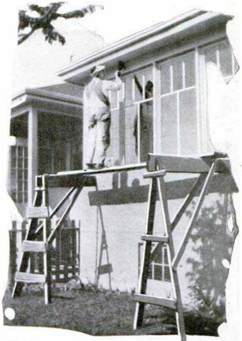
Simple Lean-To Scaffold Is Easy to Erect and Takes Little Space in the Workman's Truck
