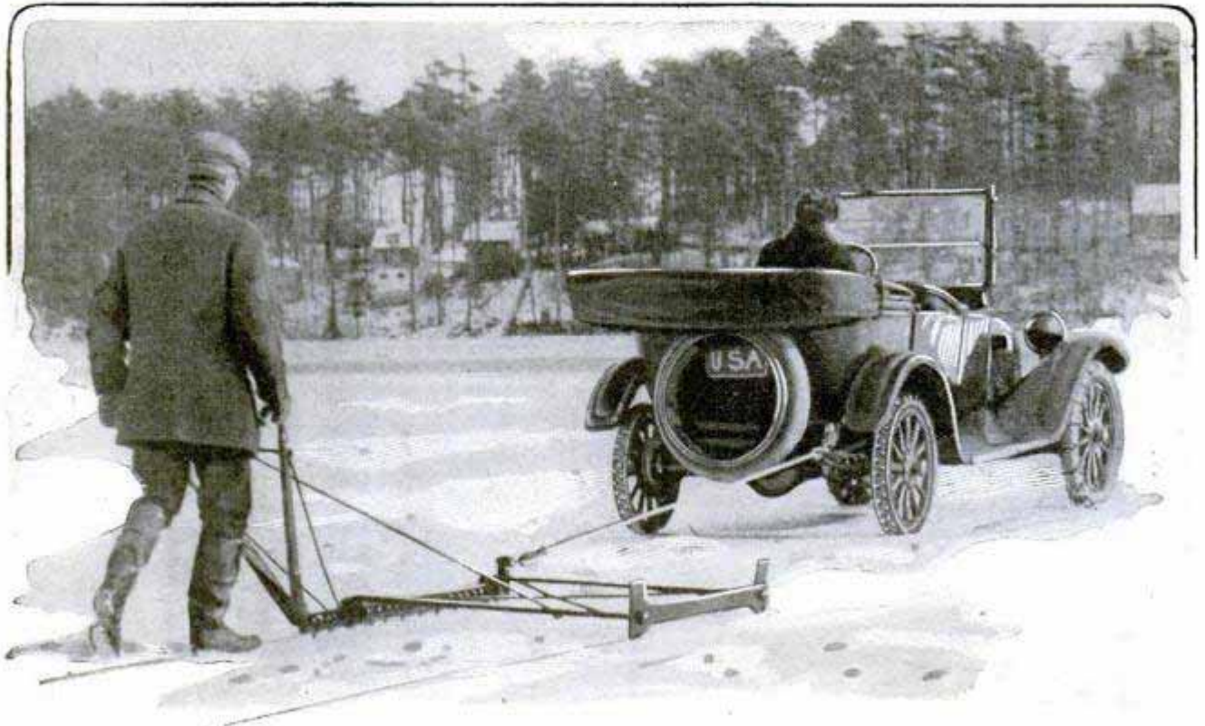
Old Auto Equipped with Spiked Rear Wheels and Provided with Skid Chains on the Front Wheels, Facilitates the Work of Cutting and Hauling Ice
