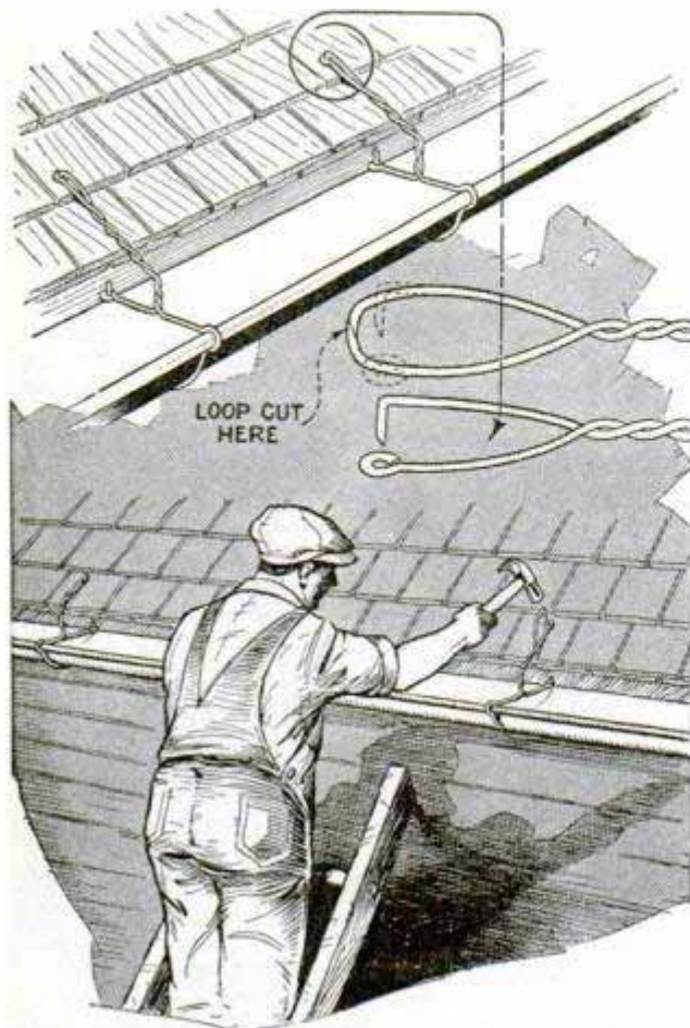
Improved Hangers Hold Eave Troughs in Position While Attaching Regular Hangers
