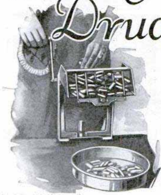
String Beans Are Cut in Uniform Lengths by This Outfit, Especially Adapted for Canning Large Quantities
