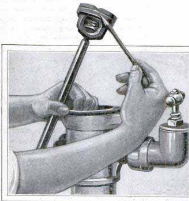
Above, the Plunger Spider; Upper Right, Form of Deck Leather and Weight; Center, Removing the Cylinder
