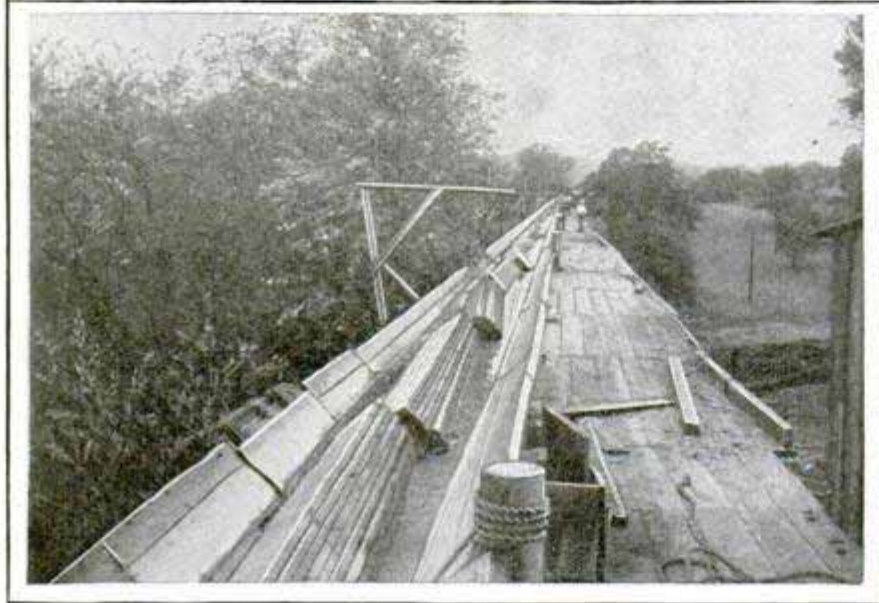
Two Views of a Sixty-Mile Flume, Built at a Cost of $3,000 a Mile, to Carry Lumber from a California Sawmill to the Railroad
