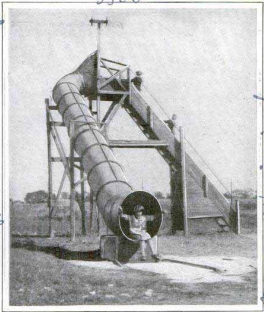
The Fire-Escape Slide for Outdoor Playground Gives a Much Longer and Faster Coast
