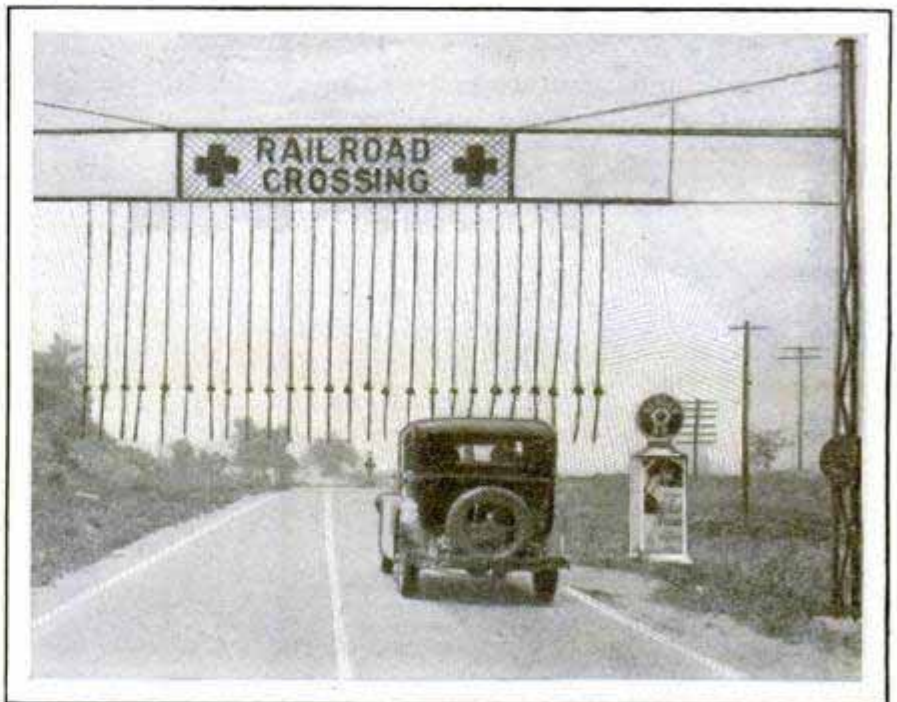
To Rouse the Indifferent Motorist to the Danger of the Railroad Crossing Ahead; the Straps Are Always on Duty
