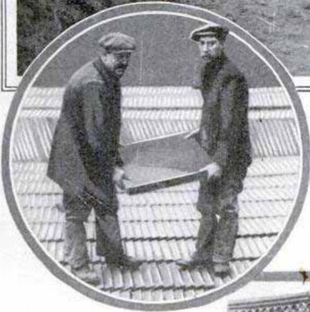
Old Tin Cans, Melted and Run into Molds, Make Paving Blocks
