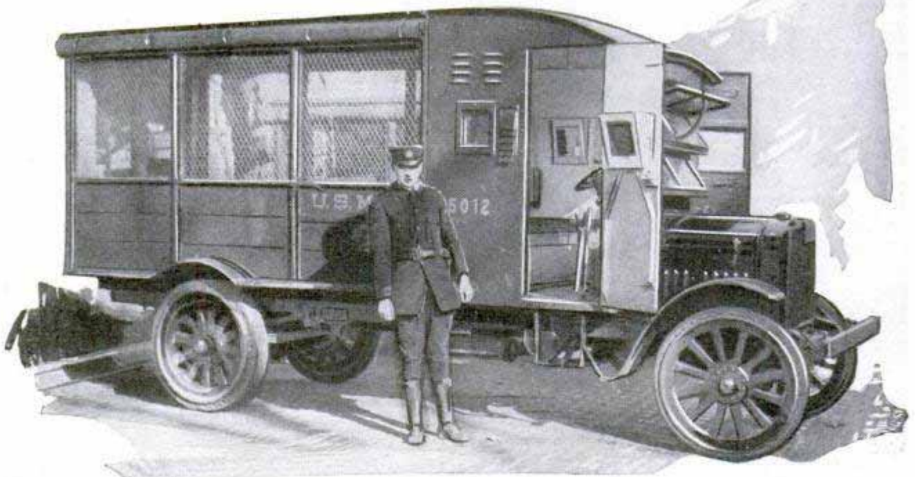
New Type of Mail Truck; the Armed Driver Rides in a Bullet-Proof Cab, Ready to Meet Bandit Guns with a Shower of Lead, While Steel and Bullet-Proof Glass Guard Him
