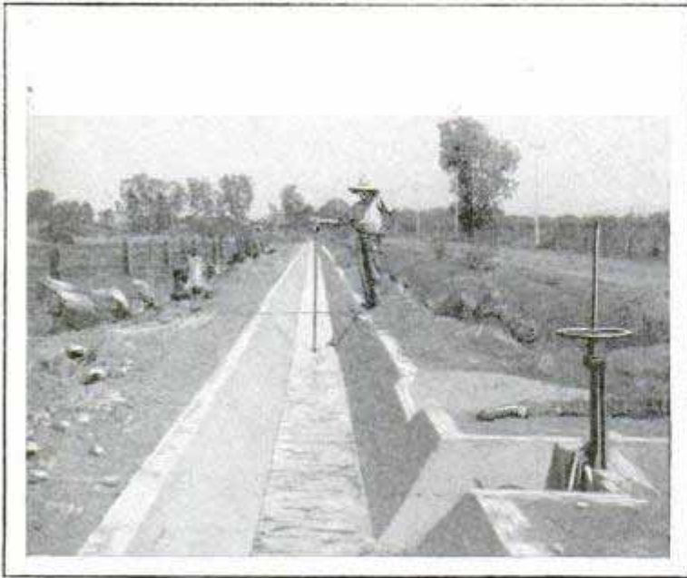
Drainage-Canal Banks Built at an Angle of 45 Degrees Are Most Economical
