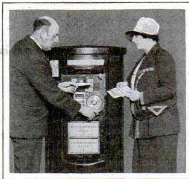
Slot Machine That Cancels Letters, Saving the Use of Stamps; It also Serves as Mail Box
