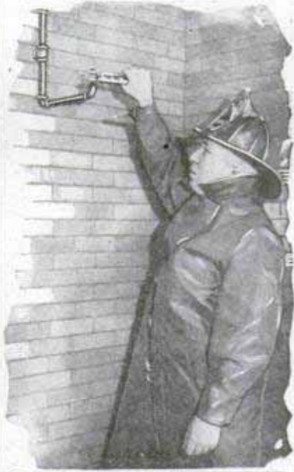
Shutting Off Sprinkler at the Head, to Prevent Further Damage from Water
