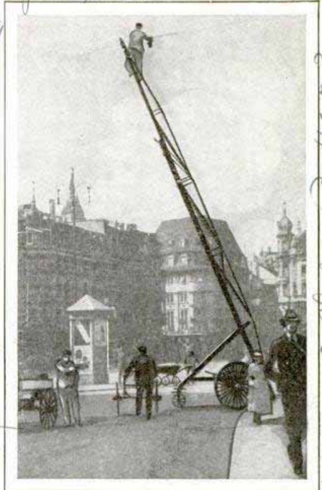
Ladder for Washing Overhead Street Lamps Does Not Obstruct Traffic, and Saves Time
