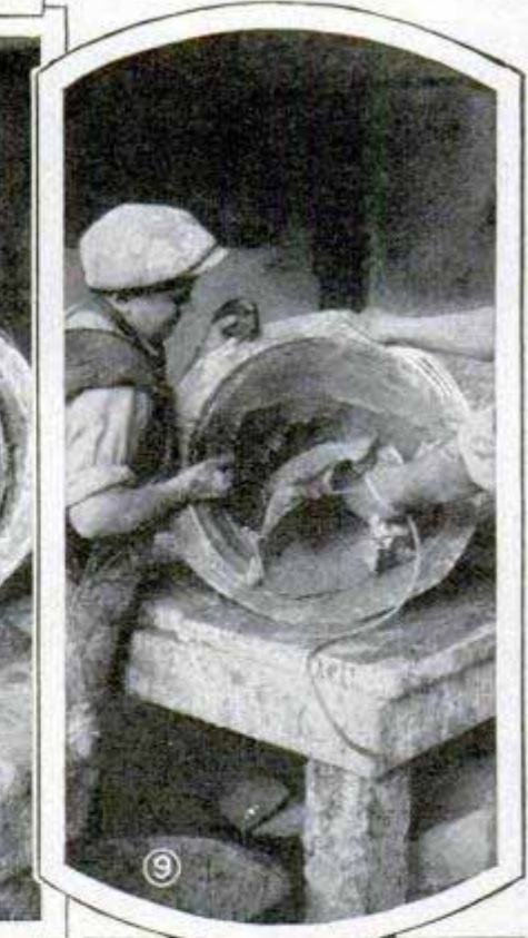
Pulling the Rope to Withdraw the Sack; the Clay Clinging to the Wall Is Then Washed Out with a Hose
