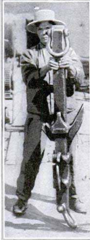
Huge Grappling Iron, Above, Which Has Been Broken by Contact with Rocks on the Sea Bottom, While Trying to Find the Cable; at Left, Workmen Repairing the Armored Sheath, the Last Step in Making a Splice in the Cable before Returning It to the Ocean, Ready Again to Transmit Messages
