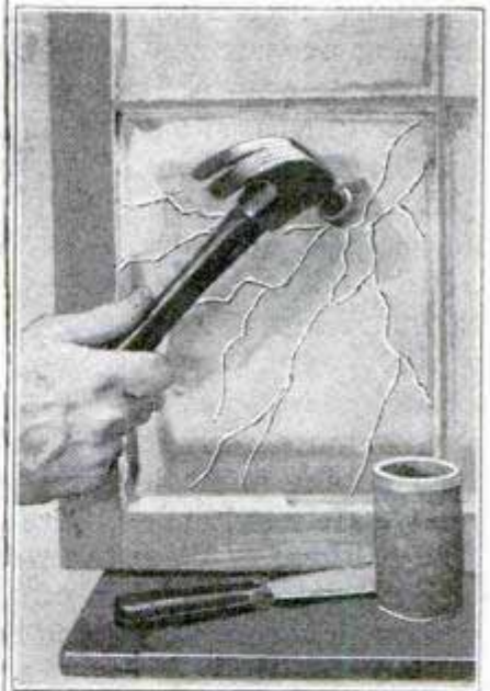
How a Cracked Pane Can Be Shattered without Dropping Any of the Glass in Removing It
