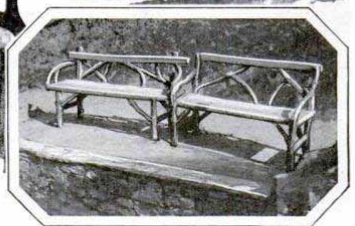
Showing How Bark Is Imitated in Concrete; Note Cement Nail in Third Plank at Left; Right, Rustic Seats of Cement
