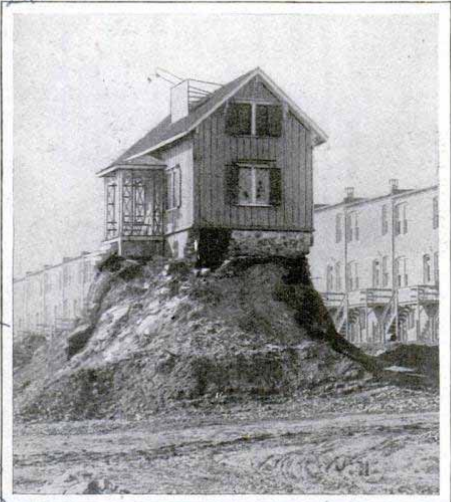
Perched on Its Narrow Pinnacle of Earth, After Street Graders Had Excavated Material around It; the Stranded House before Wrecking
