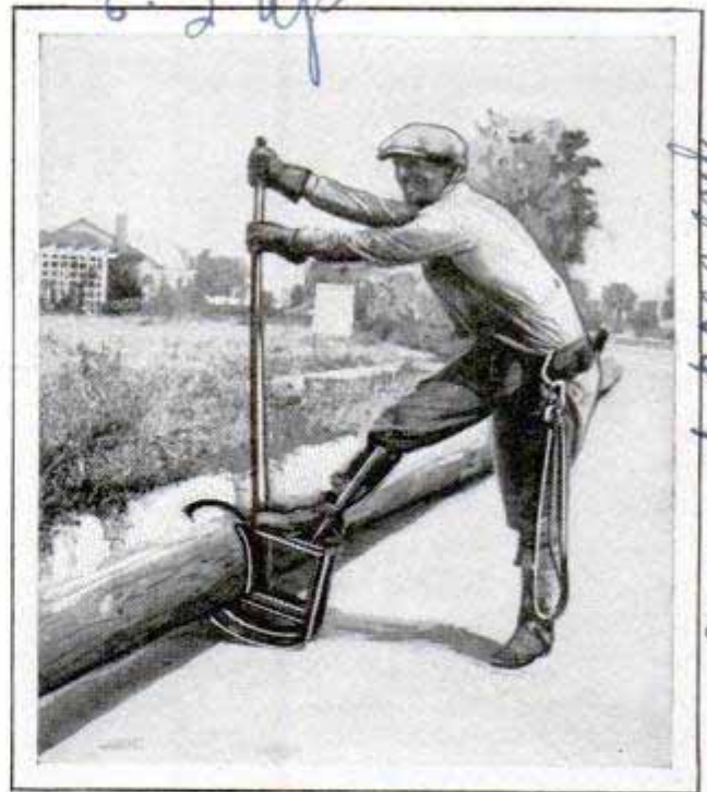
Pulling Telephone Pole onto Its "Cradle": One Man Can Safely Do This with a Cant Hook
