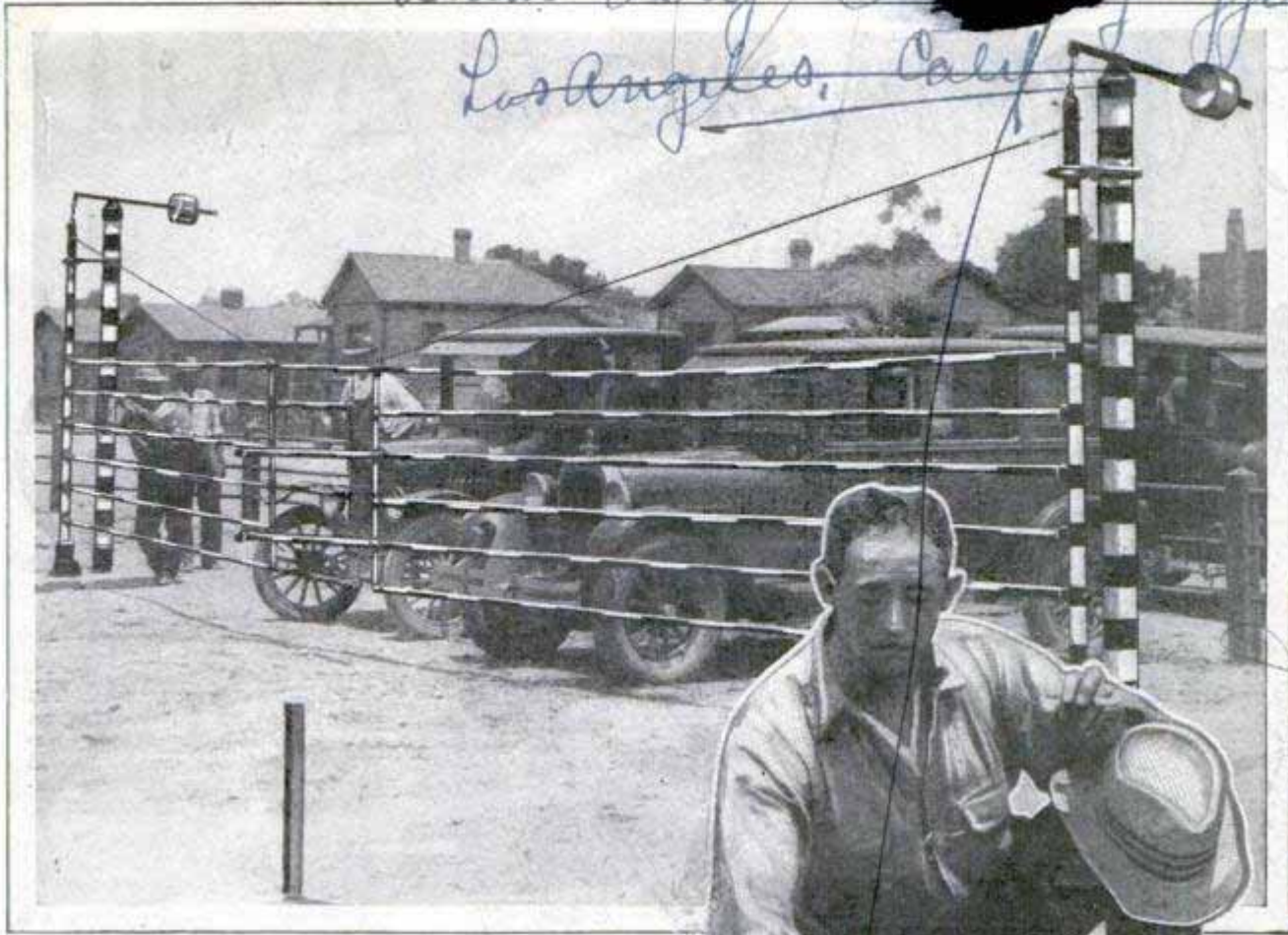
Gates Shut and a Close View of the Electric Unit through Which Train Makes Contact
