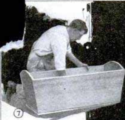
Fig. 7. Marking off Bottom; Fig. 8, Fitting Lining in Ends.
