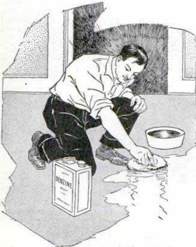
Left, Cleaning Off Dirt, Wax and Grease from an Old Floor with Benzine; Right, Applying the Ground Color on the Cleaned Floor
