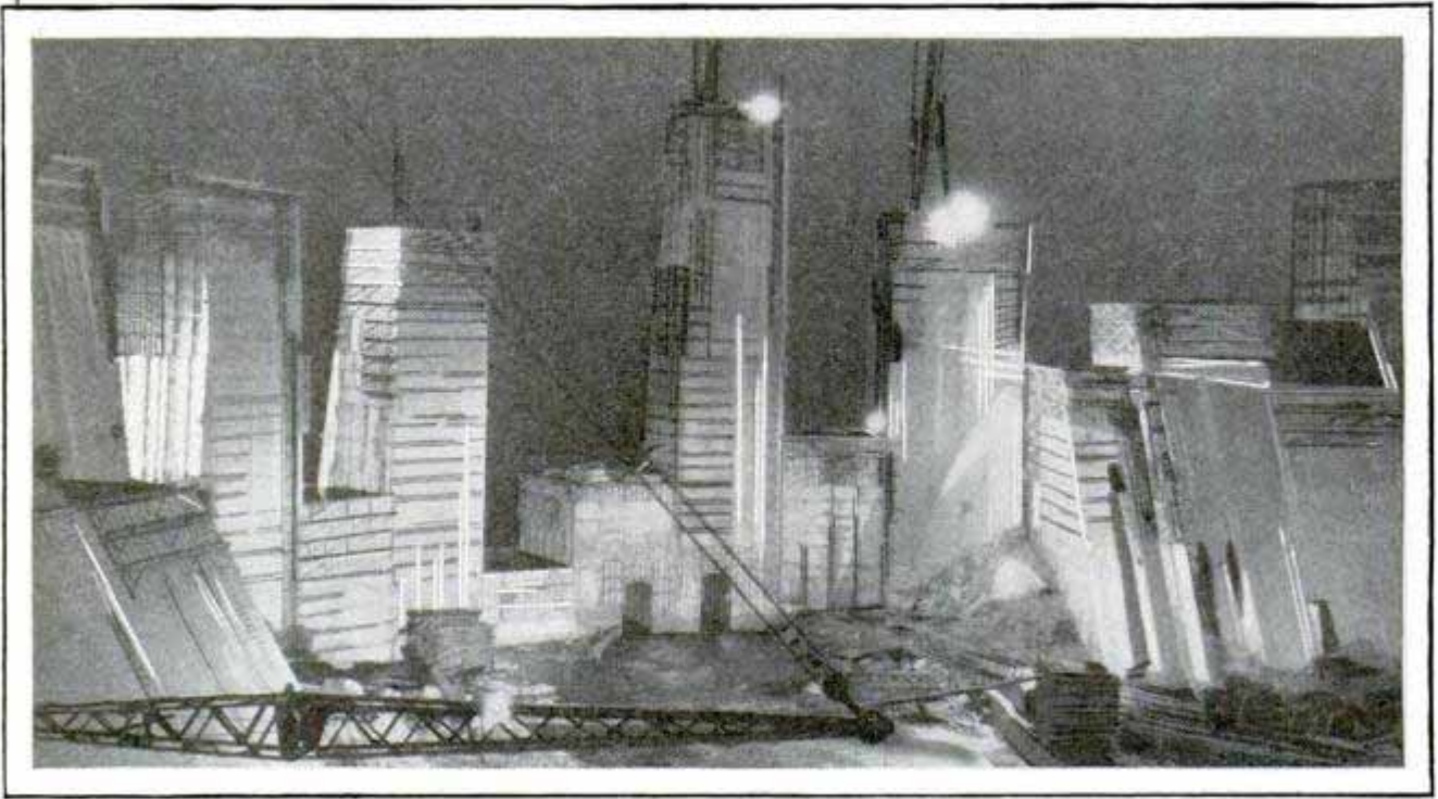
Like Some Weird Metropolis of the Future, the Towering Concrete Forms of This Huge Dam Stand Out under the Floodlights Which Illuminate the Work at Night
