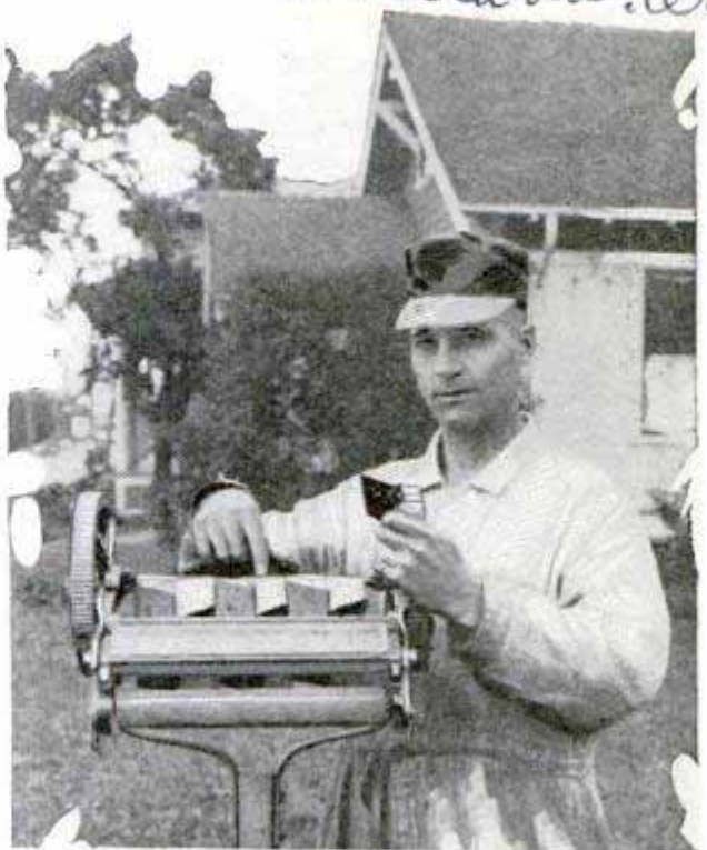
Lawnmower with Interchangeable Blades, Based on the Safety-Razor Principle
