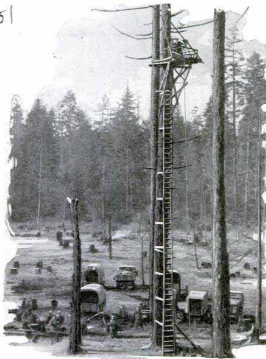
Lofty "Tripod" for Motion-Picture Camera in Filming Outdoor Scenes; the Ladder and Platform Built on Tall Fir Tree
