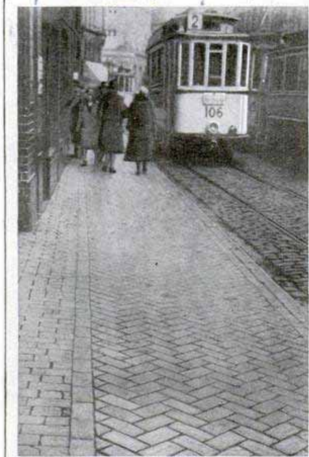
Sidewalk in Berlin Made of Bricks Formed of the Slag Left When Refuse Is Burned
