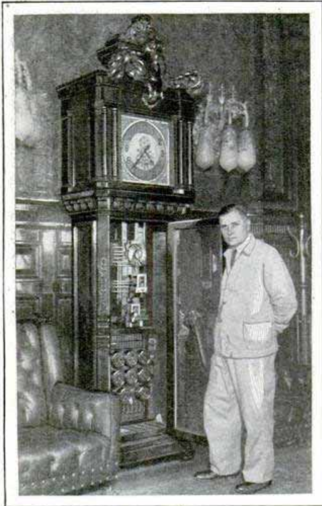
Where the Time Is Controlled for a Big City Building, the Master Clock in the Metropolitan Life Offices
