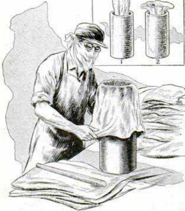
Quick Method of Turning Empty Cement Sacks Inside Out over a Section of Eight-Inch Tile
