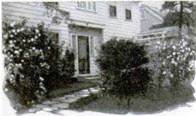
Entrance Walk Laid with "Natural" Concrete Flags, Closely Simulating the Real Thing
