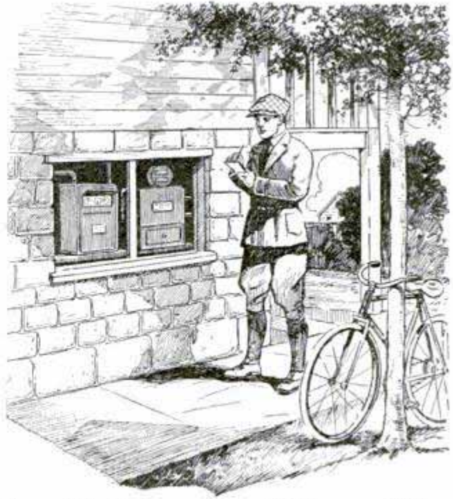
Gas and Electric Meters Arranged in Basement Window
