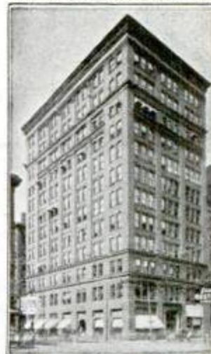
Our Pittsburgh Office Suite 514 Empire Building
