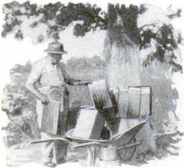
Quick and Handy Method of Painting or Staining Shingles without Waste
