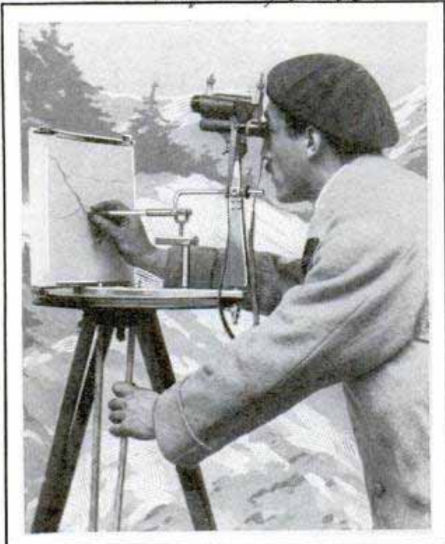
Guiding the Hand through the Binoculars; Profiles Are Easily Copied with Braced Pencil
