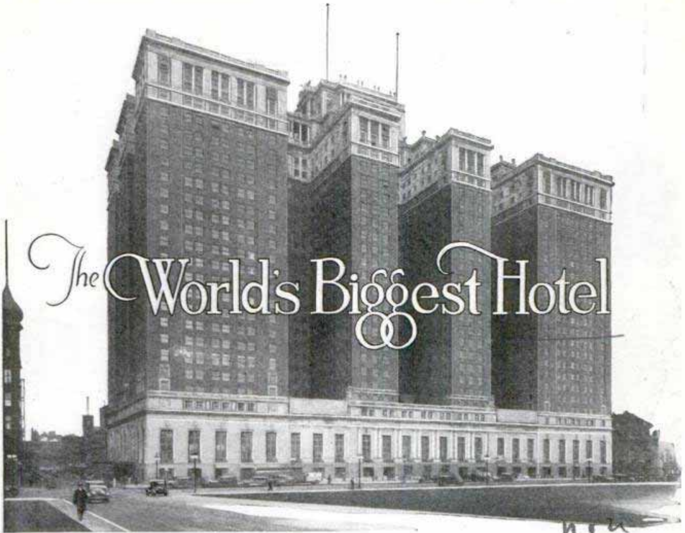
The Stevens Shortly before the Opening; the Structure Is Twenty-Five Stories above Ground and Four Below, Cost, with the Land, $27,000,000, and Contains 3,000 Rooms
