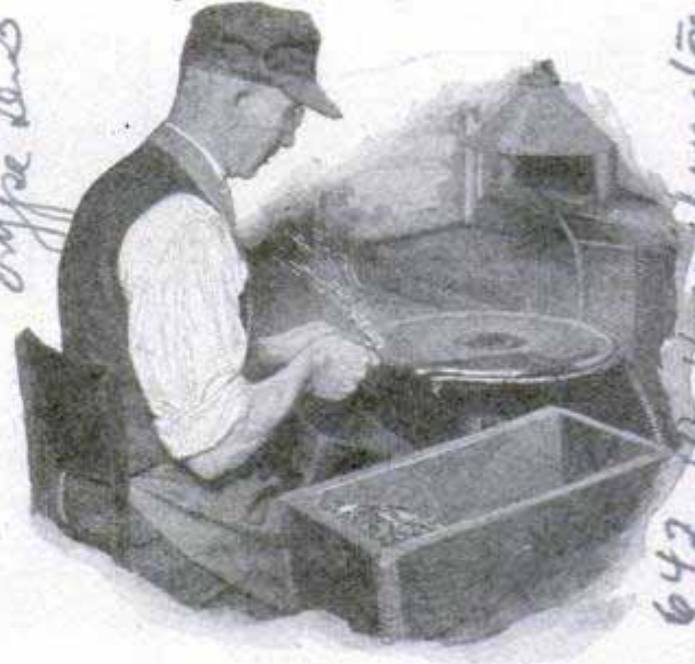
Horizontal Disk Grinder in Operation; Sparks and Dust Fly Away from Worker's Face
