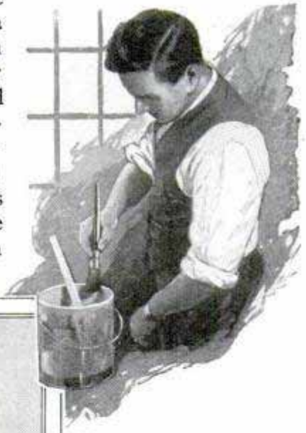
For Window Trim, Use a Flat or Oval Sash Brush
