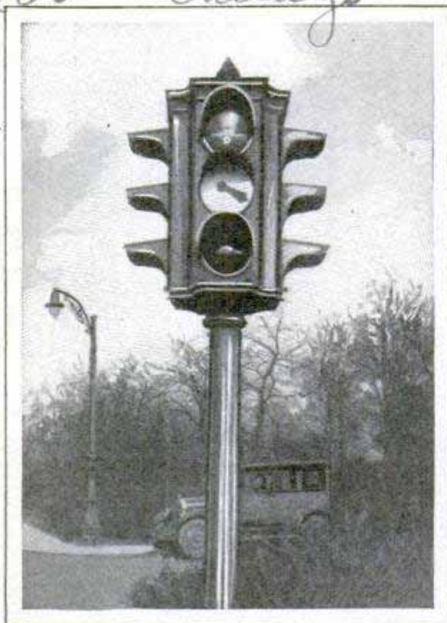
To Help the Pedestrian in Crossing the Street; the Moving Arrow in Center Indicates Walking Time
