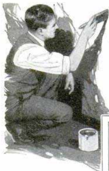
For Painting Walls, Use a Wide Brush and Save Time
