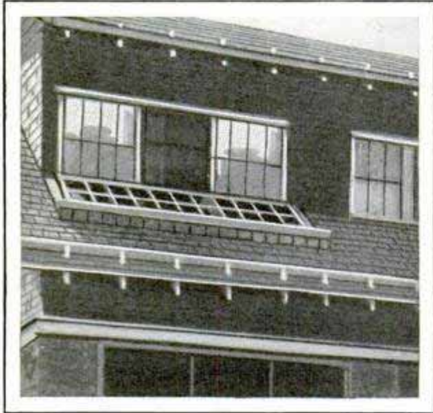
Hotbed on Porch Roof Is Convenient and Out of the Youngsters' Reach
