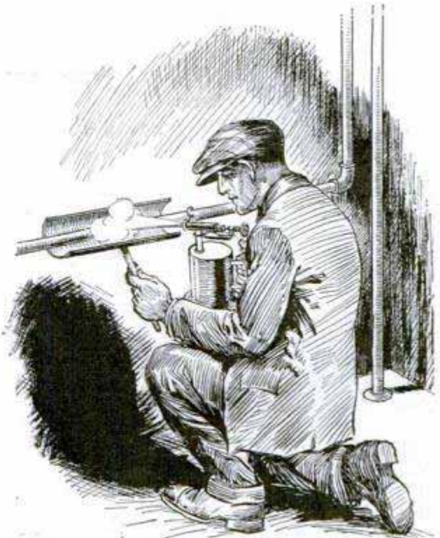
Semicircular Shield Keeps Heat around Frozen Pipe and Hastens Thawing
