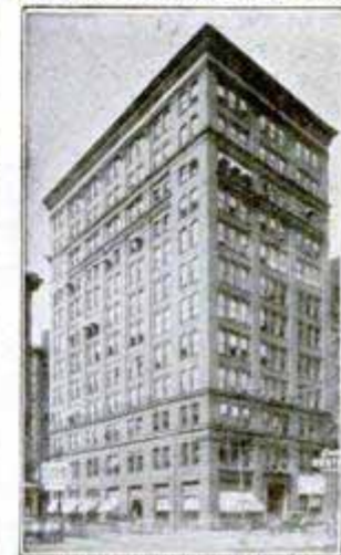
Our Pittsburgh Office Suite 514 Empire Building
