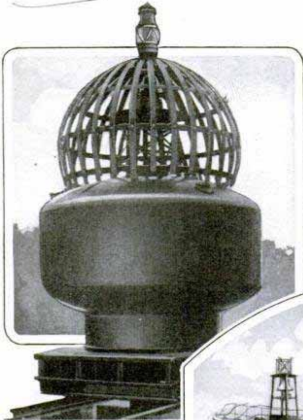
Automatic Gas Buoy, Showing the Underwater Tank That Holds the Fuel, and, at Right, Type of Lightship Employed off English Coasts
