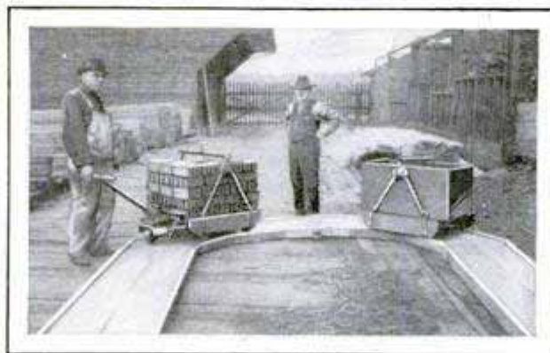
Loaded Brick Carriers Are Hauled to Building Directly from Yards, Saving Piles in Street
