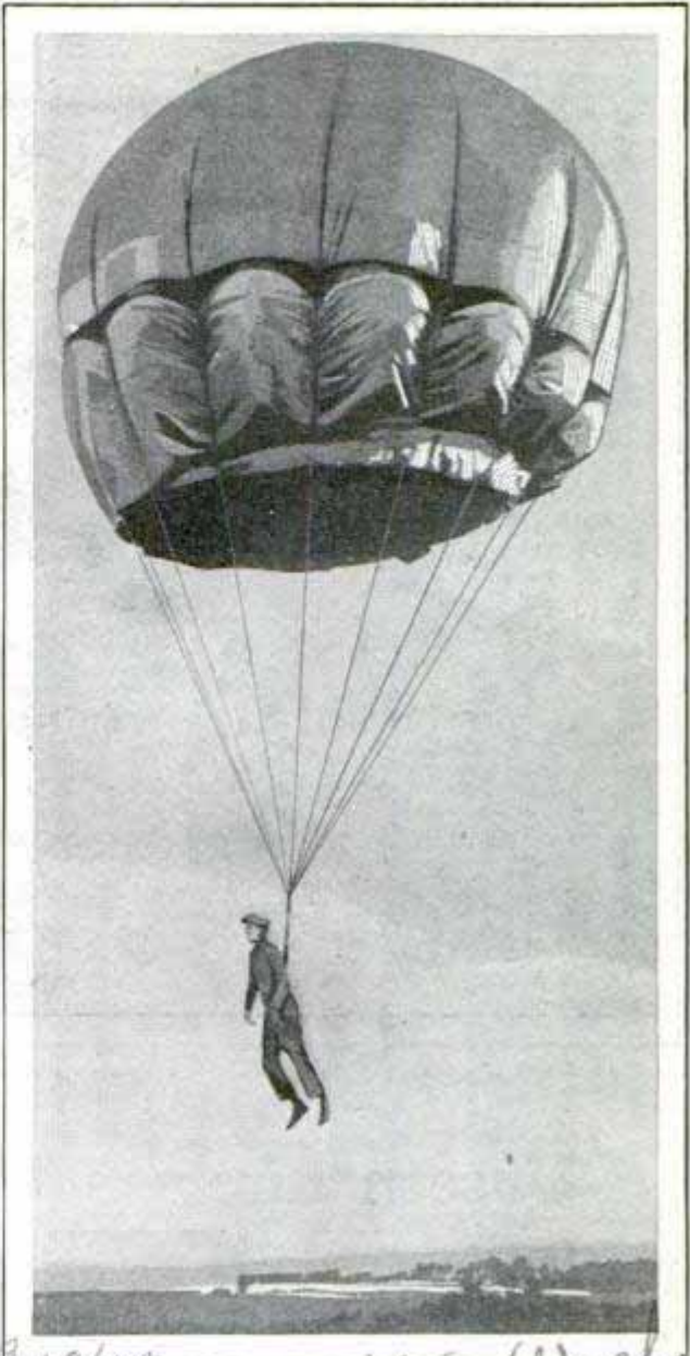
Testing the Parachute with Dummy; the Pockets on Sides Serve as Supplementary Supports
