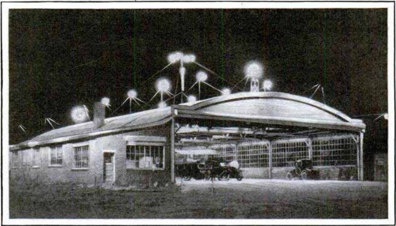
Hangars Are Covered with Lights to Warn the Pilots to Steer Clear in Making a Night Landing; the Dispatcher's Office Is in the Corner, and Back of It, the Pilots' Clubroom
