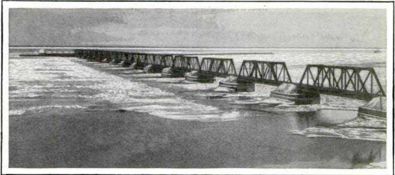
Bridge and Artificial Island Built in Hudson Bay, at Port Nelson, to Furnish Protection for the Harbor; Steel and Concrete Piers Resist the Ice and Break Up Jams
