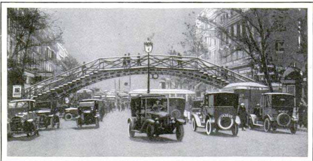
Bridge for Pedestrians over Busy Automobile Street Is Expected to Reduce Traffic Delays as Well as Help Save Lives; Absence of a Supporting Column Leaves Way Unobstructed
