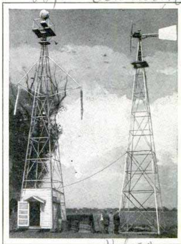
Propeller Windmill and Air-Mail Light, Which Is Supplied with Current from the Mill
