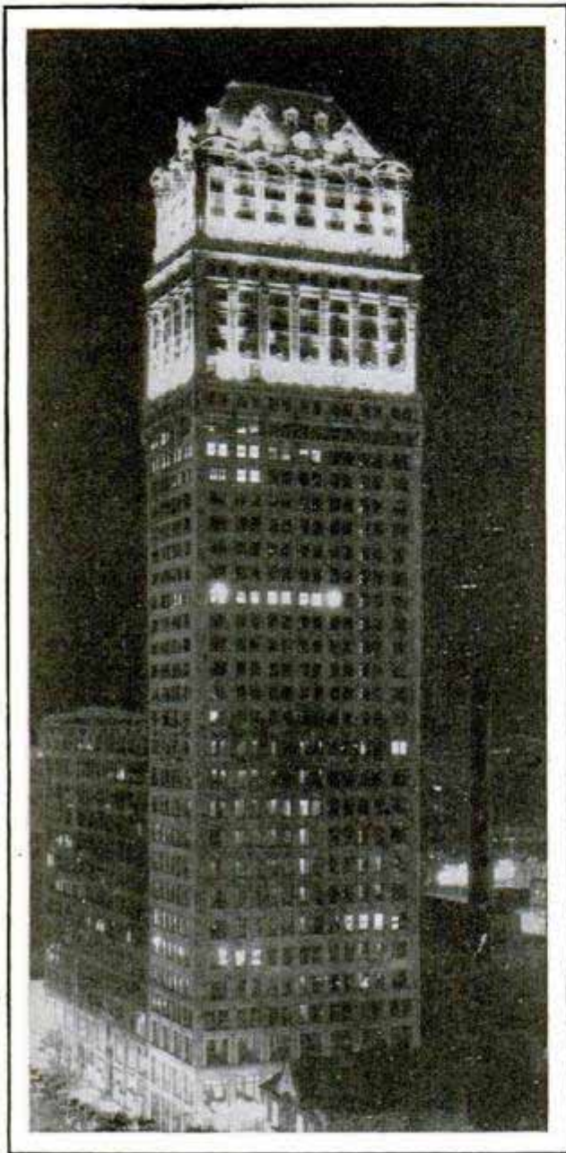
Courtesy General Electric Co.
