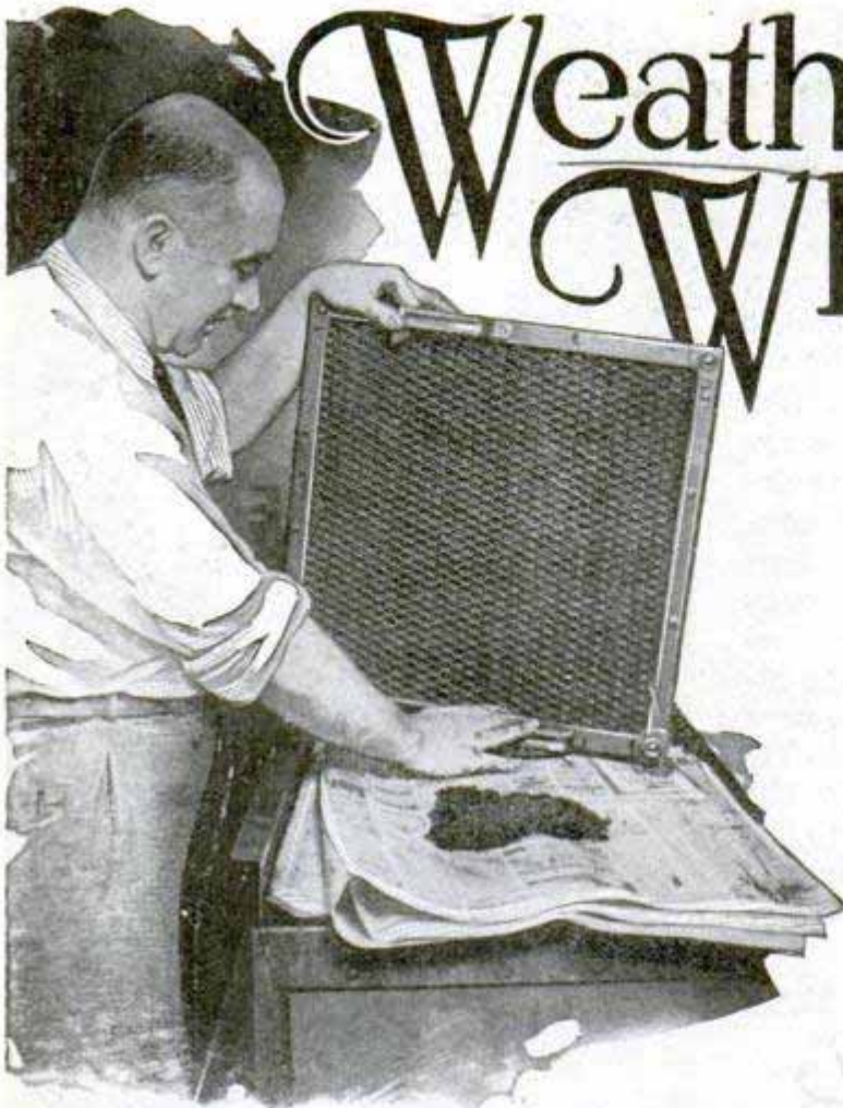
Shaking Dust and Soot from an Air Filter; Hundreds of Pounds Are Collected Yearly from a Single Large Building
