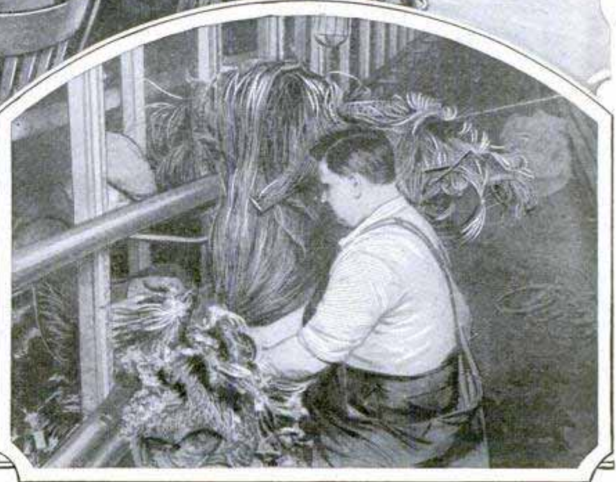
Above, a Long-Distance Test Panel in a Big Exchange, Where Experts Check the Condition of All Circuits, and, in Case of a Break, Determine Its Location; at Right, a Lineman Is Splicing 2,200 Pairs of Phone Wires in One Cable
