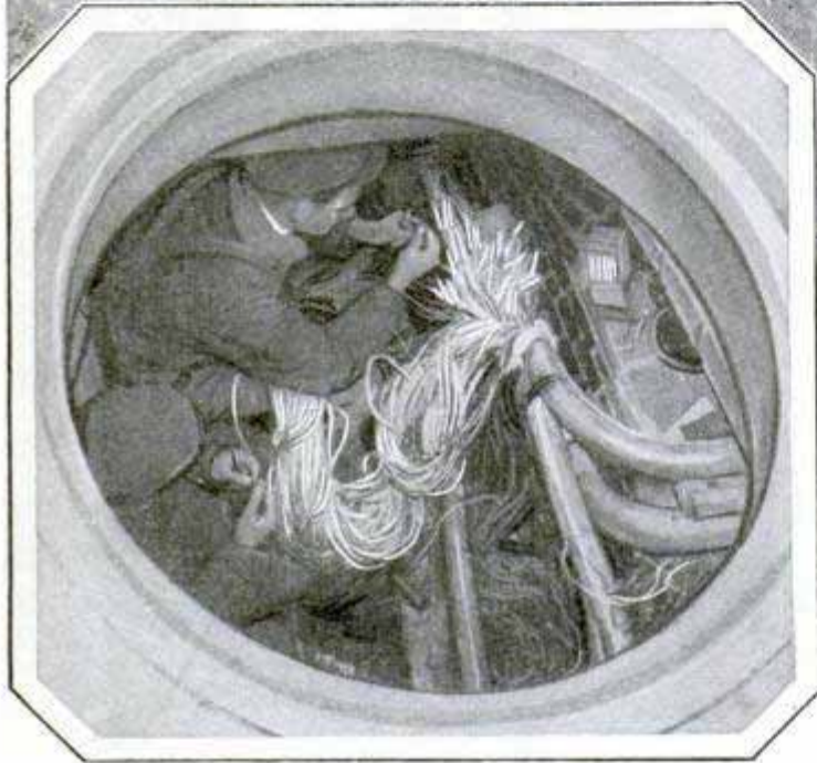
Stretching a Lead-Sheathed Cable, Above; Left, a Worker in a Manhole, Patching Wires beneath a City Street
