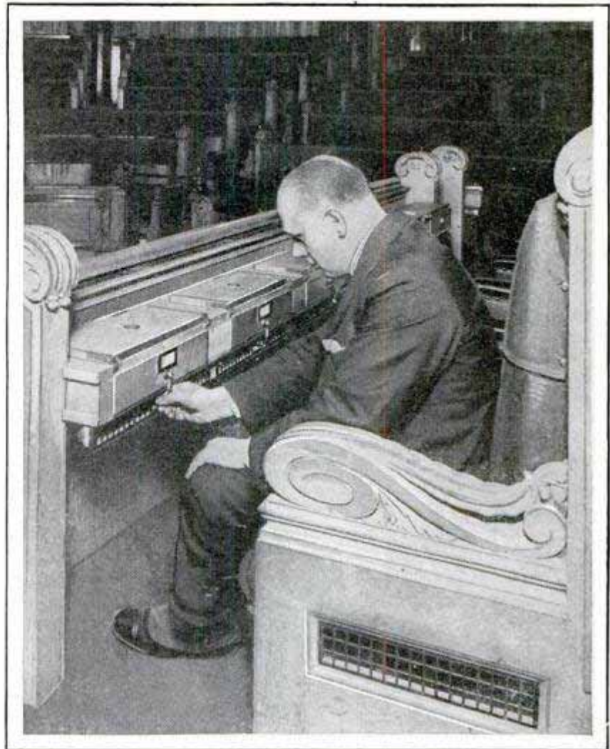
Manipulating Temperature and Ventilating Controls in London Town-Council Room; Each Member Can Adjust "Weather" to Suit Himself
