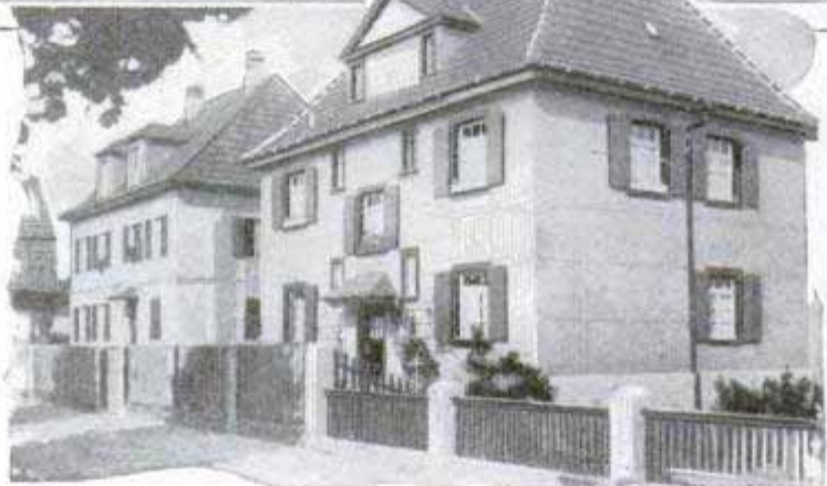
Two Stages in the Construction of the Steel and Turf Houses, and Completed Dwellings Showing Homelike Appearance
