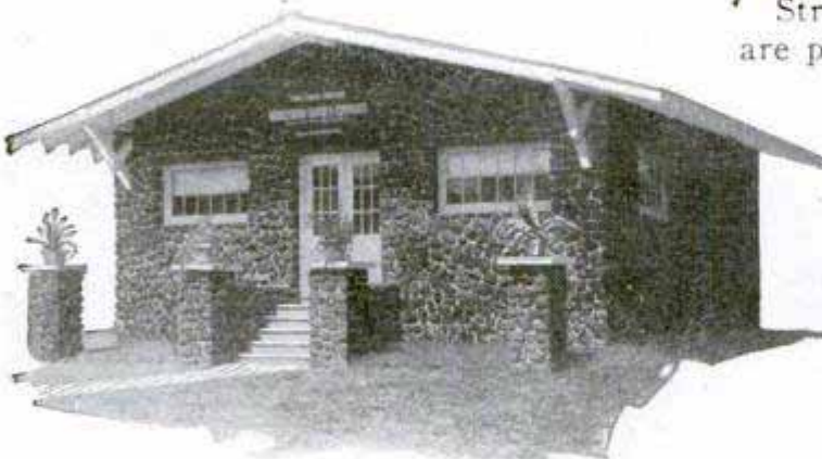
Kentucky House with Walls Made of Lumps of Coal; a Pleasing Contrast Was Gained with White Mortar
