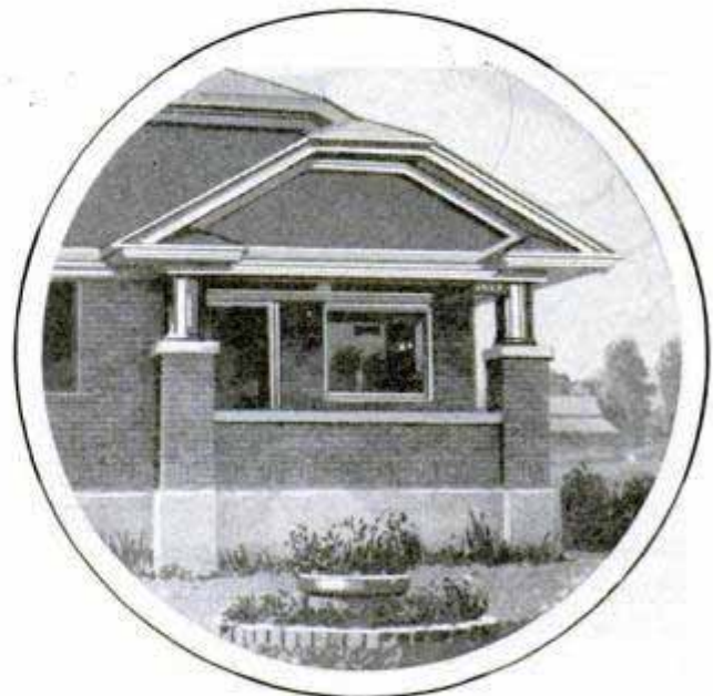
Glazed Drain Tile Can Be Used Successfully as Porch Pillars
