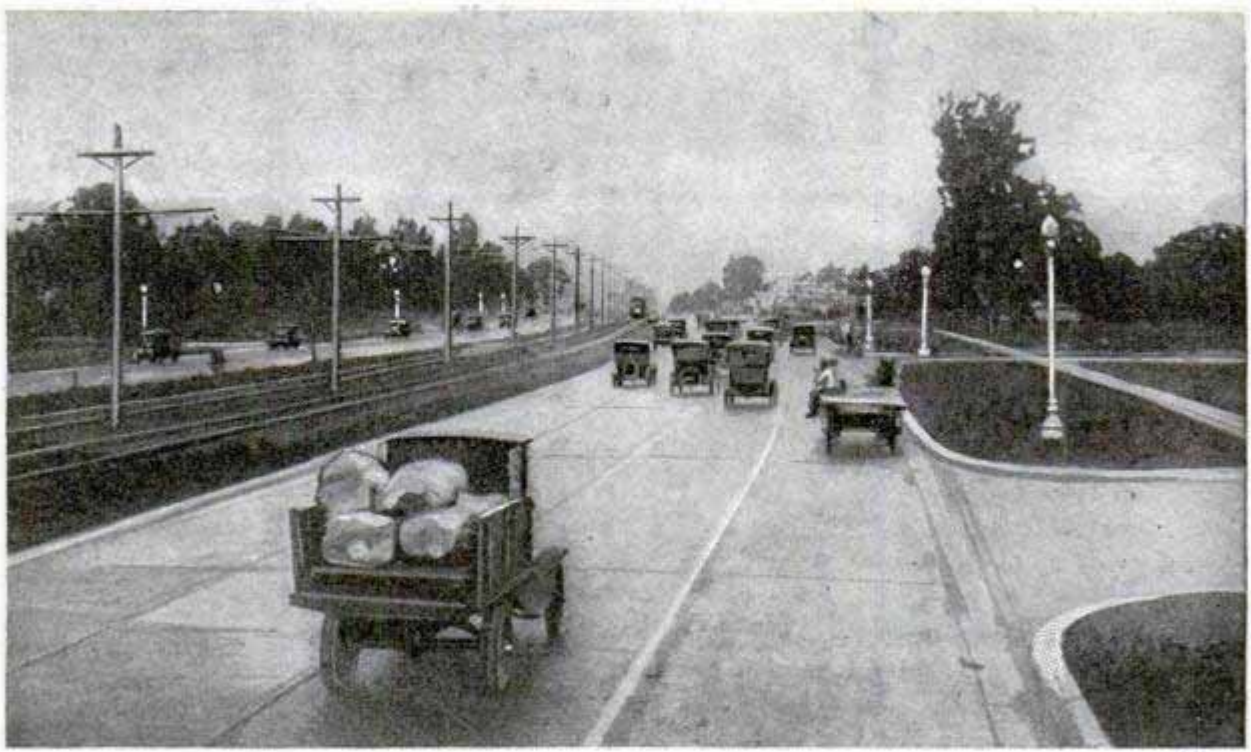
Wide Double Highway in Michigan, with Car Tracks between One-Way Pavements. Provides Lanes for Slow, Medium and Fast Traffic; the Road Connects Two Auto-Building Cities
