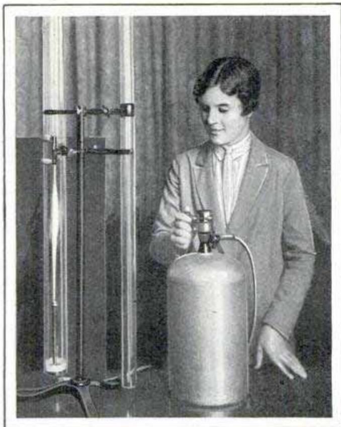
Sensitive Flame at Left and, Right, Microphone That Transmitted Voice to Extinguish the Blaze, Which Was Twelve Miles from the Broadcasting Station
