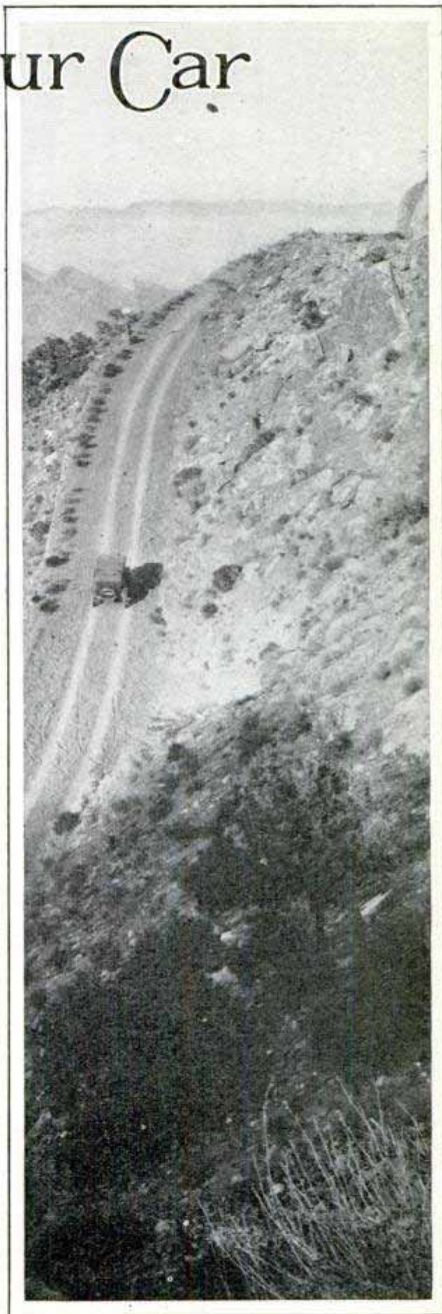
The Pechecio-Pass Road in Lower California
