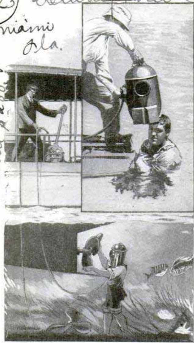
Adjusting the Helmet, and Illustrating How It Could Be Used in Repairing a Propeller
