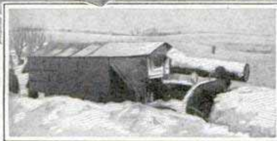
Snowplow Truck, Showing Fans and Sighting Tube
