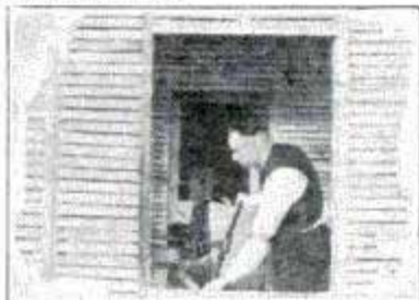
View of part of the interior of the bungalow for practicing house wiring—right in the Greer Shops. You learn here by real experience—with an expert always at hand to show you how.
