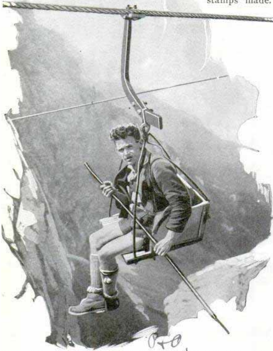
Worker Making a Test Run on Cable That Hauls Persons to the Top of an 11,000-Foot Peak in Germany
