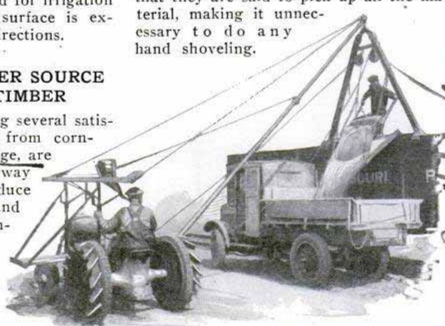
Tractor-Scraper Rigging for Unloading Cars of Loose Material; Entire Outfit Is Easily Moved to Another Car and Attached
