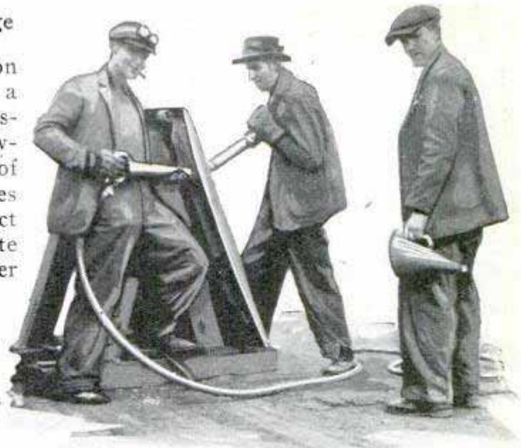
Special Frame for Holding Dump Doors Aids Riveters
