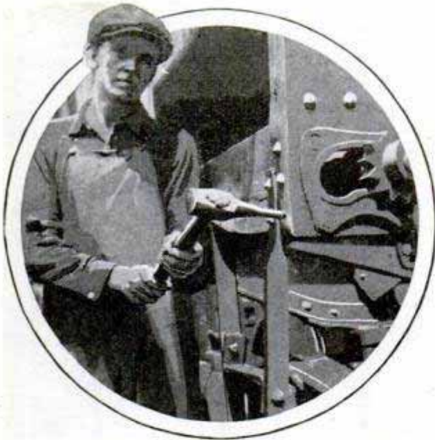
Old Hammers Drawn Out Make Good Tools for Removing Rivets
