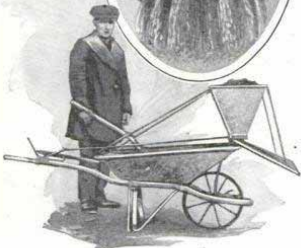
Wheelbarrow Sander Attachment in Operation, and Side View Showing Connections
