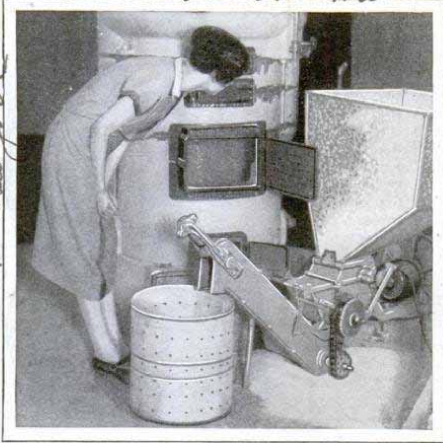
Examining the Electric Stoker; Fuel Bin Is Seen at Right, with the Ash Chute in the Foreground, and Motor under Hopper.
