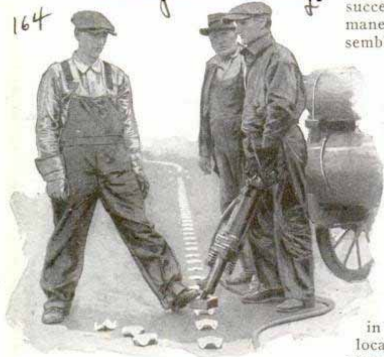
New Form of Metal Traffic Marker Is Easily Driven In with an Air Hammer
