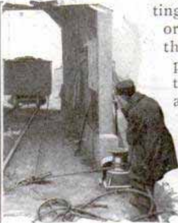
View of Puller on Small Truck and in Use in Railroad Yard Setting a Freight Car
