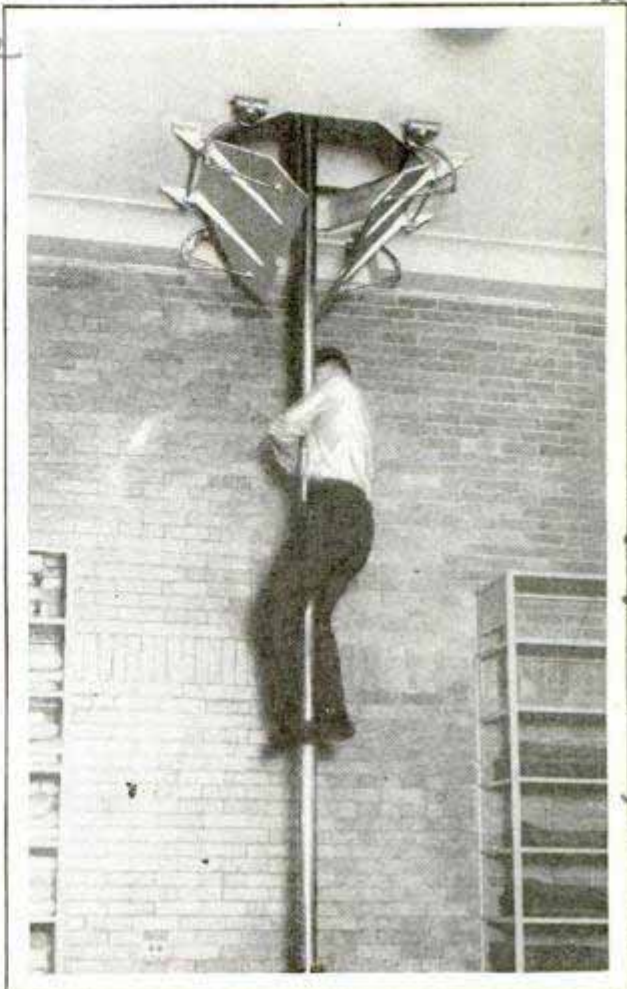
After Fireman Has Passed Through, the Trapdoors Automatically Close, Shutting Out Drafts
