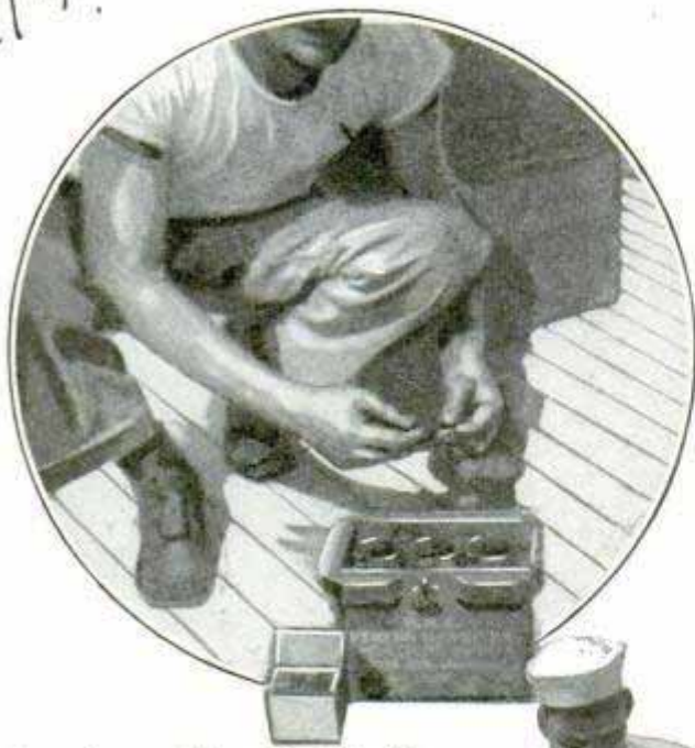
Preparing to Mine a Derelict; the Detonator, Top, Is Being Inserted in a 1,500-Pound Mine in the Center; Below Is the Cable and a Small Mine
