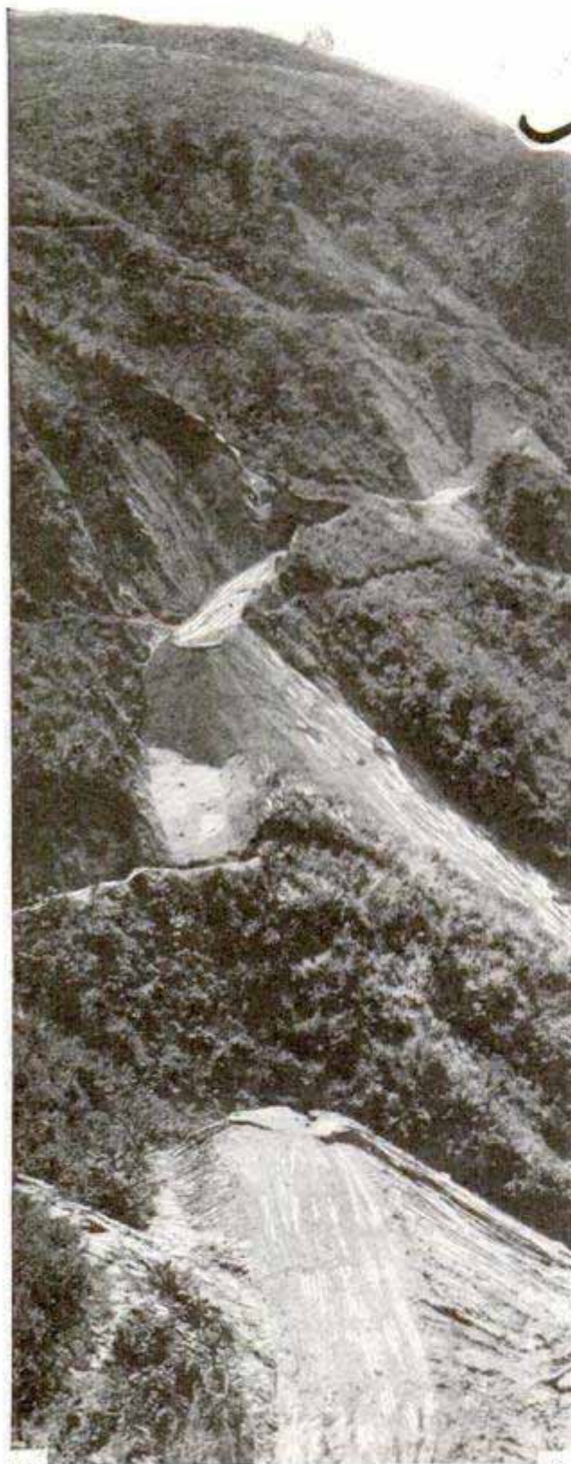
View of Construction Line
