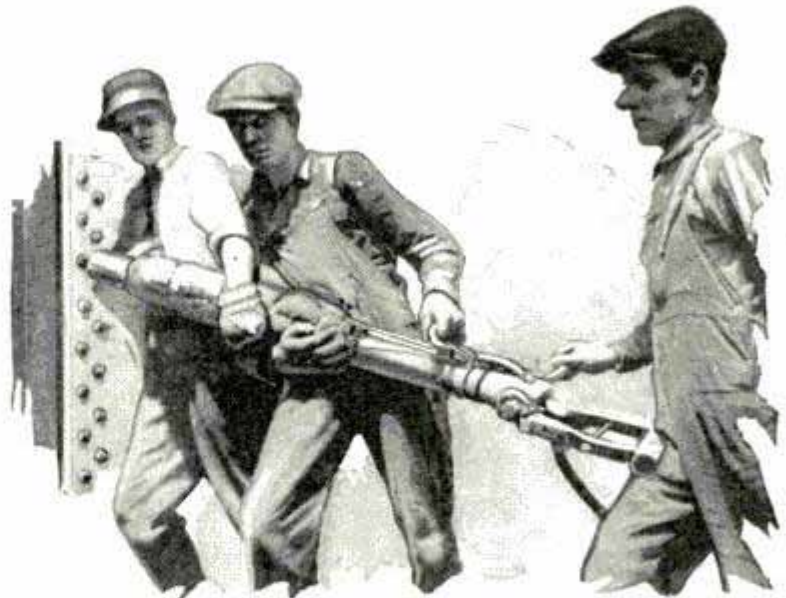
Lightening the Task of Handling a Heavy Air Hammer by Burlap Padding and Heavy Rubber Tube
