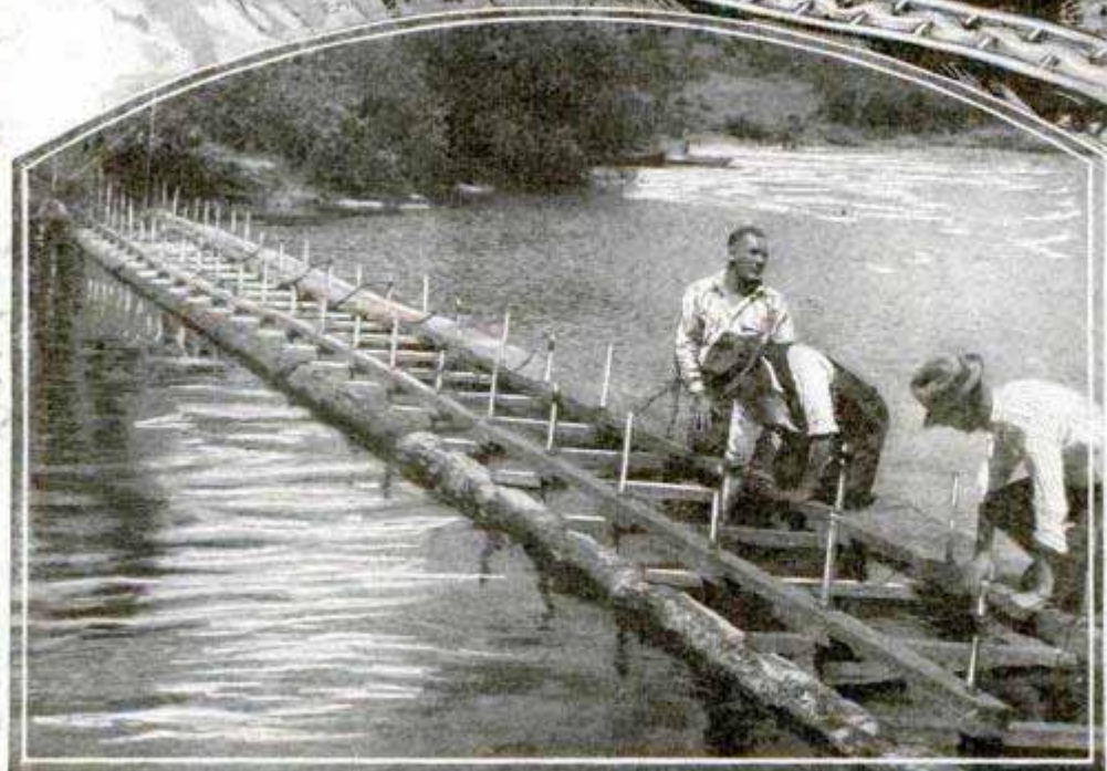
Drawing of Electric-Dam Installation on Rogue River, Oregon, to Keep Fish from Entering the Turbines, and Photograph Showing Arrangement of the Charged Rods; Shocks Drive the Fish from the Danger Area into the Ladders That Lead Downstream
