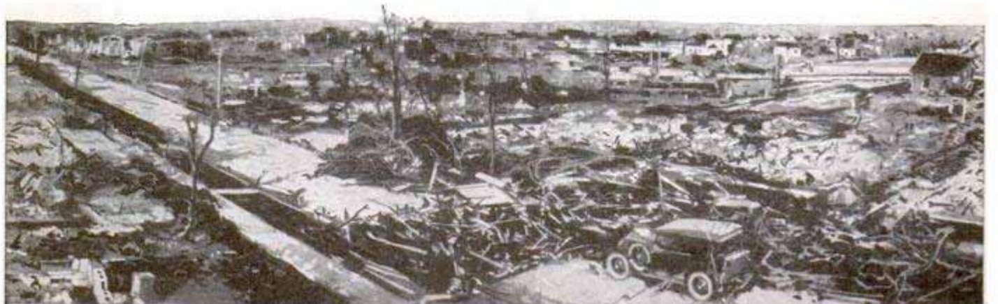
Murphysboro, Illinois, as It Looked after the Tornado Last Year, When a Large Part of the Town Was Wiped Out, and, at Top of Page, as It Was Rebuilt with Red Cross Aid
