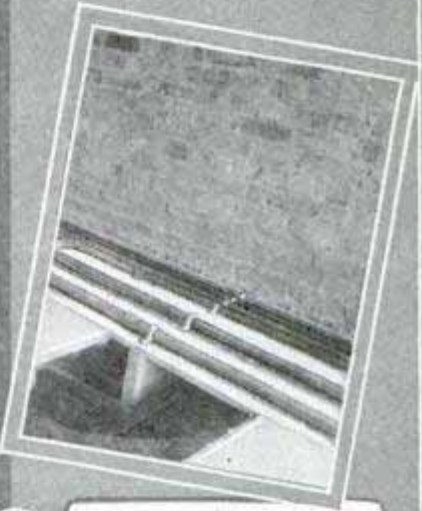
Pipes Held on Floor to Prevent Moving
