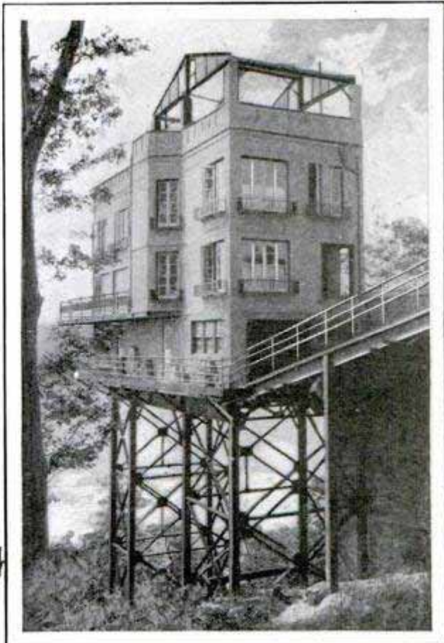
How Steel Is Aiding the Home Builder; Stilts under House on Bank of Hudson River
