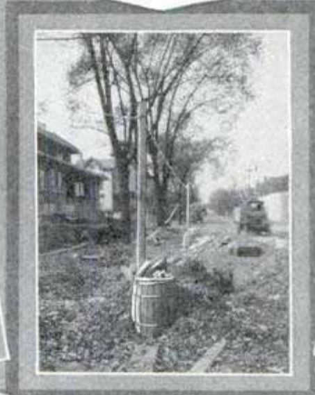
Stone-Filled Barrels for Temporary-Line Poles
