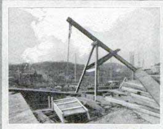
Quickly Erected or Dismantled Wooden Derrick
