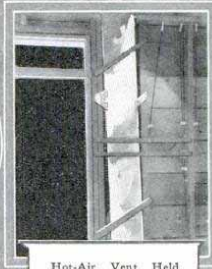
Hot-Air Vent Held Securely by Ears
