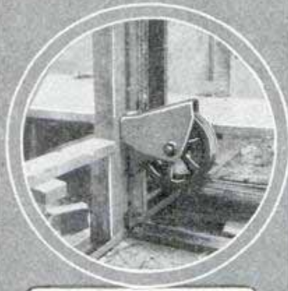
Hood over Pulley Protects It from Debris
