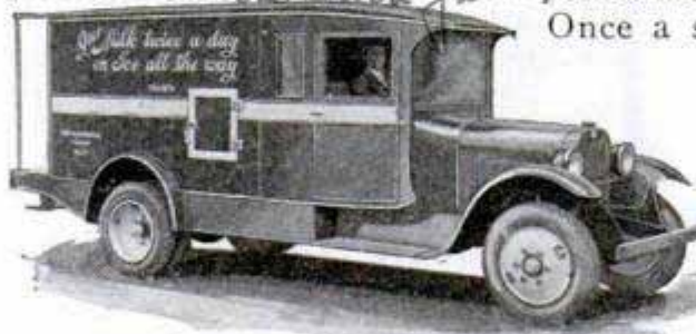
Big Brine Tank in This Motor Truck Keeps Milk Fresh on Long Hauls from Dairy Farm
