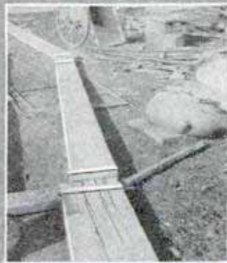
Strap Irons on Plank Ends Prevent Splitting
