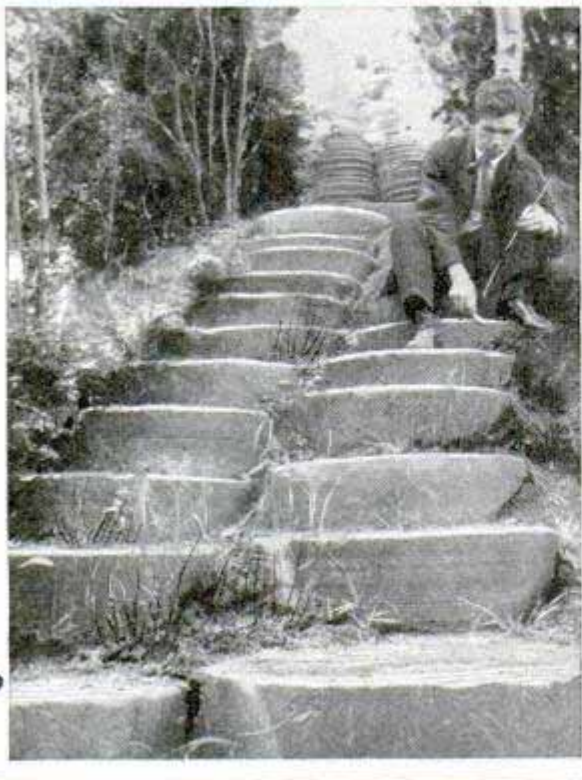
Old Grindstones Form Serviceable Stairway as Their Thickness Is Right for an Easy Step
