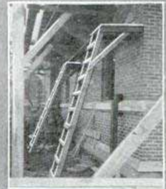
Convenient Platforms for Cornice Builders
