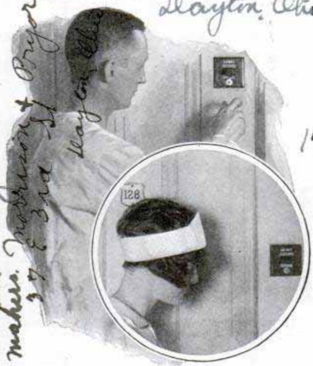
Hotel Guest Setting the Dial from Inside Room and Maid Reading the Indicator
