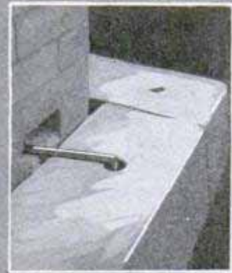
Holding Stone Veneer to a Brick Wall
