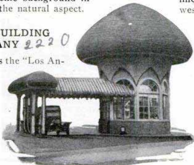
Stucco Gasoline-Filling Station with Mushroom-Shaped Roof; the Shingles Are Arranged like Thatch
