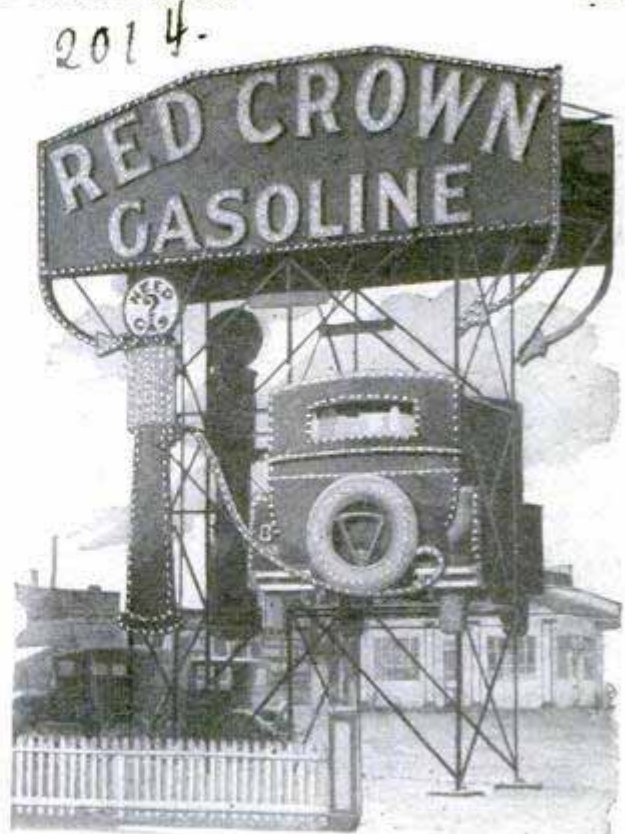
Successively Flashing Lights Lead from Imitation Pump to "Tank" on Auto, Part of Filling-Station Sign
