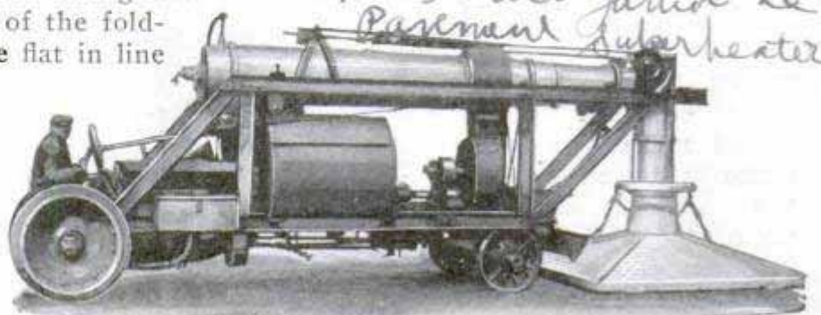
At Work on Asphalt Pavement with the Oil-Burning Heater
