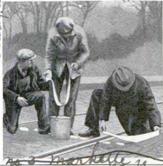
Laying Canvas Strips as Traffic Markers Instead of Painted Lines; Adhesive Holds Them to Pavement
