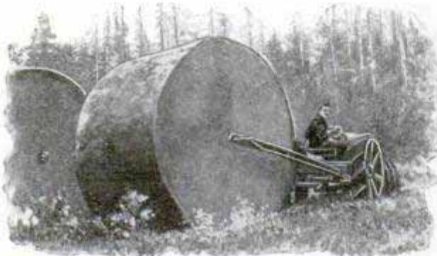
Rolling Huge Blocks from Forest to Mill with a Tractor Linked to Their Centers
