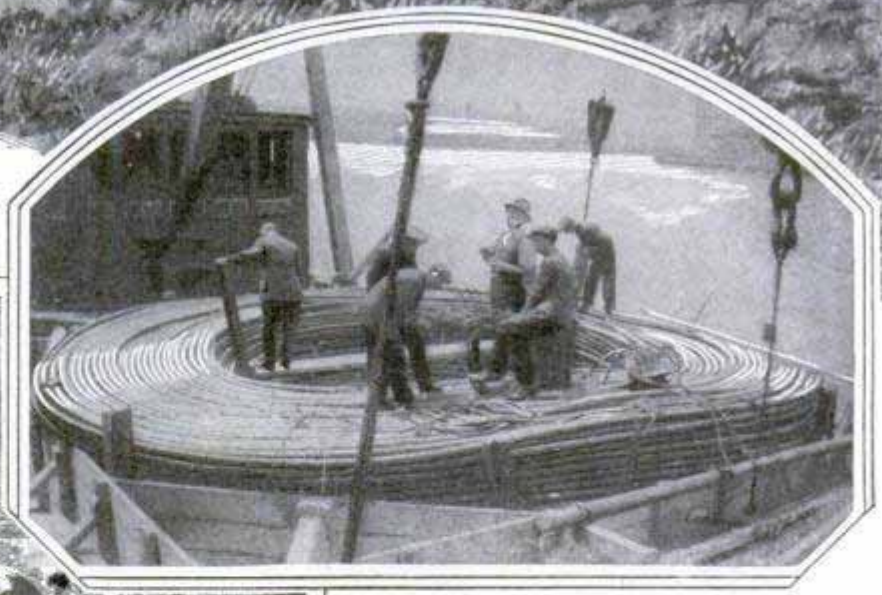
In Laying the Shore End, Barrel Buoys Temporarily Support the Line Until It Is Connected; a Coil Containing Seven and One-Half Nautical Miles of Cable; at Left, Buoy to Mark the Course; on Op- posite Page, Inset, Grapple to Hoist Cable and Cable Ship "Faraday"
