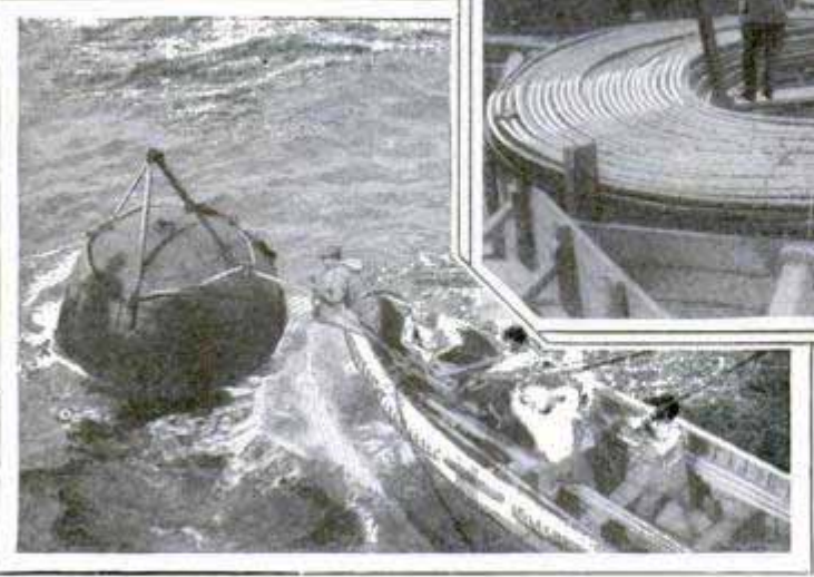
In Laying the Shore End, Barrel Buoys Temporarily Support the Line Until It Is Connected; a Coil Containing Seven and One-Half Nautical Miles of Cable; at Left, Buoy to Mark the Course; on Op- posite Page, Inset, Grapple to Hoist Cable and Cable Ship "Faraday"
