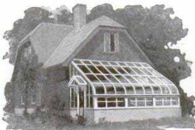
Conservatory Added to Dwelling; Parts Are Prepared Ready for Assembly
