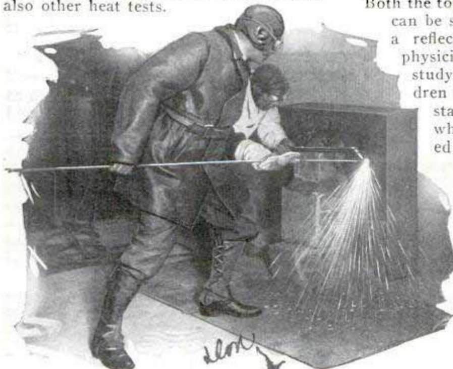
Trying Vainly to Melt the Steel with Torch
