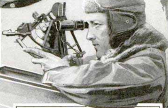
Byrd Using the Special Sextant from the Plane's Observation Seat; This Instrument Had a Horizon All Its Own, Making the Navigator Independent of the Natural Line
