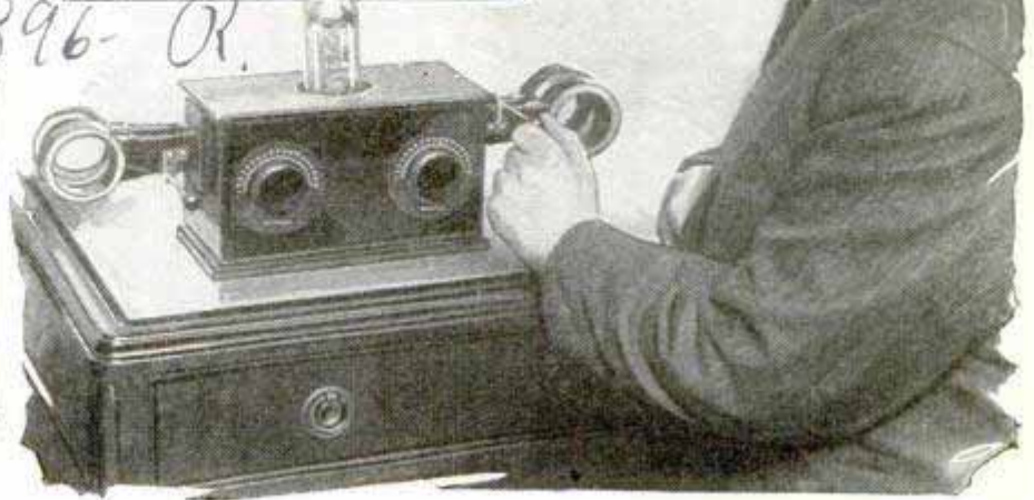
Furniture David R. Lowe, of Berlin, Demonstrating New Radio Tube Combining Detector and Two Stages of Amplification; Tuning Coils Complete the Set; Left, Tube Showing Six-Prong Base
