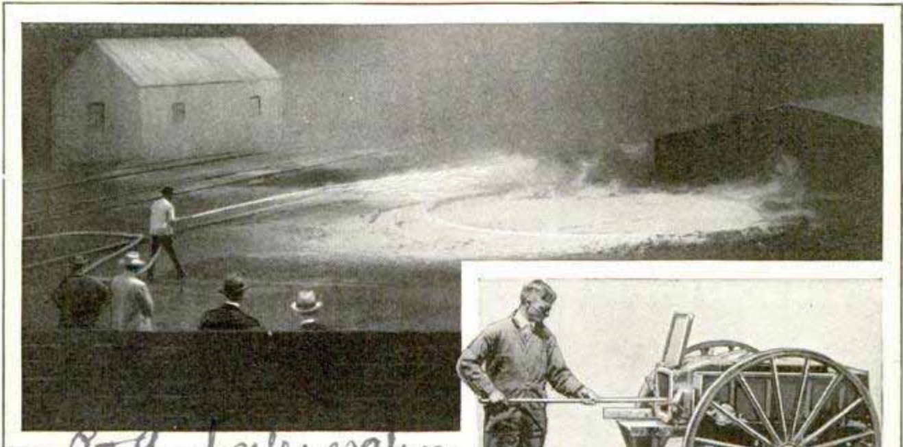
Conquering the Blazing Pool of Oil with Stream of Foam, and Close View of the "Gun"
