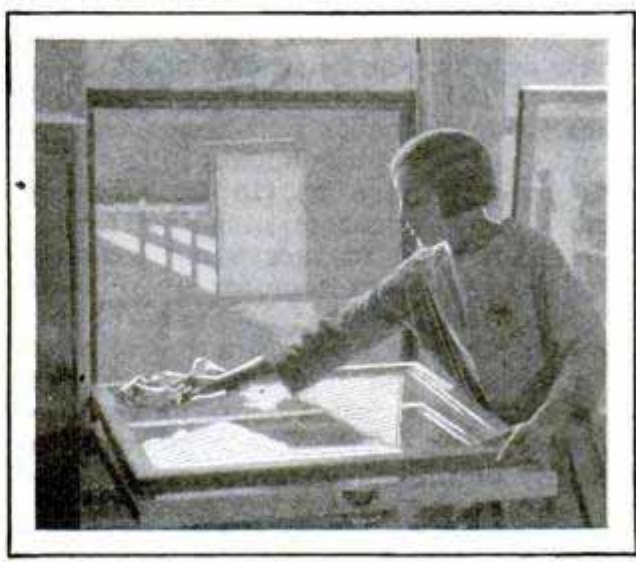
Window Swung Inward for Washing
