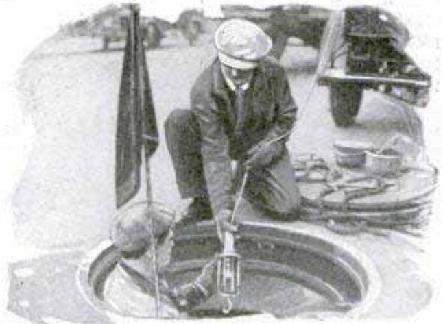
Special Six-Volt Lamp on Extension Cord for Lighting Manholes
