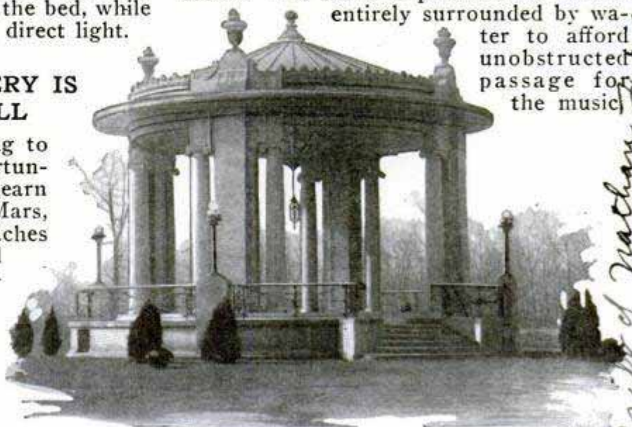
New Bandstand in St. Louis Park; Constructed of Copper and Stone, It Is Intended to Insure Successful Concerts
