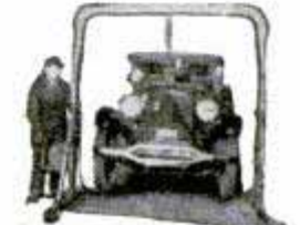
Using a Weaver Crane—on the repair floor
