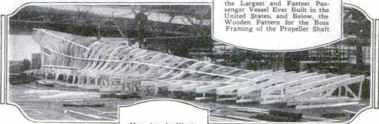
Here are the Workmen Making the Wooden Pattern for the Main Deck of the "Malolo"; Every Part of a Ship is First Laid Out on the Floor of the Pattern Loft
