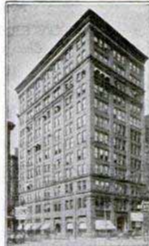
Our Pittsburgh Office Suite 514 Empire Building
