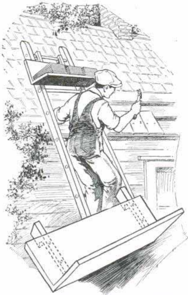
Wooden Rack on Ladder Rung Holds Shingles
