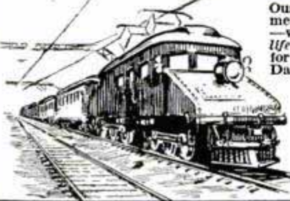
New electrified railway near the Greer Shops
