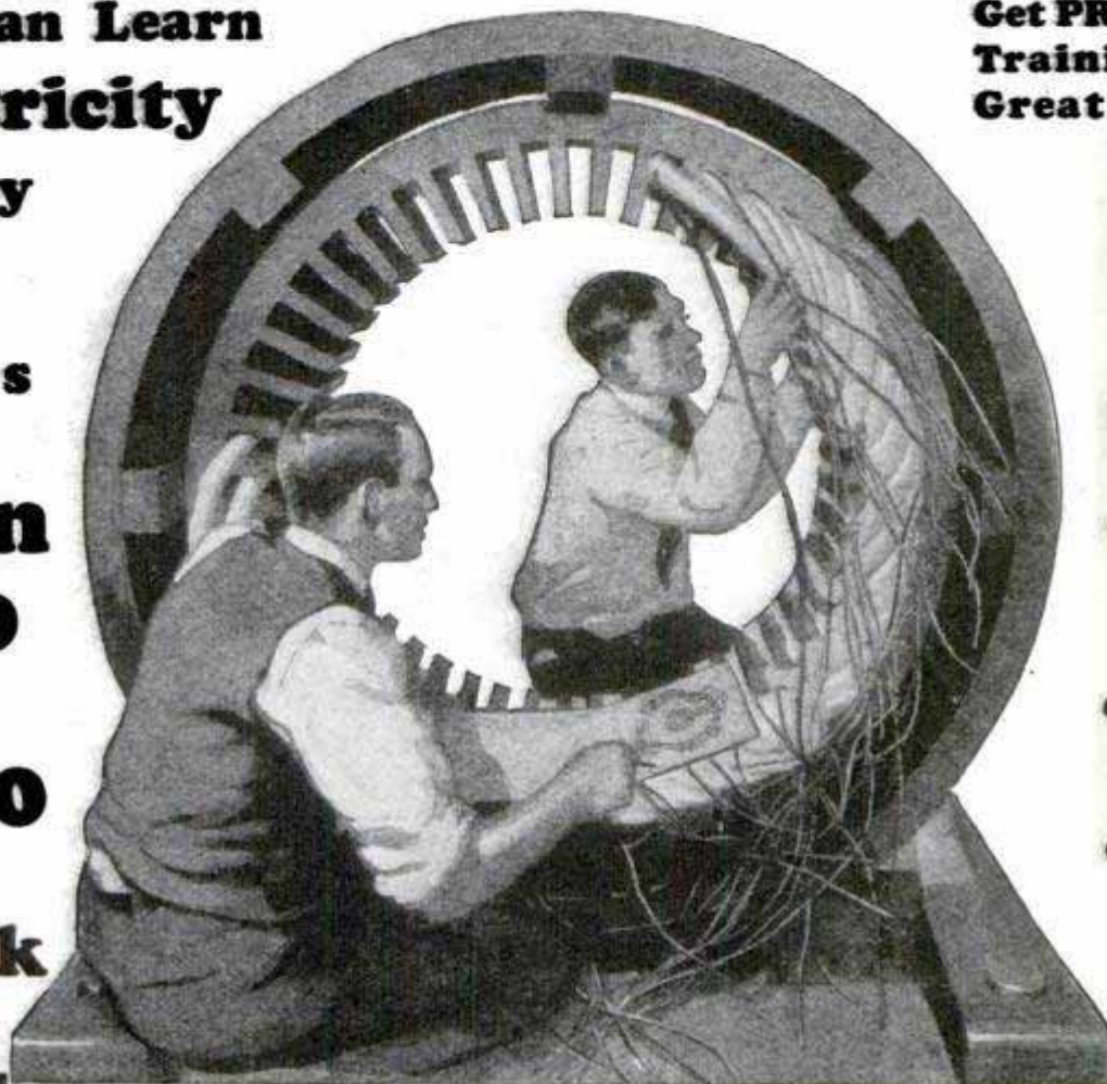
Student Winding Stator
