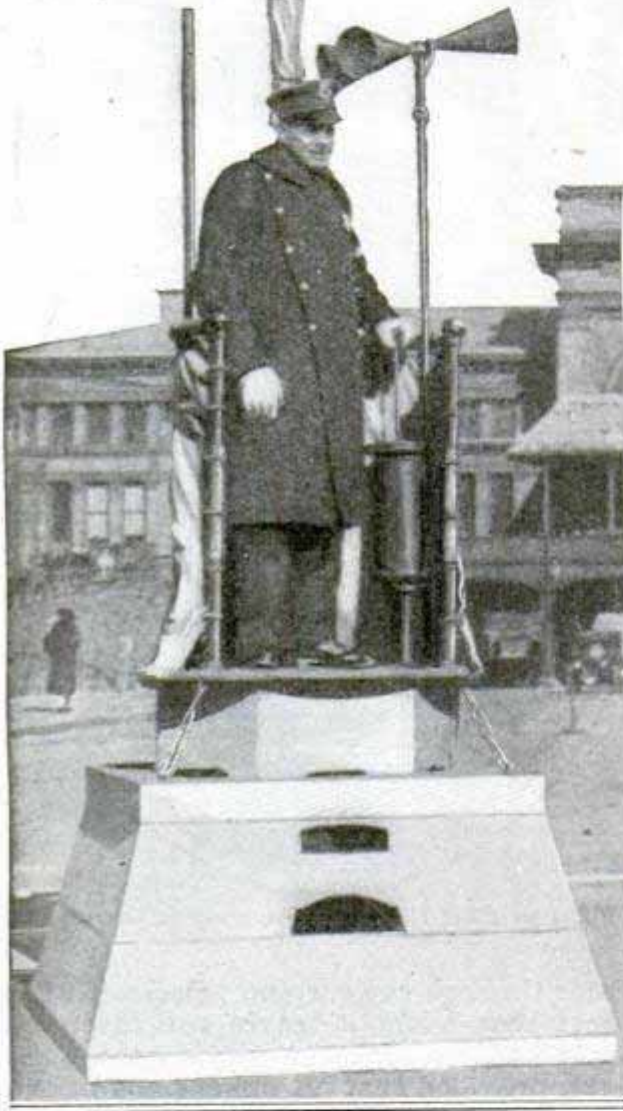
Policeman on Pedestal with Whistle Plunger in Left Hand; Sound Is Carried to All Parts of Square
