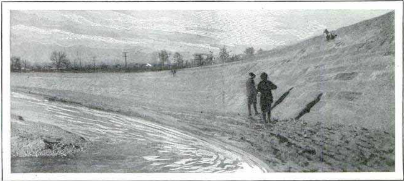
Flood Banks of Western River Protected Effectively against Scour by Paving with Curbstones That Were Too Worn to Be Used in Street-Improvement Work
