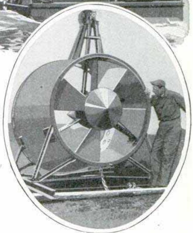
Turbine on Float Ready for Placement in Current and a Close View of the Wheel
