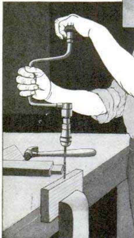
Above, Chiseling Out the Mortise; Left, Making the Mortise by Boring
