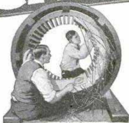
Student Winding Stator at COYNE
