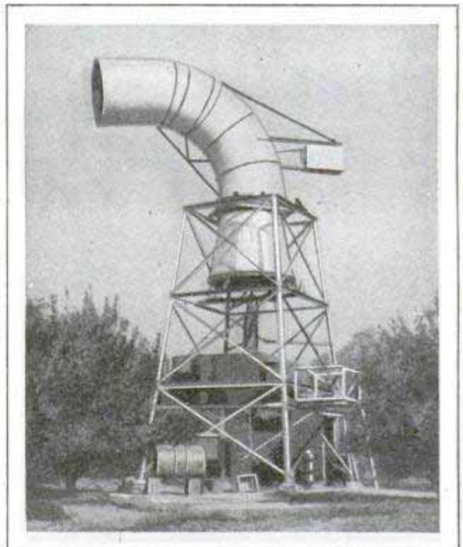
Left, Type of "Windjammer," Which Brings Down Warm Air from Above and Spreads It over the Ground; Right, Another Type That Sends Warm Air above Tree Tops; Both Use Airplane Propellers
