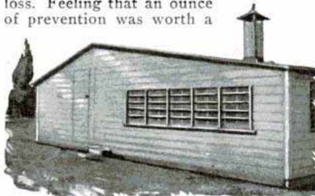
Old Pipe, Held in 2 by 4-in. Brackets, Protects This Poultry House against Thieves
