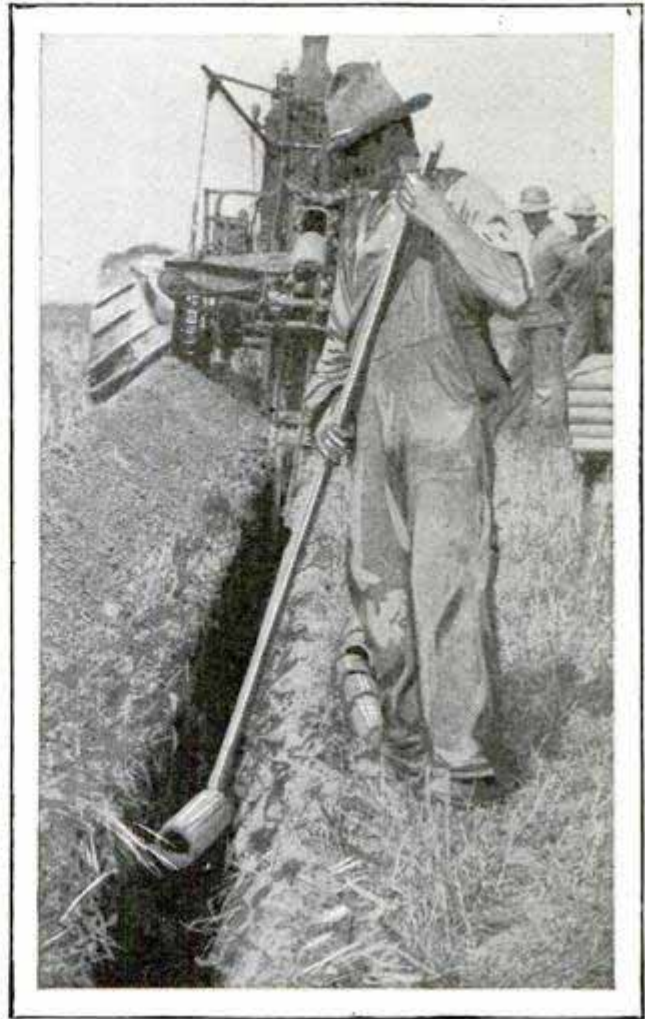
Easily Made Tile Hook Facilitates Laying Drain Tile in Deep Ditches
