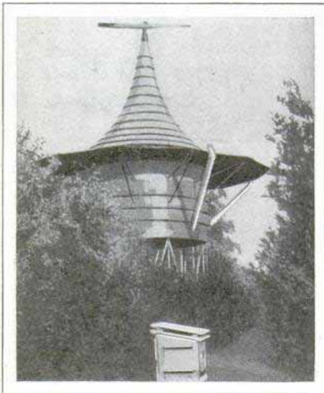
Left, Type of "Windjammer," Which Brings Down Warm Air from Above and Spreads It over the Ground; Right, Another Type That Sends Warm Air above Tree Tops; Both Use Airplane Propellers
