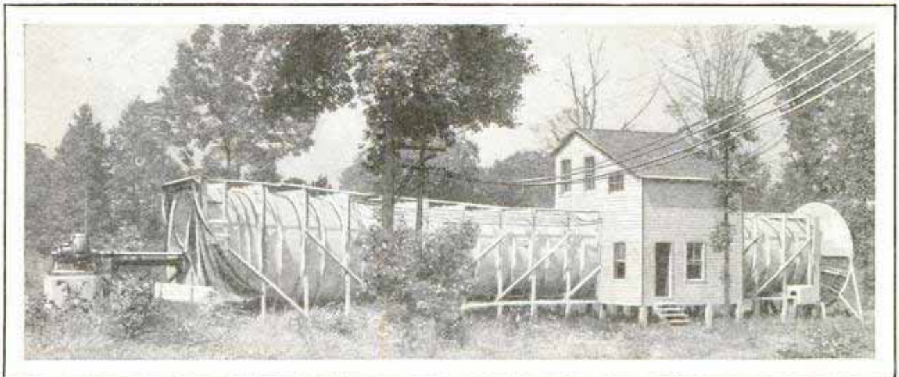
Huge Wind Tunnel of the Bureau of Standards at Washington, Used to Test Building Models and Determine Exact Figures on Gale Pressures Their Walls Must Stand
