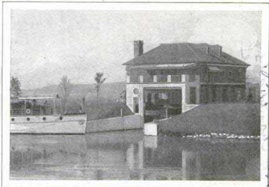
Motor Launch Entering Its Dock through Wide Back Door of Residence; Pumped Dry in Winter, the Space Holds Cars
