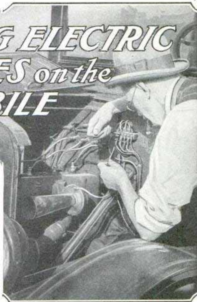
Connecting Accessories to the Ford Manifold Terminal Block
