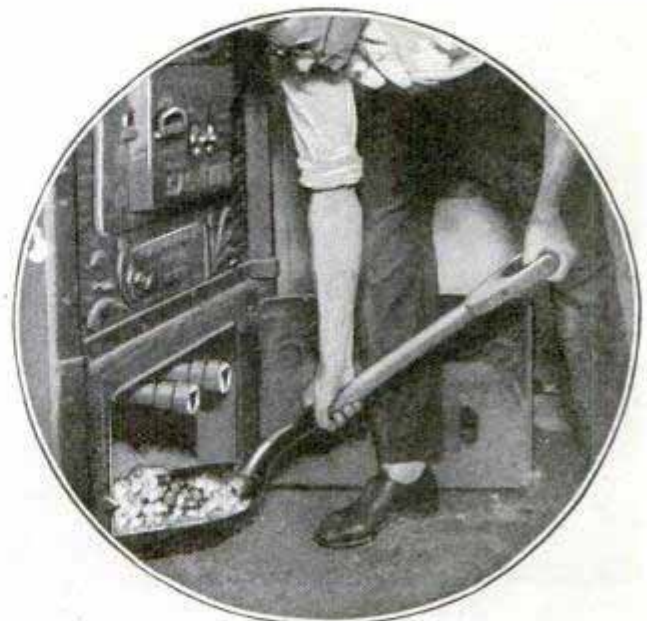
Keep the Ashpit Free from Ashes and Clinkers to Permit the Air to Get to the Fire
