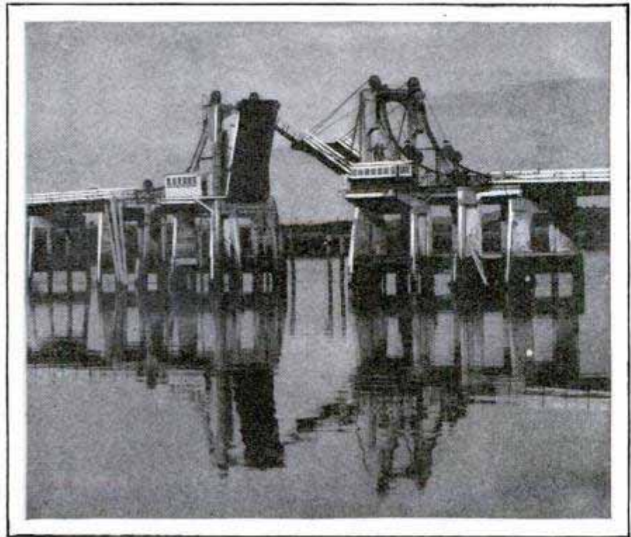
At the Center of the Bridge Are the Lifts, the Detours Are a Third of the Way from Each End
