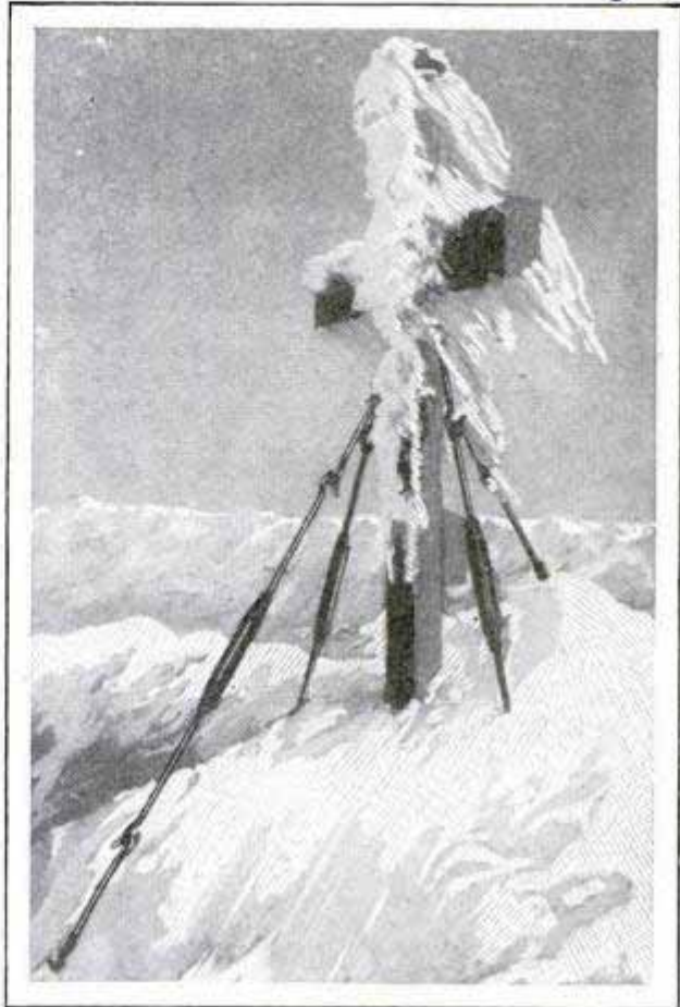
Defiant of Winter Storms, Iron Cross, Guyed to Rocks, Caps Alpine Mountain Crest
