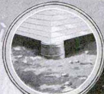
Old Nail Kegs Make Pier Forms
