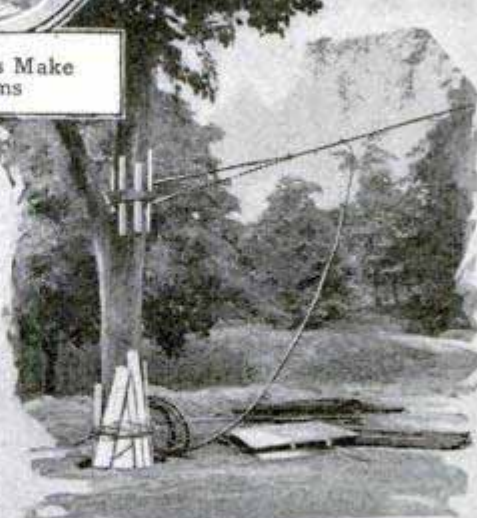
Preventing Cable from Cutting Tree
