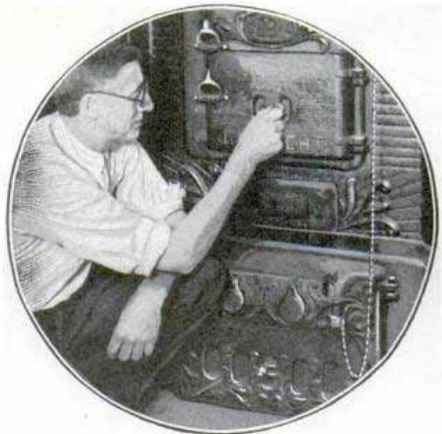
The Feed-Door Damper, Which Supplies Air above the Fire, to Aid in Combustion
