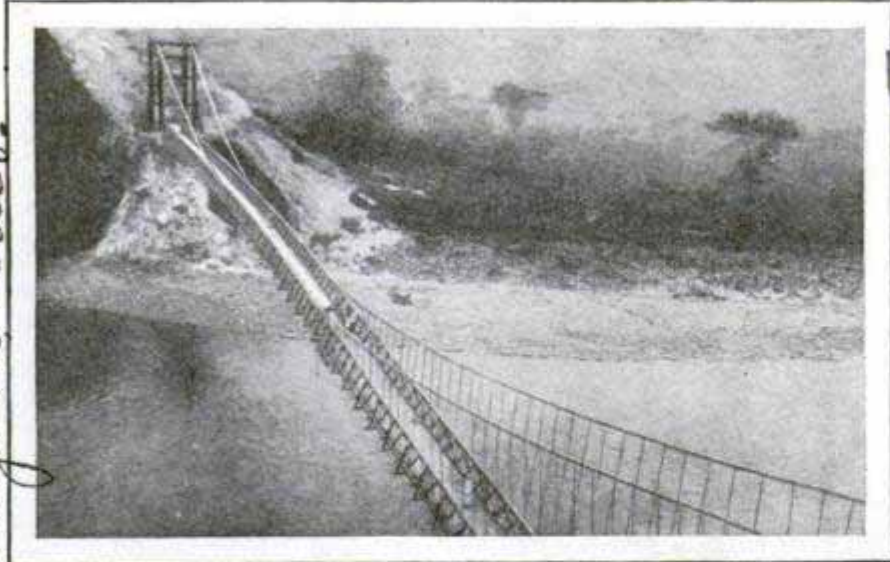
South American Suspension Bridge, Five Hundred Feet Long, Is Tied Together Wholly with Knots, No Nails Being Used
