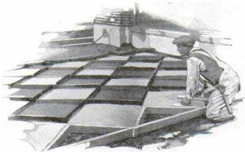
Large Squares of Different-Colored Cement Make an Unusually Attractive Sidewalk
