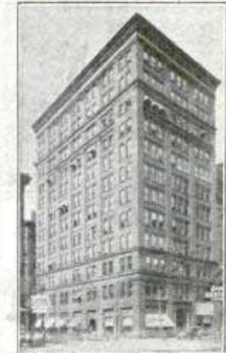
Our Pittsburgh Office Suite 514 Empire Building
