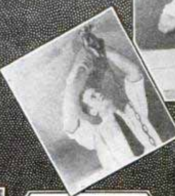
Here a student is doing a house-wiring job—installing a ceiling fixture.
