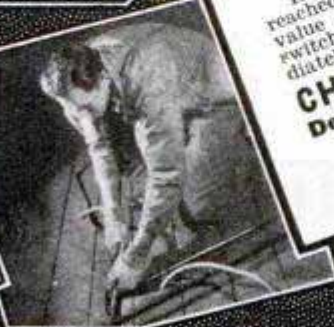
One of these outfits is a $10 motor. Same type as the big fellows in a power plant. You wire the commutator and the field, assemble it, change the voltage from battery to power current, make it run, change it over into a generator
