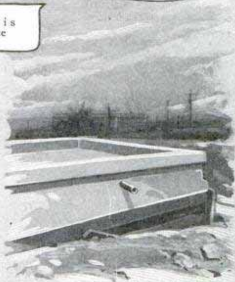
Pipe Drains Porch Floor
