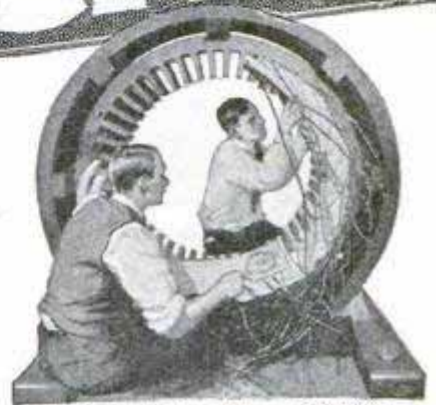
Student Winding Stator at COYNE
