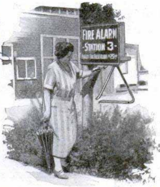
One of the Triangle Fire-Alarm Signals That Tell Location of Blaze by Their Pitch
