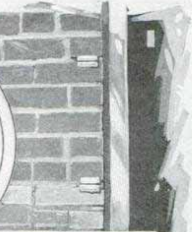
Sheet-Metal Bracket Holds Nails in a Brick Wall
