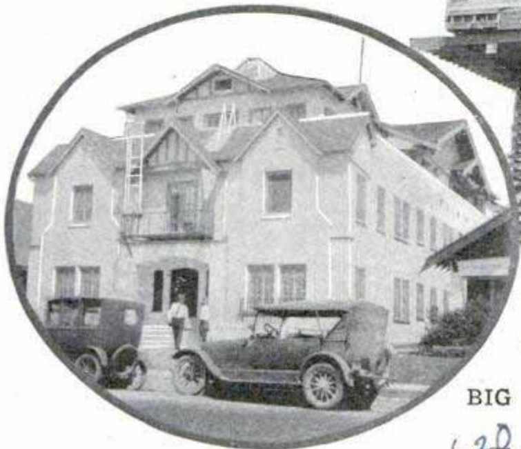
Bungalow on Props and on Rear of Roof of Apartment House Built under It
