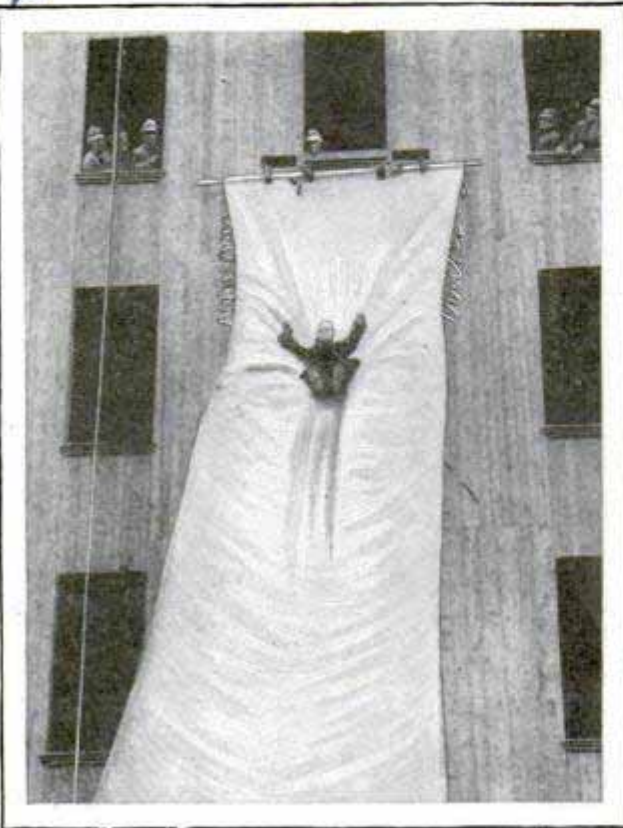
Demonstrating Use of Asbestos Chute as Means of Escape from Burning Building
