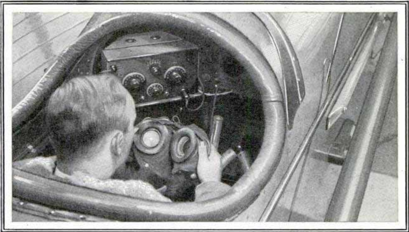
The Air-Mail Pilot's Headphones Are Built Right into His Helmet, So That When He Puts It On, He Is Ready to Tune In on the Radio Receiver in the Corner of the Cockpit
