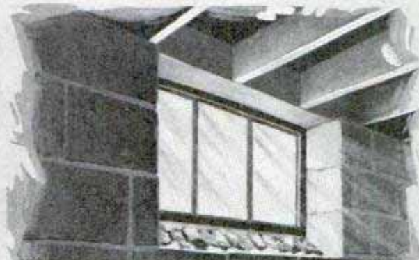
Beveled Sill of Basement Window Admits More Light and Makes Neat Job; Finished with Cement
