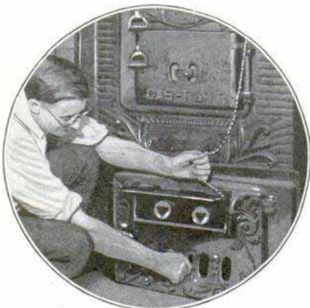
There Are Two Draft Dampers in This Ash-pit Door, for Better Regulation
