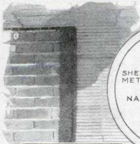
Wire Lath at Joint Prevents Cracks in Finished Plaster
