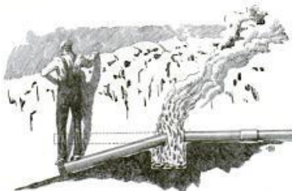
Novel Method of Bending Gas Mains in Trenches to Conform to Grades
