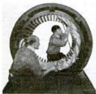
Student Winding a Stator
