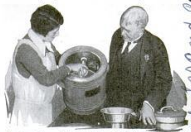
Demonstrating Electric Cooker Which Utilizes Heat of Light Bulb Attached to Socket in Side
