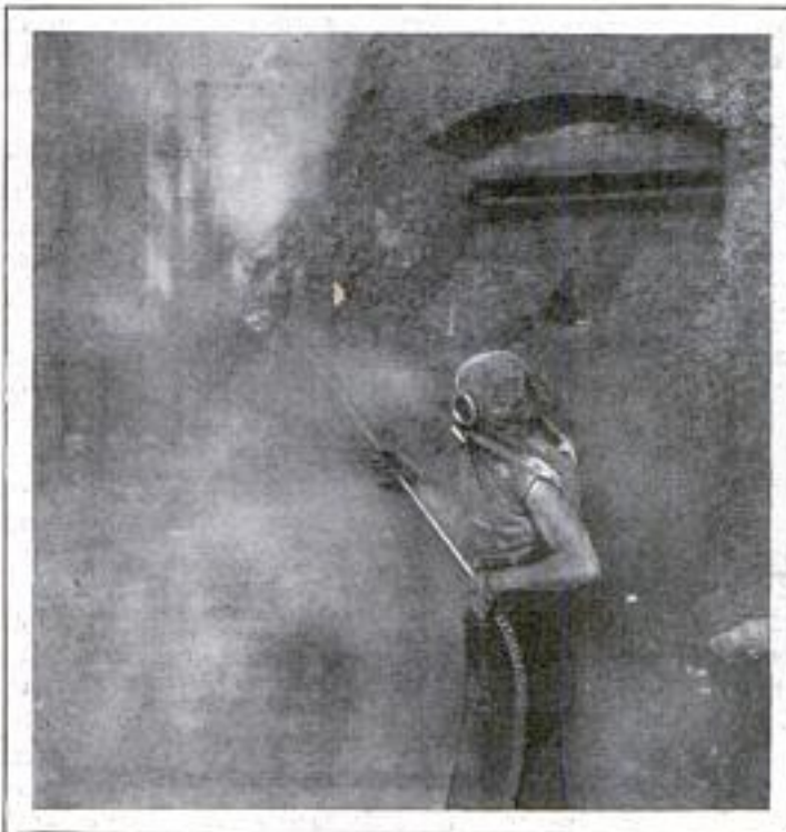
Face Mask Protecting Worker Cleaning Dusty Pit
