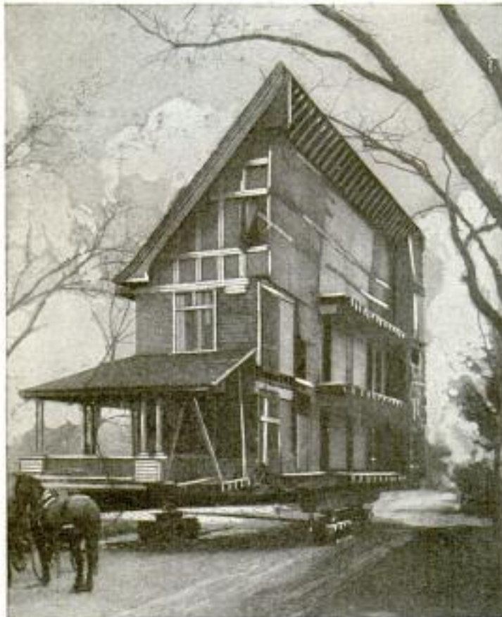
When Houses Are Too Wide, the Mover Saws Them in Half, Moves the Sections and Then Rejoins Them
