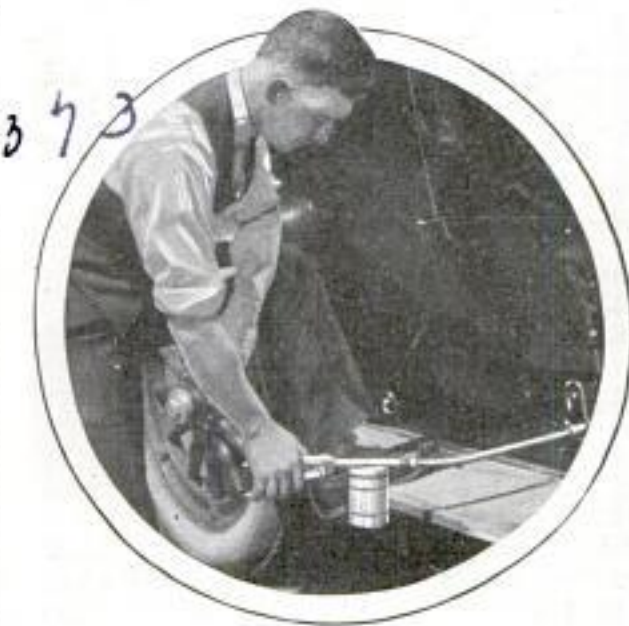
Greasing Auto with One-Hand Gun Operated as Pump
