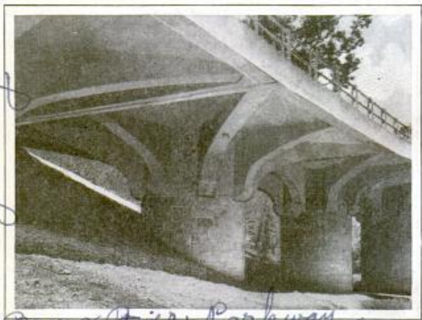
Round-Pier Automobile Bridge with Buttressed Concrete Roadway Intended to Support Heavy Weights with Little Vibration
