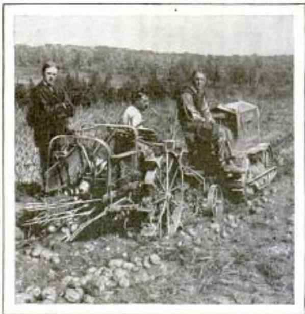
As Digger Is Drawn along by Tractor, Potatoes Are Piled in Row for Quick Gathering
