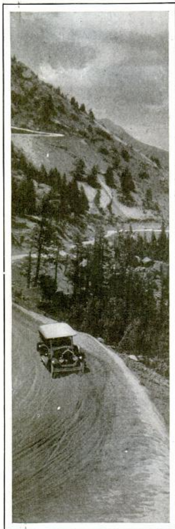
Broad Turns, Sloping Inward and Protected by Heavy Walls Make the Numerous Turns Safe
