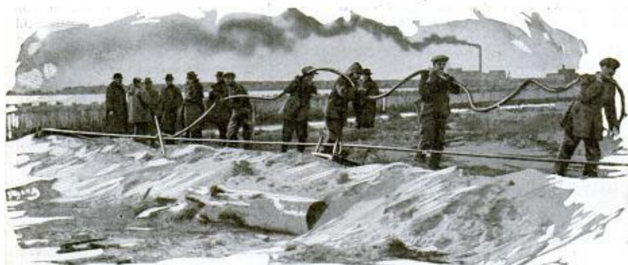
© U. & U. Dragging the New York End of the Cable up the Beach After It Had Been Landed by Small Boats and Floating Buoys; the Land End Is Built Extra-Heavy to Withstand Wear and Tear
