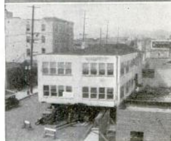
A Single Motor Truck Moved This Los Angeles Apartment House Twenty-Seven Blocks in the Night
