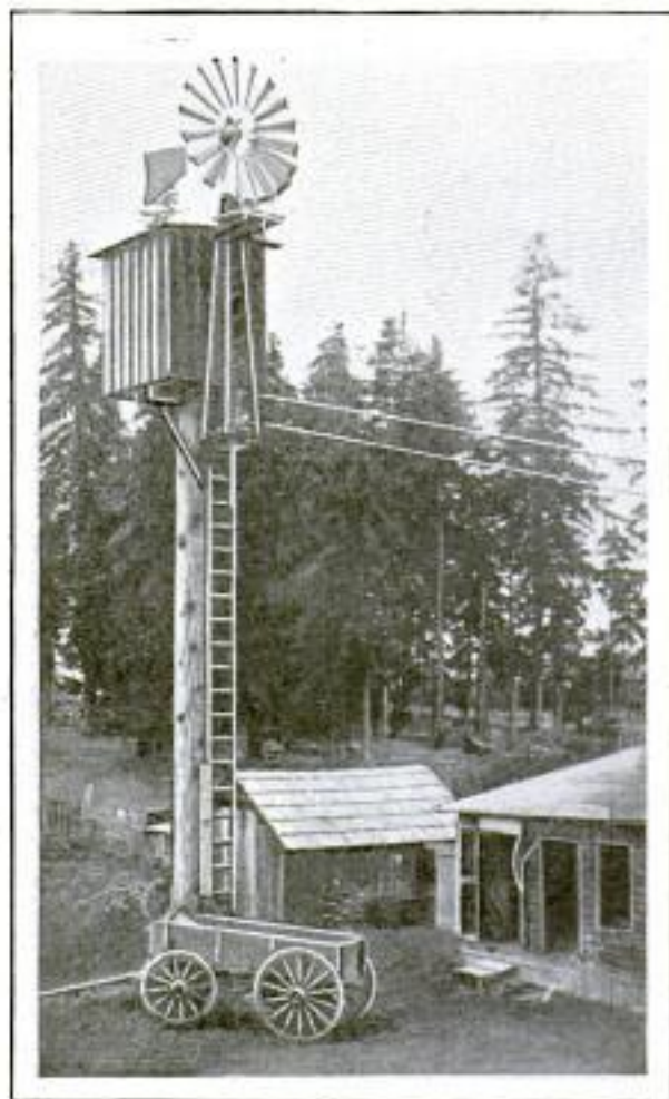
Water Tank and Windmill Built on Top of a 40-Ft. Fir Tree Have Given Service for 14 Years
