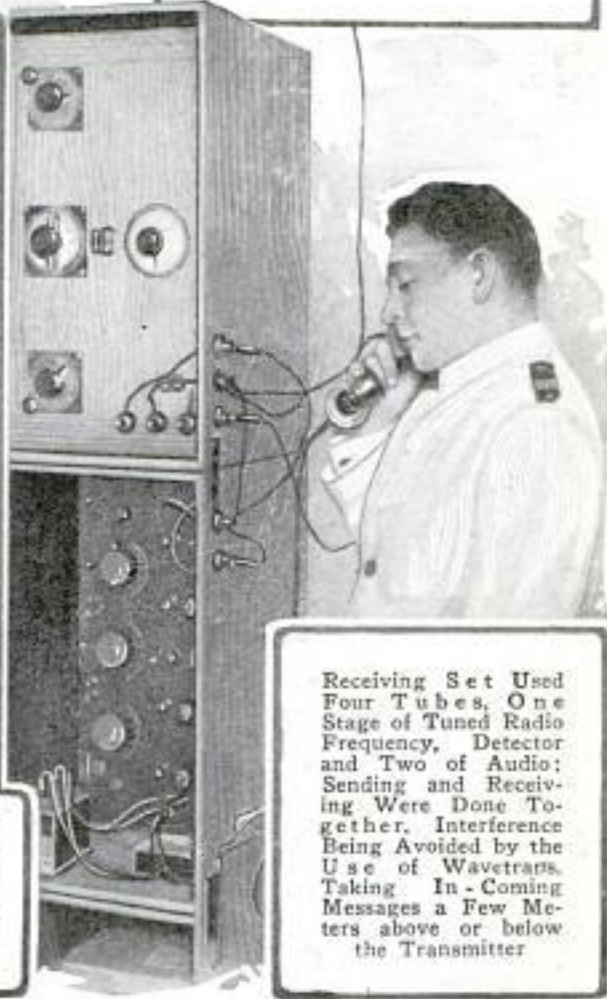
Steamer's Antenna Tuning Coil Is of Tapped Construction and, to Afford Greater Selectivity, a Huge Specially Designed Condenser, Seen at the Upper Left, Is Employed
