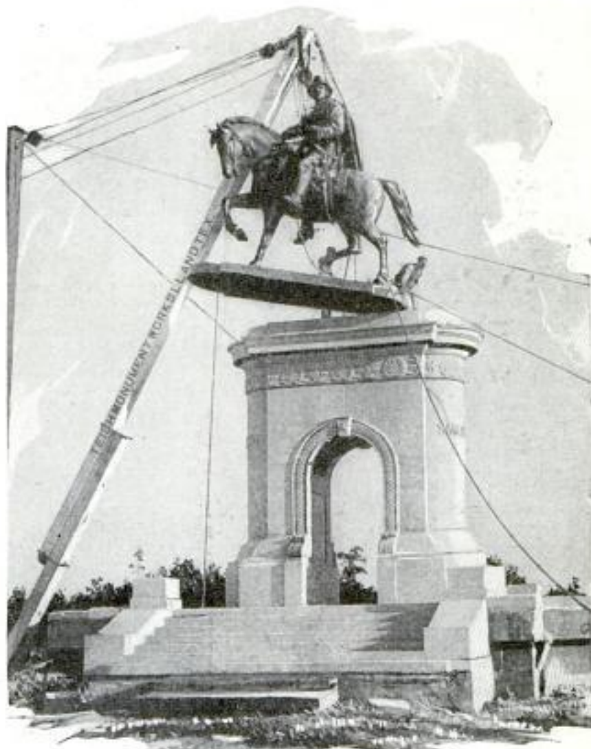
Swinging Huge Bronze Statue of Gen. Sam Houston to Its Position on High Stone Pedestal Arch with Strong Derrick
