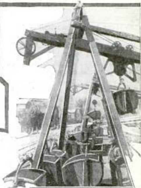
Tramway Machines, to Left, Displaced the Wheelbarrows, and Sent Their Steam-Operated Buckets Direct into the Hold, to Be Filled by Shovelers; Transfer Cars, Above, Capable of Moving Many Buckets to the Blast Furnaces, Were the Next Step to Meet the Incessant Speeding Up of the Mills
