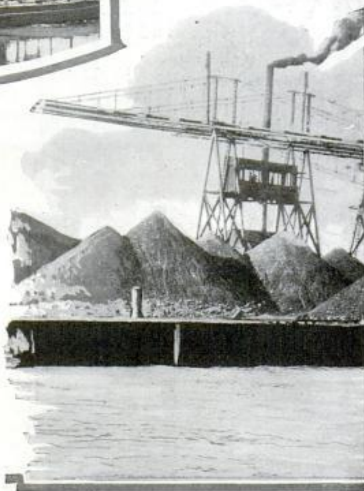
Above, the First "Fast Plant," Introduced with a New Type of Boat; the Unloading Buckets Dipped through the Hatches and Brought Up the Ore; Right, One of the Unloading Bridges Which Went Out When the Lake-Type Steamship with Its Huge Hatchways Came In
