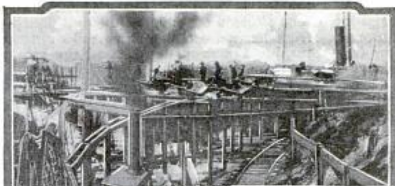
Previous to 1880, Donkey Engines Hoisted the Ore and Men Carted It to the Storage Piles in Wheelbarrows
