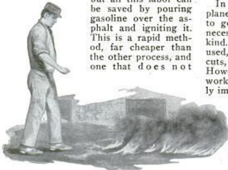
Burning Off Asphalt Coating on Concrete with Gasoline
