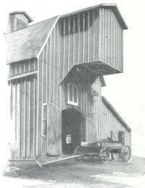
Projecting Gable with Trapdoor on Barn Makes It Easier to Take In Hay
