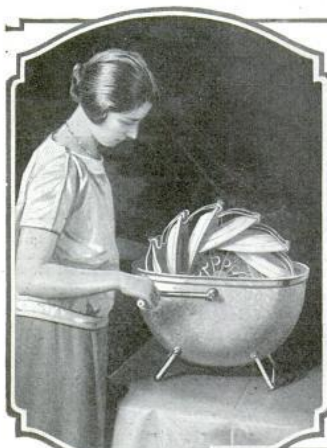
Simple Rotary Dishwasher That Spins the Dirty Plates in Boiling Soap and Water
