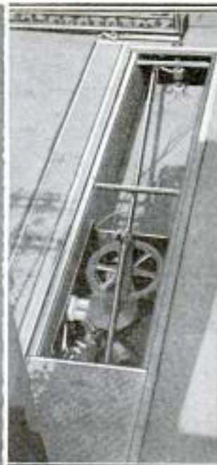
Gates Opening as Release Is Unlocked at Entrance to Grounds, and View of Motor Mechanism Showing How It Is Geared to the Gate Support
