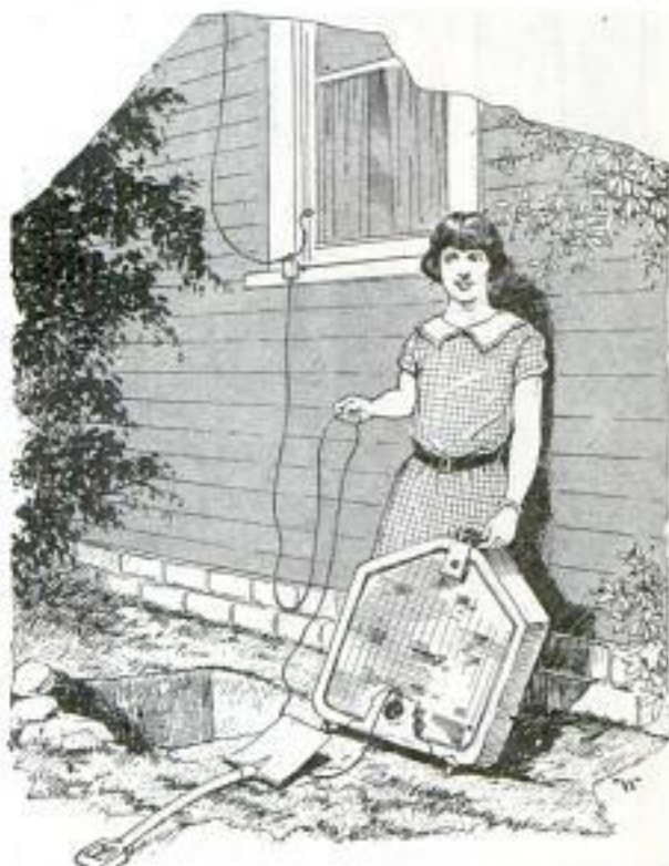
Worn-Out Automobile Radiator Buried in Yard Makes Good Radio Ground
