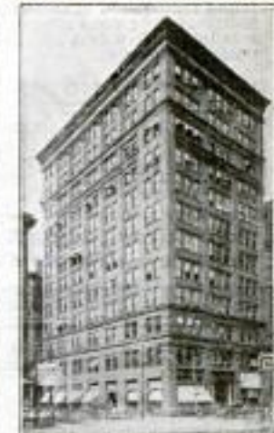
Our Pittsburgh Office Suite 514 Empire Building
