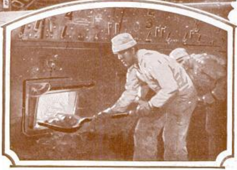
Above, Repairing a Target after Big-Gun Practice at Sea; Two Direct Hits Have Been Made in the Canvas Sheet, Towed Miles Away behind Another Ship; at Right, a Scene in the Fire Room; the Middies Get the Older Coal-Burning Battleships for Their Summer Training Instead of the More Modern Oil Burners and Learn How Hot a Fire Room Can Get
