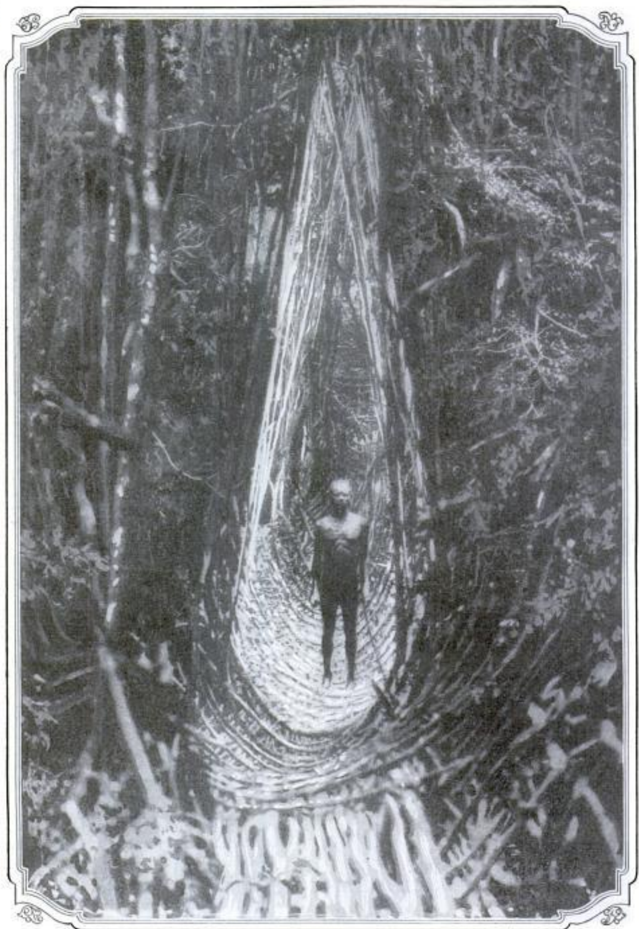
Suspension-Bridge Building in the Heart of the Congo; a Native Workman Building a Roadway High above the Impenetrable Jungle, Following the Monkey Route through the Trees
