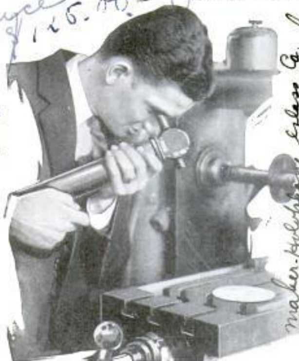
Using Meter Which Eliminates All Guessing as to Amount of Light Reaching Worker's Bench
