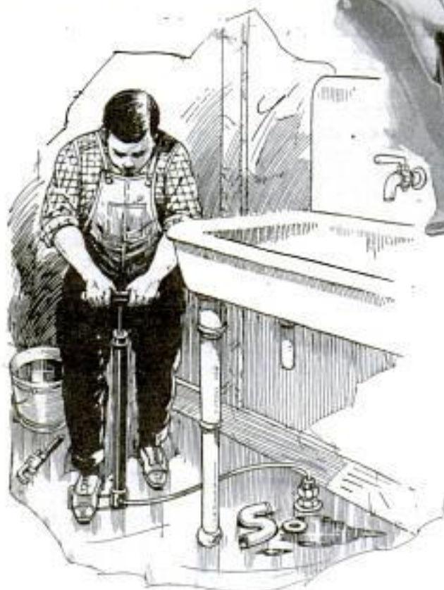
A Force Pump Made from an Automobile Tire Pump Which Will Remove Obsolete Obstructions from the Drain Pipe
