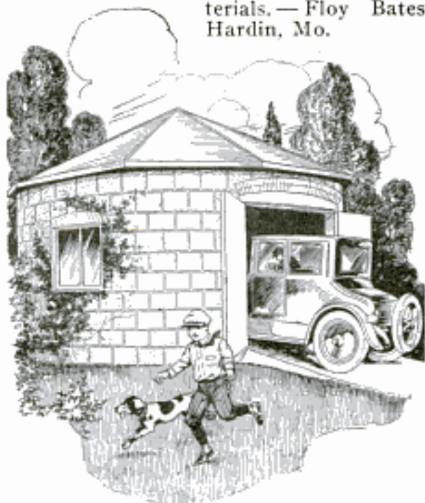
Novel Circular Garage on Farm Is Built from Silo Blocks
