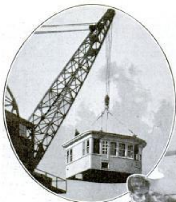
Pilot House Being Lifted Aboard after Its Erection on Land
