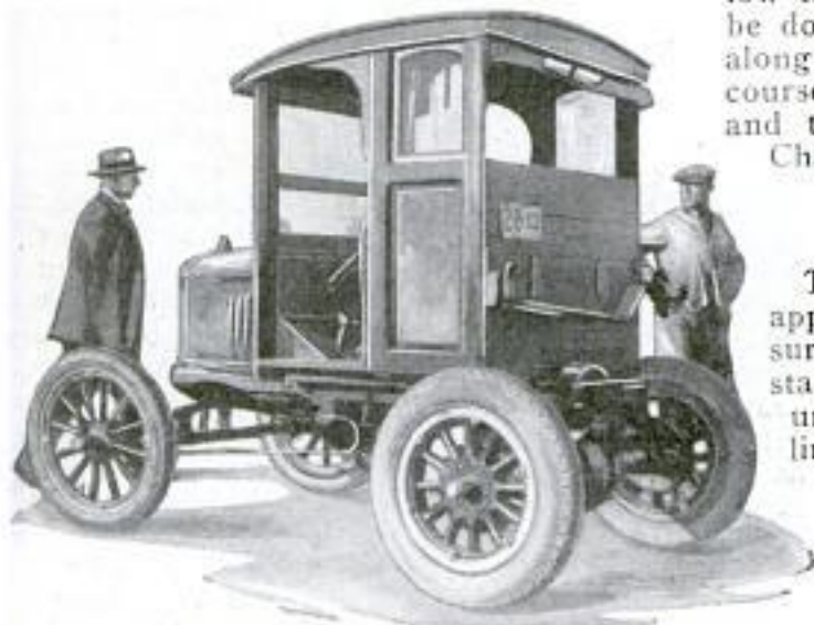
Truck with Shortened Driveshaft Makes Sharp Turns on Piers
