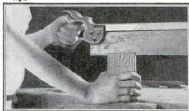
Fig. 2, Ripping an End Rabbet; Fig. 4, Cutting Out Waste Wood in Rabbet
