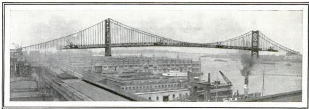
Swinging the Roadway into Place for the New Suspension Bridge Which Is to Link up Philadelphia with Camden, N. J., the Latest of the Great Bridges of the United States
