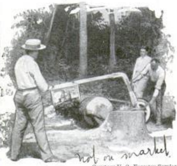
not on market. Courtesy U. S. Forestry Service After Felling Tree, Chain Saw Is Used to Cut the Log into Sections
