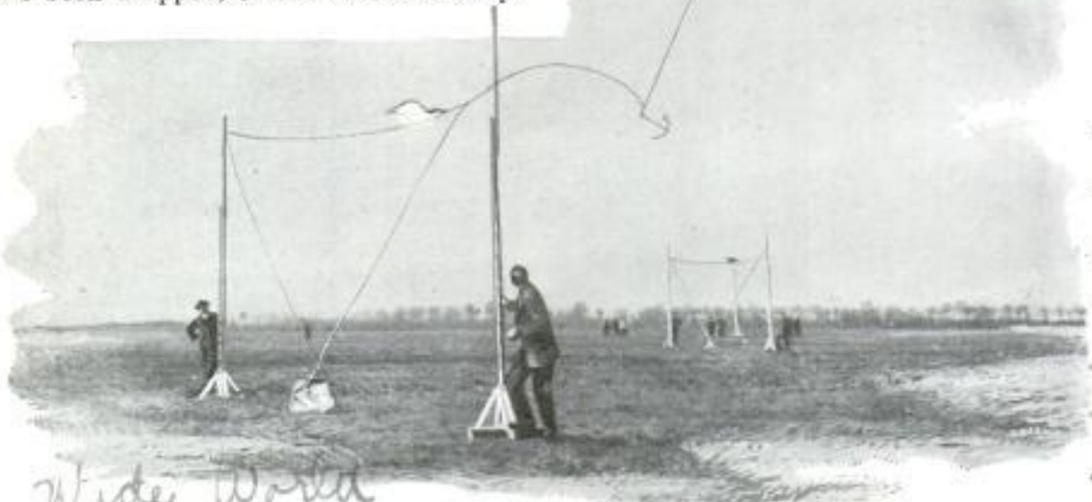
Airplane Snatching Mail Bag from Ground While in Flight: Pilot Steers Low, Drops Anchor and as Airplane Passes between Poles, It Catches Rope Tied to Sack
