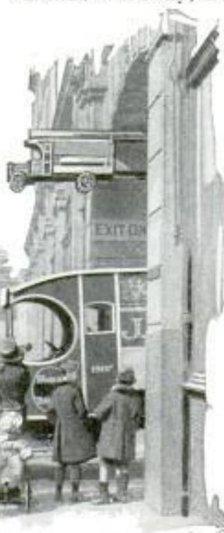
Courtesy L. Lyons & Co., Ltd. Little Pilot Auto on Overhead Track Rolls Out as Cars Emerge from Passageway
