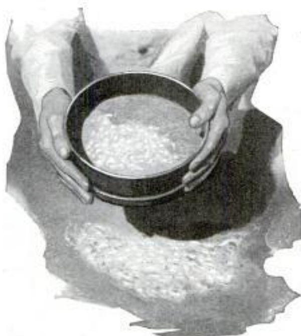
Sifting Cement through Wire Sieve Finer than Silk, Is a Government Requirement
