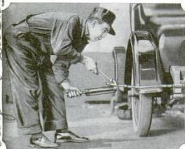
Lever "Booster" on Grease Gun to Increase Force and Save Work in Lubricating Car
