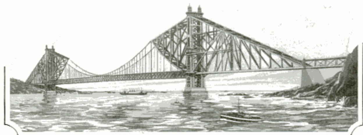
Proposed Bridge Across the Golden Gate at San Francisco, Combining Cantilever Sections at Either End with a 4,000-Foot Suspension Bridge above the Pacific
