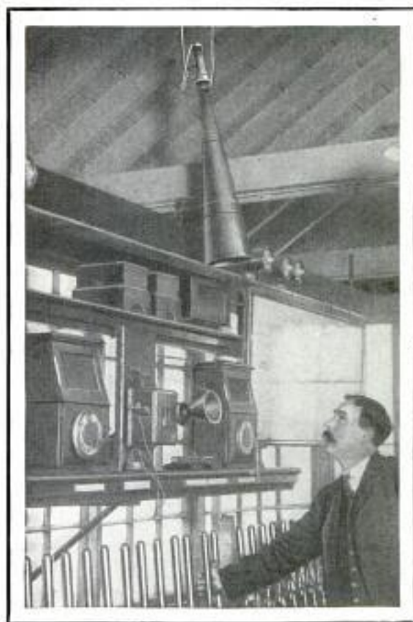
Loud Speaker in Switch House Amplifies Telephone Conversation
