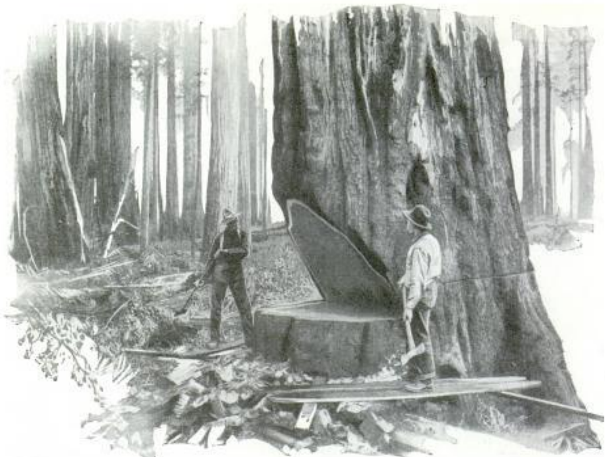
Felling a Giant Possibly Seven Centuries Old; Tree Is Sawed in Half on Side Opposite to That on Which It Is to Fall and Then Chopped Down
