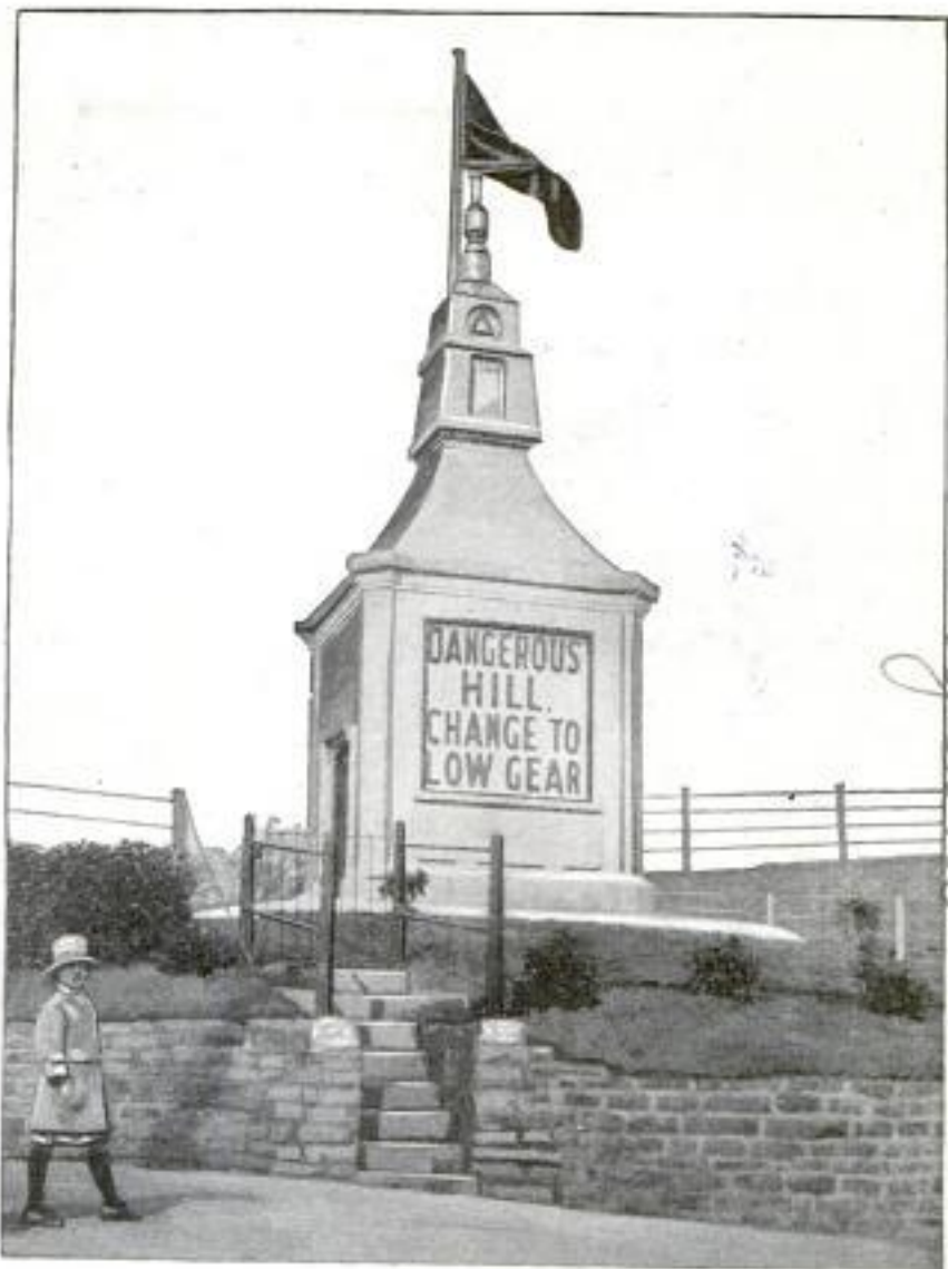
Flag, Beacon and Big Sign on This Conspicuous Lighthouse, Give English Motorists Ample Warning of Dangerous Hill
