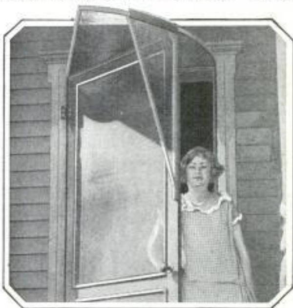
Attachment on Screendoor Prevents Flies from Getting into Kitchen
