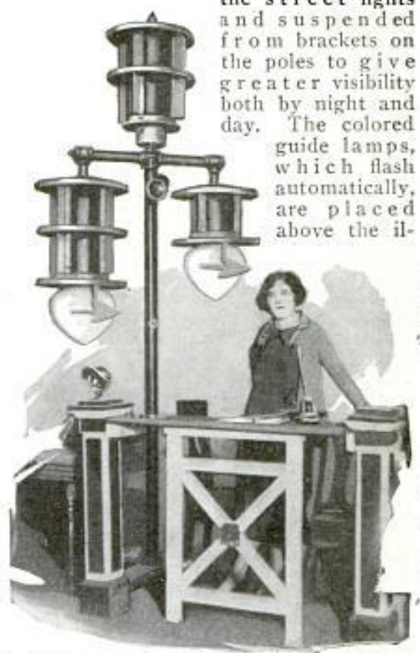
Sample Arrangement of Combined Street and Traffic Lights with Direction Arrows and Colored Lanterns
