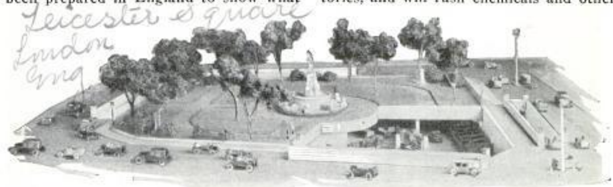
Model with Section Cut Out of Top, Illustrating How Autos Could Be Parked beneath City Square to Relieve Street Congestion; Entrance Is Seen at Right
