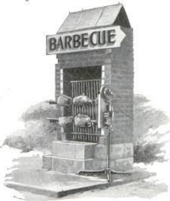
Meat on Spits That Are Revolved by Electric Motor at Proper Speed for Roasting
