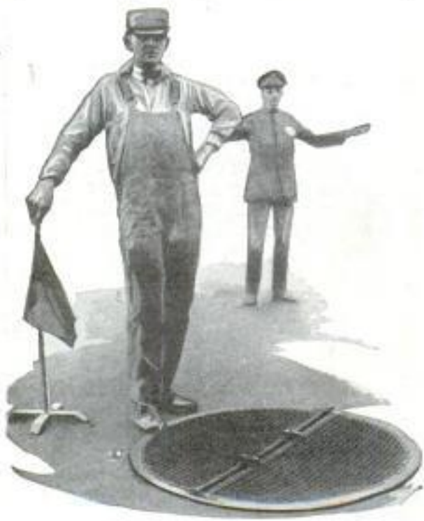
Folding Screen Cover for Manholes That Guards Autos and Workmen Inside as Well
