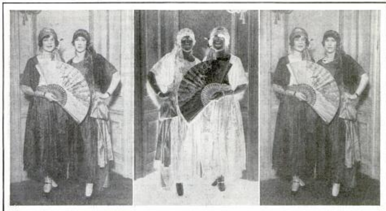
Left, Unretouched Copy of an Original Picture; Center, the Negative Print of the Positive Film Transmitted, and, Right, the Telephoto Picture as Received
