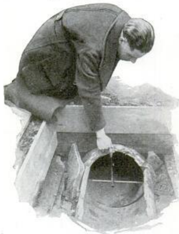
End of Underground Radio Antenna Which Carried Signals from Maryland to Los Angeles
