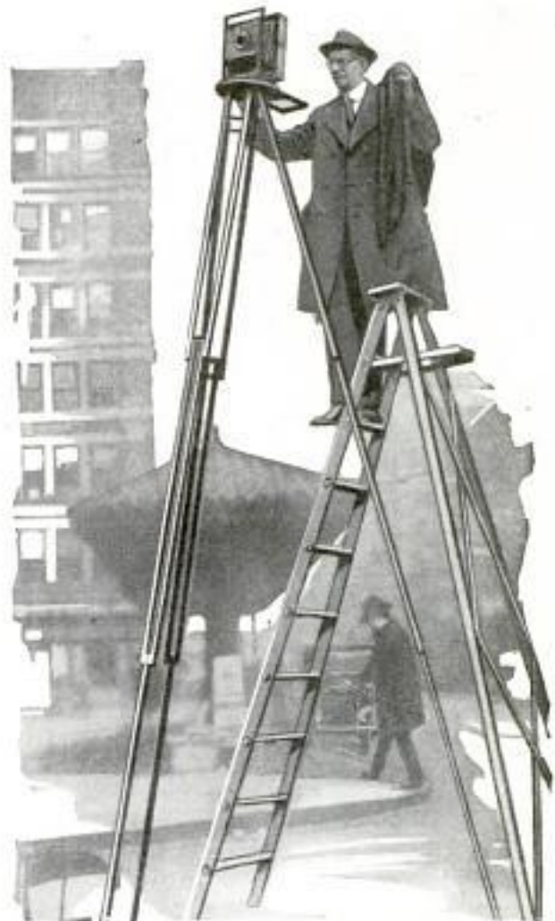
Lofty Photographers' Tripod Which Elevates Camera above Obstructions When Taking Pictures
