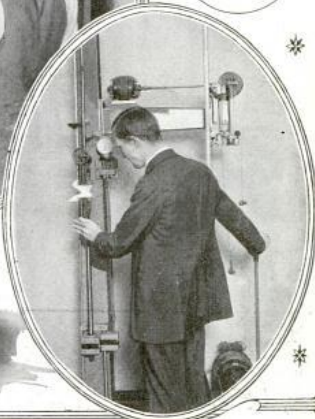
Where the Standards of Cotton Fabrics Are Set by Textile Experts of the Agricultural Bureau, Who Keep an Accurate Record of Their Findings; Left, Registering the Pull Required to Break a Strand of Cotton Fiber; Below, Left, Instrument That Tests the Twist of Wool and Cotton Threads, and Right, Determining the Resistance of Sheets to Rips and Tears
