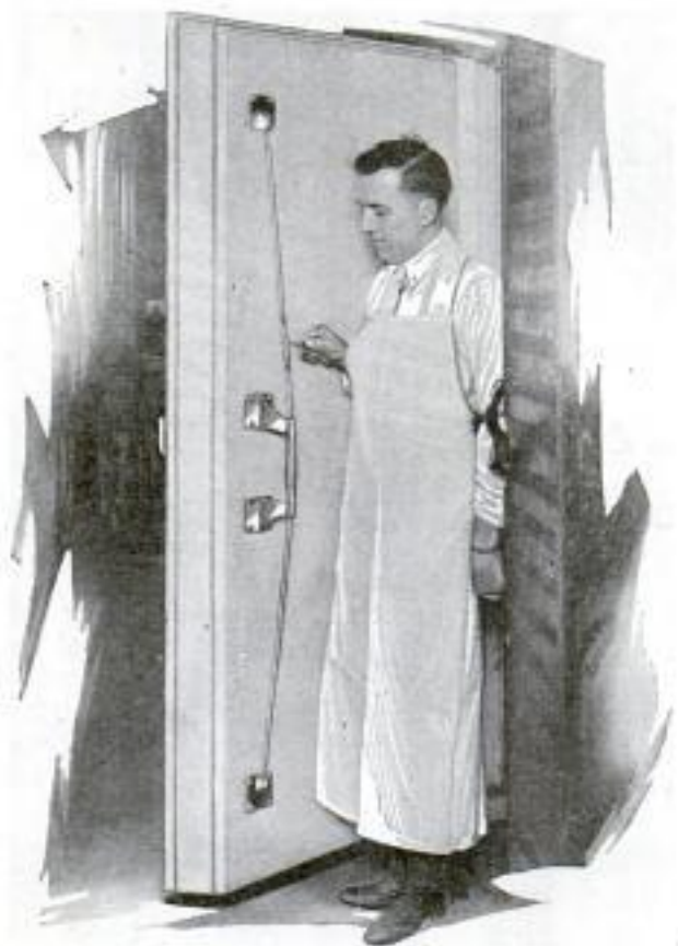
Truss Rod in Place; Man Is Pointing to Sleeve for Tightening or Loosening It
