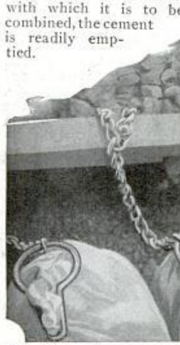
How Self-Emptying Cement Sacks Are Fastened to Truck; Above, Load Ready for Dumping
