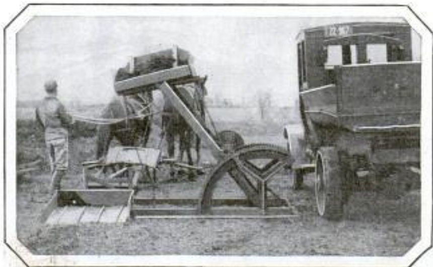
With This Rig, the Team Dumps the Scraper Load and Empties It into the Truck in One Continuous Operation
