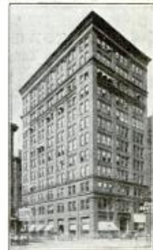
Our Pittsburgh Office Suite 514 Empire Building
