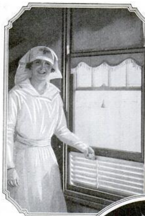
For the Sick-Room or Any Window in the House, This Adjustable Ventilator Allows Fresh Air to Enter without a Draft, Keeps Rain from Floors and Prevents Children from Falling Out
