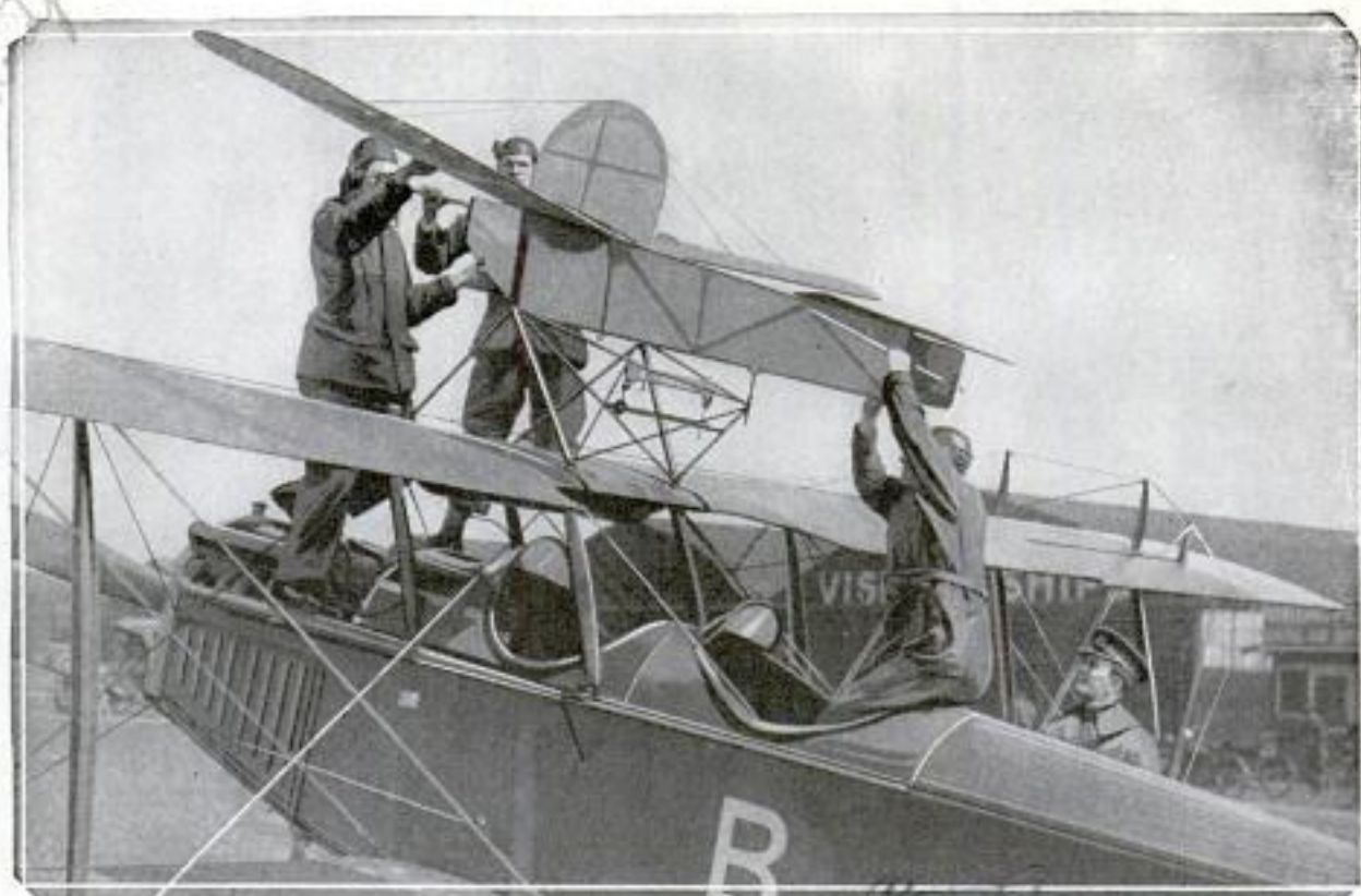
Adjusting the Model Glider Plane to Its Rigging, from Which It Was Released as a Target for Anti-Aircraft Guns to Test the Efficiency of the Marksmen and Ordnance
