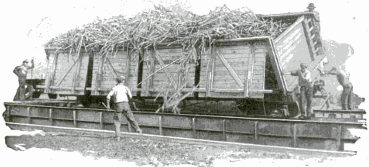
Specially Designed Cars, Emptied by One Operation of a Dumping Tipple, Facilitate the Hauling of the Newly Harvested Sugar Cane from the Field to the Mills
