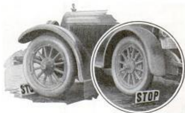
Rubber Traffic Sign Installed in Street Paving
