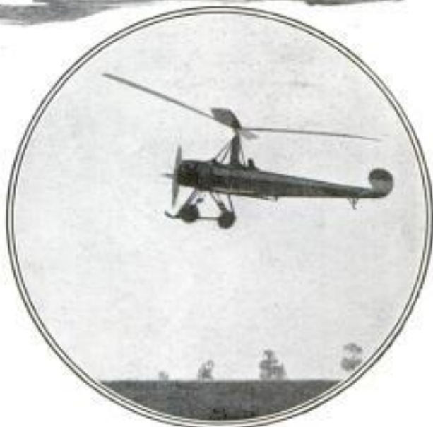
Four Freely Revolving Wings Replace the Usual Upper Surfaces in This Rebuilt Training Biplane
