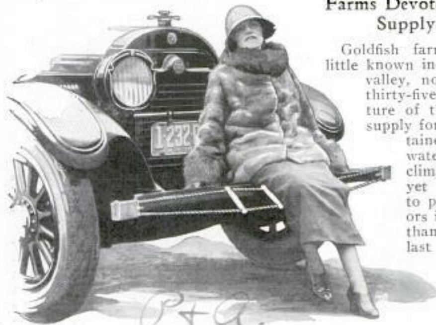
Auto Bumper That Keeps Persons from Falling under Wheels and Also Cuts Off Ignition and Applies Brakes
