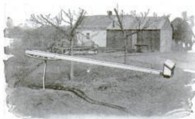
Revolving Mail-Box Support Eliminates Need of Crossing Muddy Ditch to Get Mail
