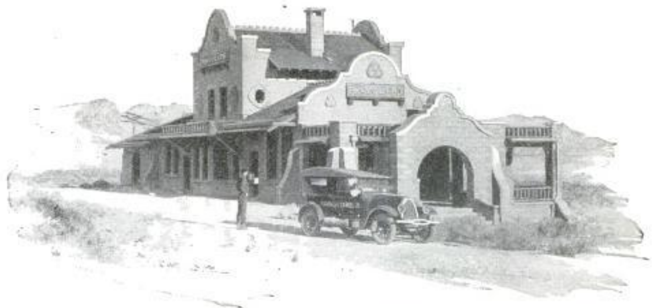
Left to the Whims of Time and Weather, the Railroad Station That Welcomed the Hopeful Stranger Registers a Mute Record of Blasted Ambitions and Wrecked Fortunes
