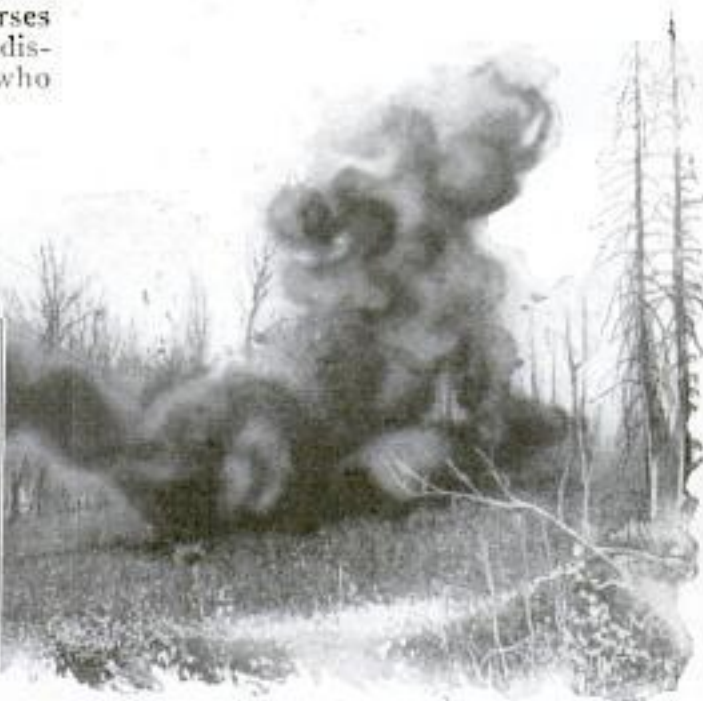
Blast of Salvaged War Explosive That Uprooted Group of Stumps; Left, One of the Powerful Artillery Tractors Going into Action to Aid in Breaking Down Underbrush
