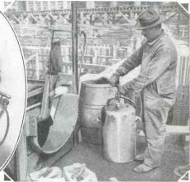
Portable Heater for Thawing Pipes, and Outfit Attached to Concrete Mixture with Flame Directed inside Drum
