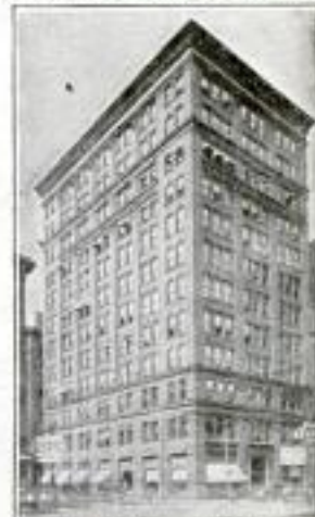
Our Pittsburgh Office Suite 514 Empire Building
