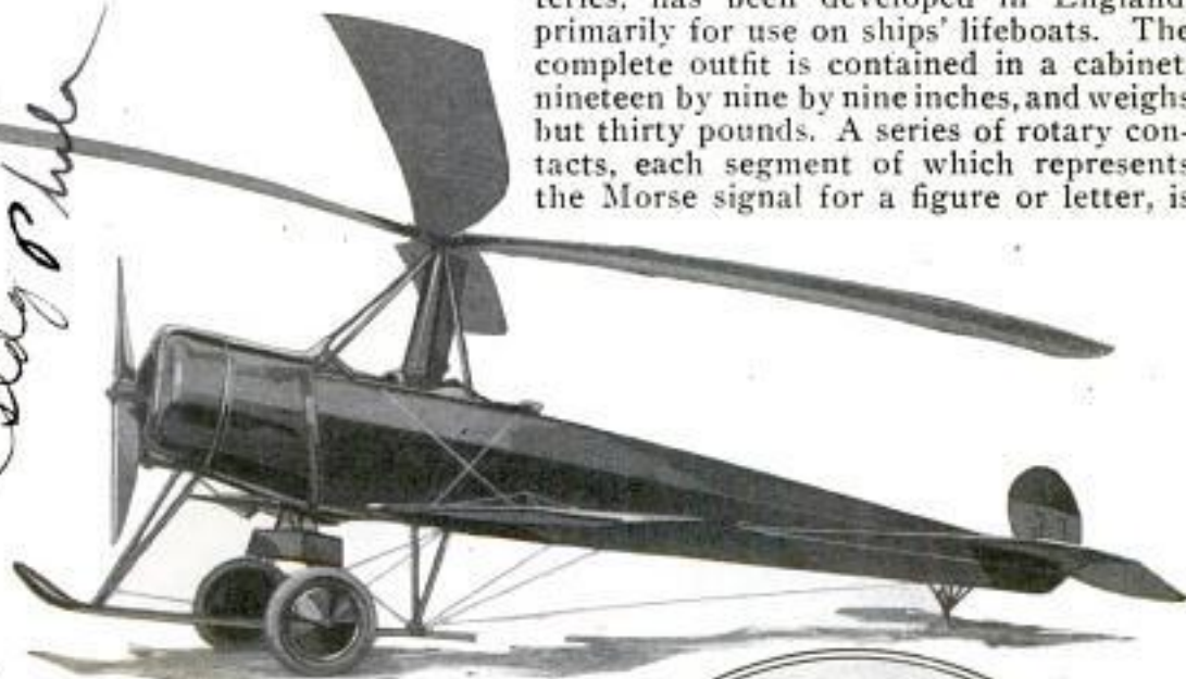
Four Freely Revolving Wings Replace the Usual Upper Surfaces in This Rebuilt Training Biplane
