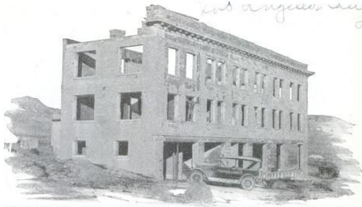
Empty Shell of What Was Once an Imposing Bank, the Abandoned "Ghost" City's Center of Finance during a Brief Heyday of Industrial Clamor and Commercial Boom
