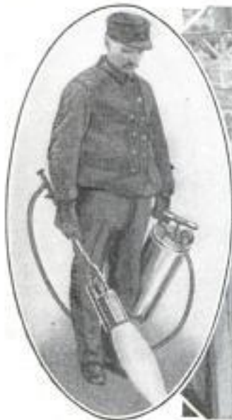
Portable Heater for Thawing Pipes, and Outfit Attached to Concrete Mixture with Flame Directed inside Drum
