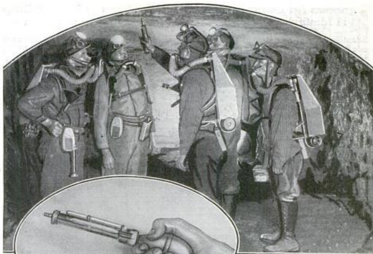
Miners Using the Gas Detector on Roof of Gallery, and Close View of Apparatus Showing the Bulb and Tubes
