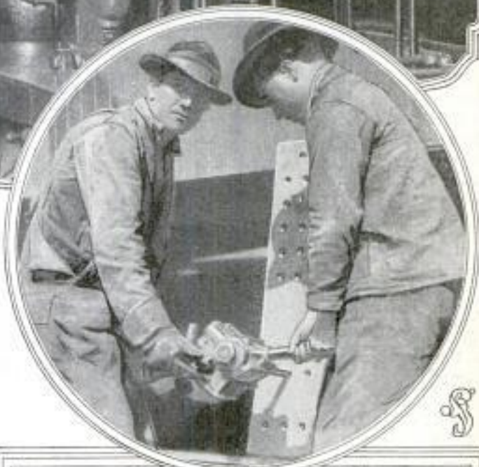
Hunting for Defects in Triple Air-Brake Valve in Testing Rack, and at Right, Cutting Holes in Metal Bar with Air-Motor Drill
