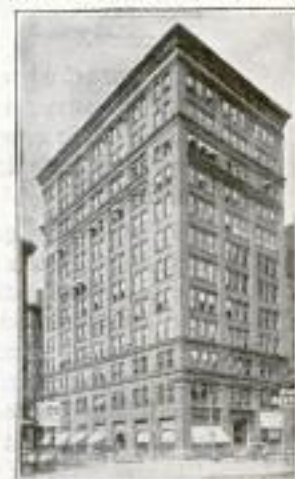
Our Pittsburgh Office Suite 514 Empire Building
