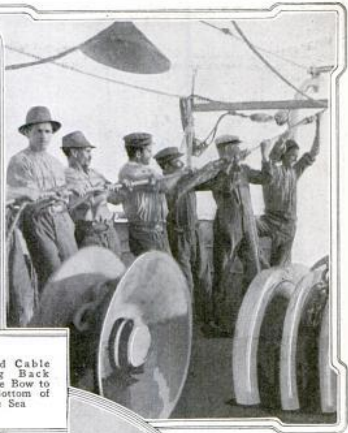
Crew Lowering the Grapple Hook over the Bow to Drag for the Submarine Cable, Which Must Be Lifted and Tested Until the Defective Spot Is Located
