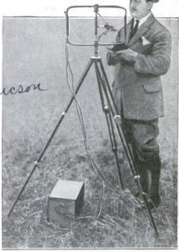
Radio Prospector Seeking Ore with Tripod and Loop Aerial
