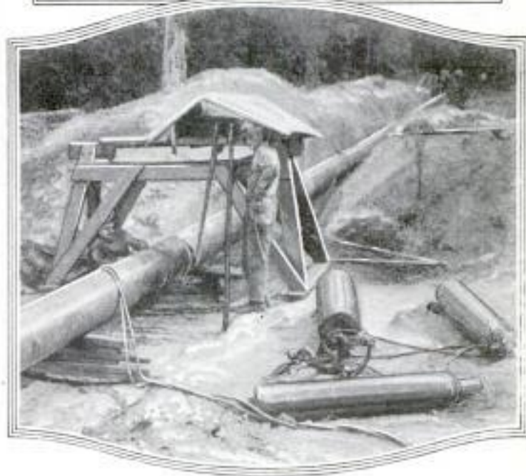
The End of the Line, Above, Showing a Refinery from the Air; the Helper, Left, Holds the Sunshade While the Welder Works on a Pipe Blocked Up to Cross a Gully; Below, Finishing the "Tie-In" of Completed Sections
