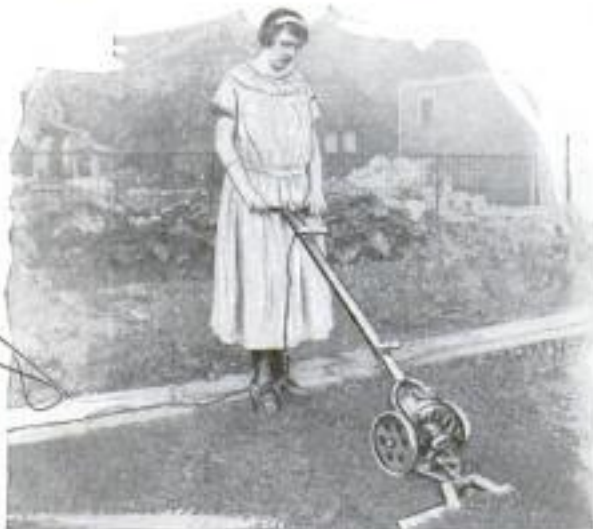
Lawn Clipper in Operation; the Motor, with Cord Attached, Moving Cutting Blades in Front
