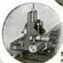
Threading Pipe Union
