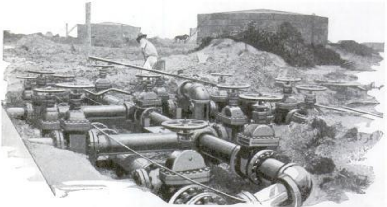
Some of the Valves through Which the Oil Is Routed to Fill the Various Tanks That Dot the Great Storage Fields Surrounding Every Refinery
