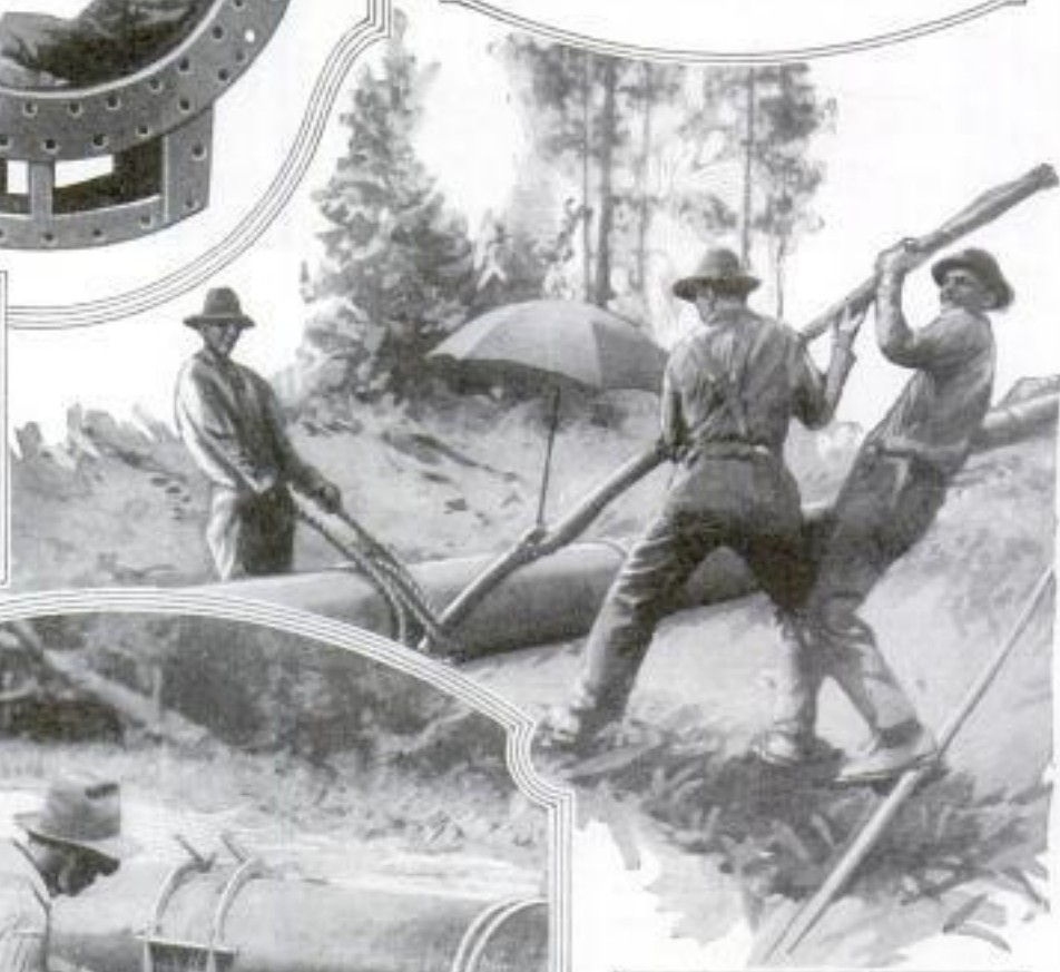
In Some Soils the Pipe Is Covered with Asbestos Paper or Coated with Tar to Resist Corrosion
