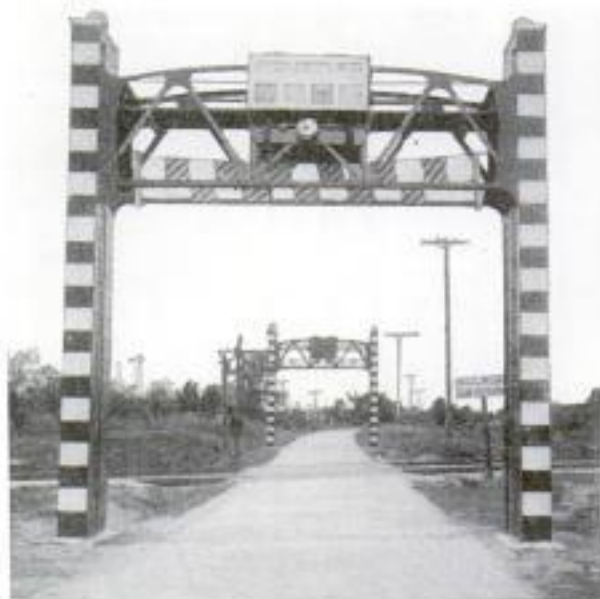
Safety Gate at Highway Railroad Crossing Which Drops as Approaching Train Enters Electric Circuit
