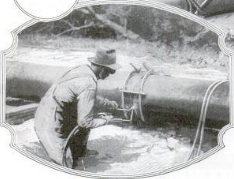
The Steam Cylinder of an Oil-Pipe Pump (Above) Is an Enormous Thing; at the Right, Workmen Alining the Pipe for the Welders
