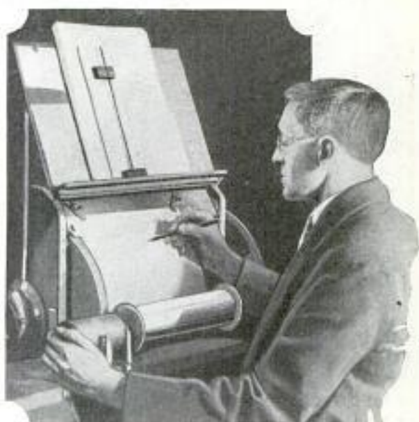
At Work on Master Player-Piano Record with Musical Score as Copy Guide
