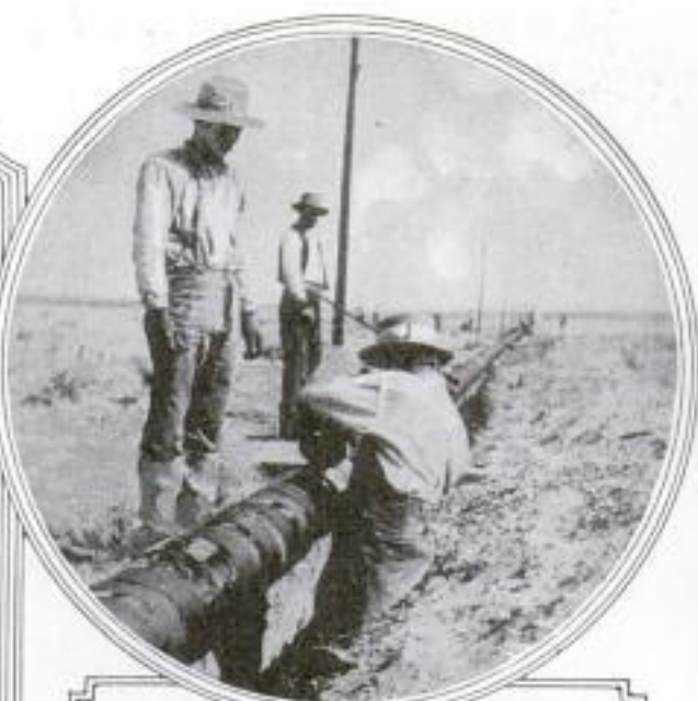
In Some Soils the Pipe Is Covered with Asbestos Paper or Coated with Tar to Resist Corrosion
