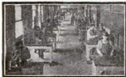
Electrical Experts $175 Month and Up
