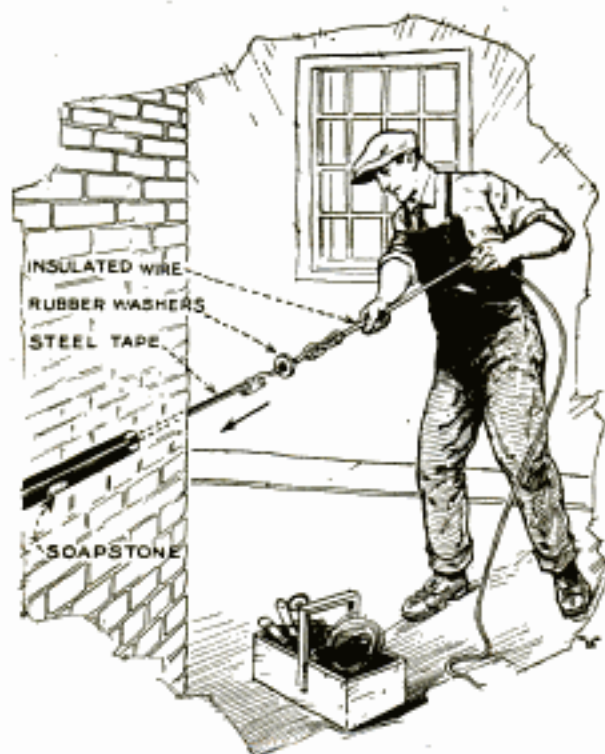
Simple Method of Dusting Soapstone in Conduit to Prevent Wires from Sticking
