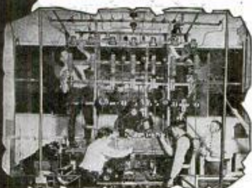
Students Doing Actual Work On Power Transmission Apparatus
