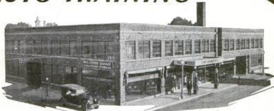
Here's Dulyea and Vander Bie's Garage and Salesroom
