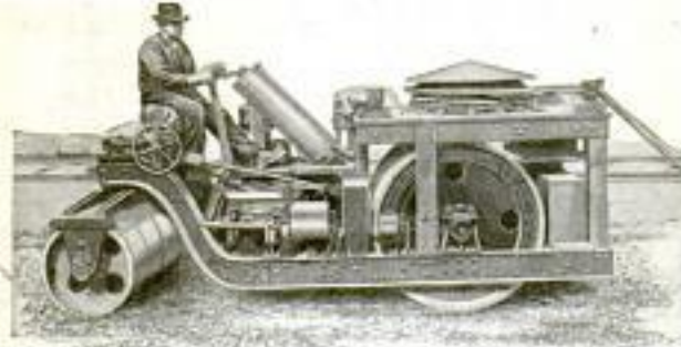
Supplied with Power from Near-By Trolley, Electrified Road Roller as It Appeared Remodeled
