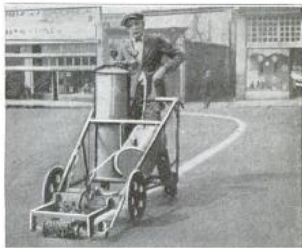
Painting Traffic Guide Line with Marker Truck
