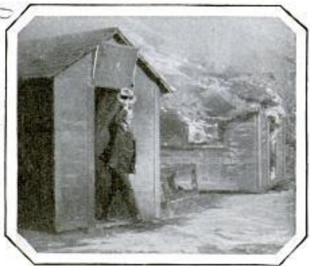
Leaving Building Painted with Fireproof Solution After Unsuccessful Attempts Were Made to Burn It
