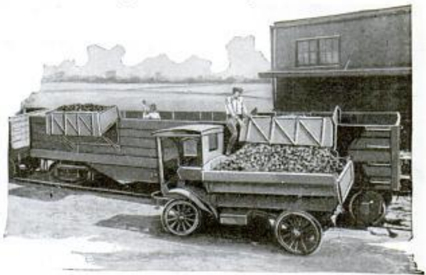
Emptying Loaded Chute into Truck While Shoveler Fills Another Clamped to Side of Car for the Next Driver
