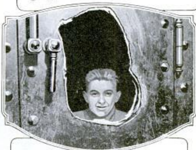
There Is No Explosion to Awake the Neighbors When a Modern Bank Bandit Burns His Way into a Vault with His Noiseless Oxyacetylene Equipment
