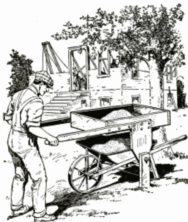
A Fixed Sieve That Hastens the Riddling of Sand on Concrete Work
