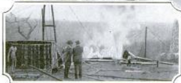
Erecting the Big Steel-Hood Snuffer over Flaming Gas Well to Extinguish the Fire
