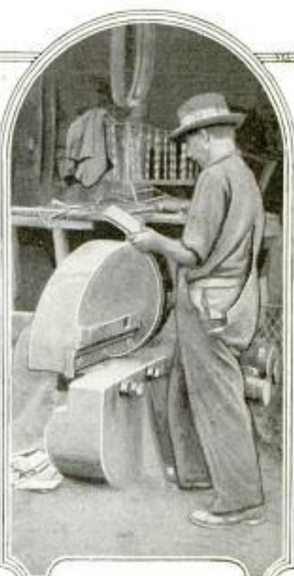
Cutting Up Iron Strips with Power Shears in Junk Shop
