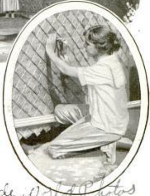
Nailing the Paper Lumber to the Wooden Frame
