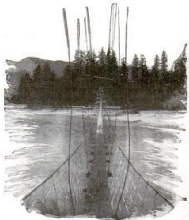
Footbridge Swung between Trees on Banks of River to Give Passage from Waterlocked Farmland
