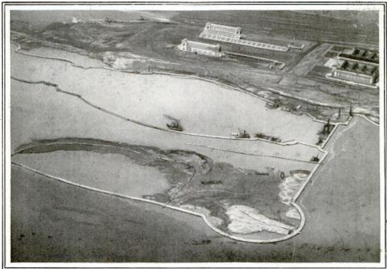
Copyright, Chicago Aerial Survey
