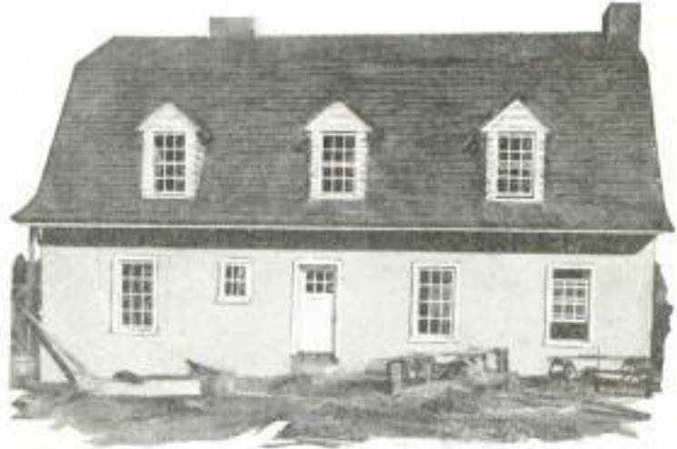
The Walls of This House, Built by a Washington Scientist, Are Made of Rammed Earth at a Great Saving over Concrete, Brick or Wood
