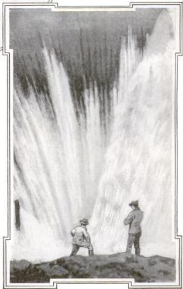
Model to Illustrate Water's Course Flowing into Funnel, and View of Actual Spillway
