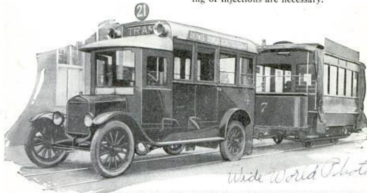
Motor-Bus Street-Car "Train" with Its Trolleyless Passenger Trailer on Track
