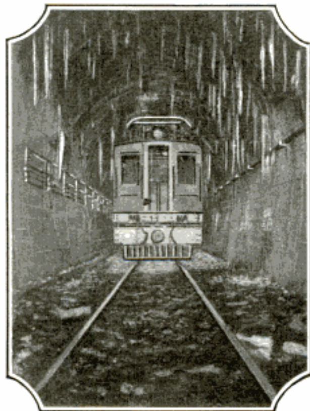
Electric Locomotive in Otira Tunnel Passing under Forest of Icicles Caused by Winter Weather
