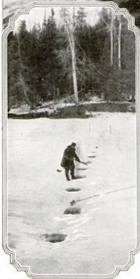
Digging Holes in the Frozen Surface of a Wide River through Which the Measuring Instrument Can Be Lowered to Register the Winter Flow of the Stream
