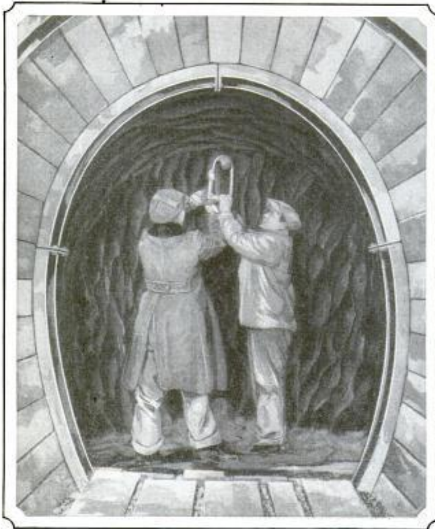
Carving a New Tunnel into the Clay with a Scraping Knife Is Strenuous Work but Overcoats Are Not Uncomfortable
