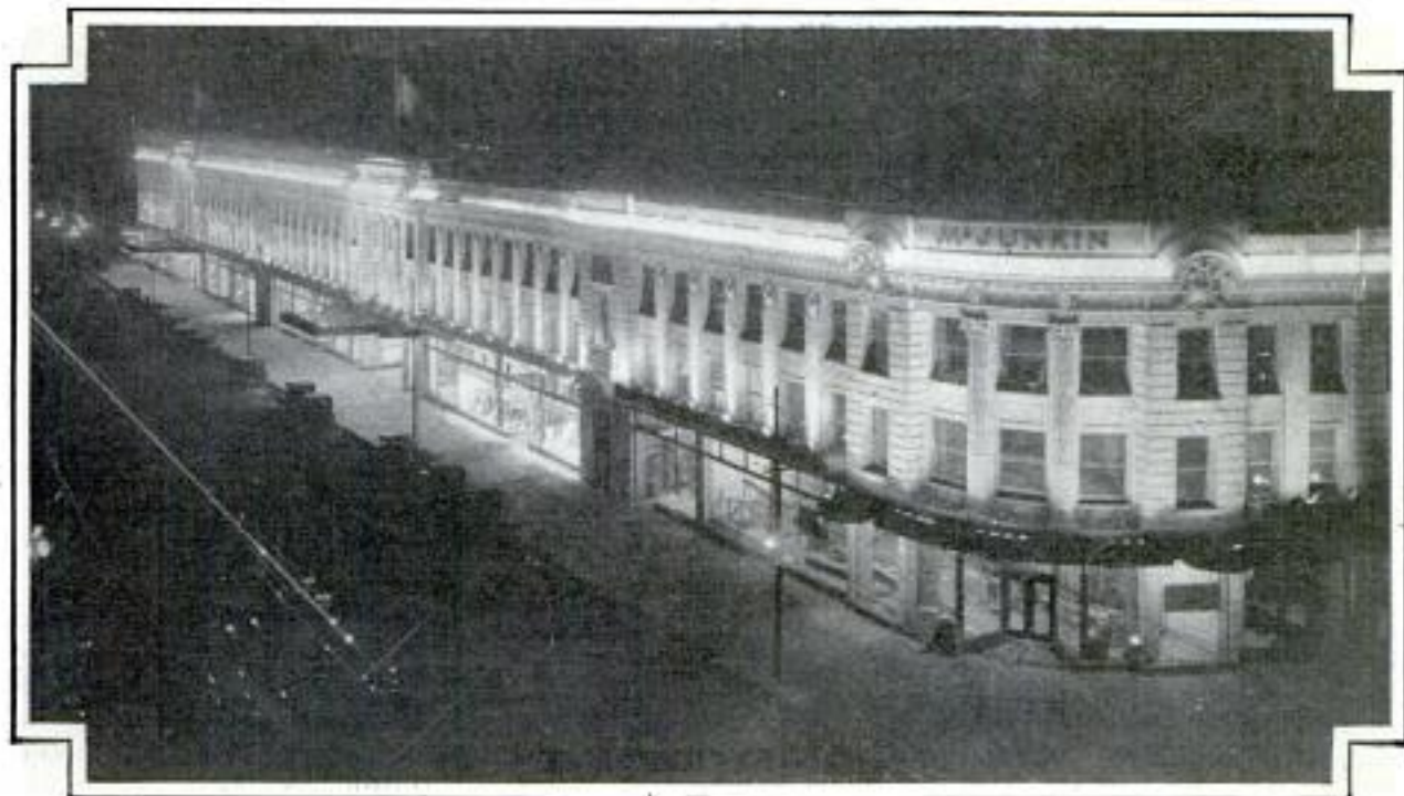
Building Front Illuminated by Floods of Various Colored Lights Hidden under Powerful Reflectors; Shades Change Regularly Every Few Minutes, Bathing the Walls in Different Hues
