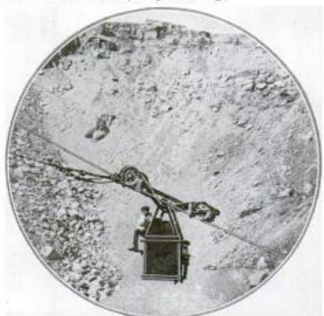
Copyright, Underwood & Underwood Trolley Cage and Its Operator Bound for the Bottom of a Big Working
