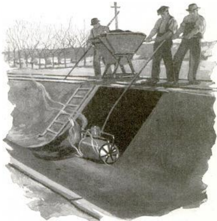
Applying Asphalt Coating to Bed of Irrigation Canal, Using a Heated Roller to Distribute and Compress the Material Evenly over the Surface
