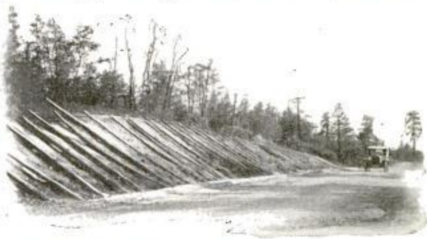
Preventing Sand Drifts on Hard Roads by Means of Poles Laid on the Banks
