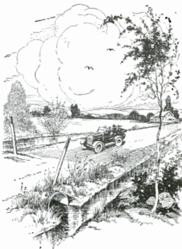
Painted Markers Set at Ends of Road Culverts Protect Passing Motorists from Accidents
