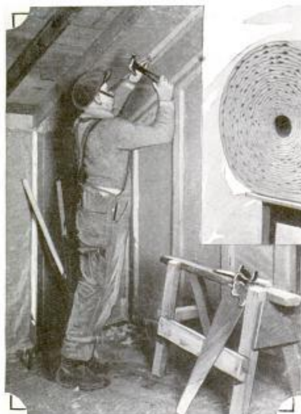
Trying Fireproof Qualities of Wood Wool for Building Walls with Flame of Blowtorch, and Left, Attaching the Sheets Inside of Frame for House to Prevent Entrance of Cold
