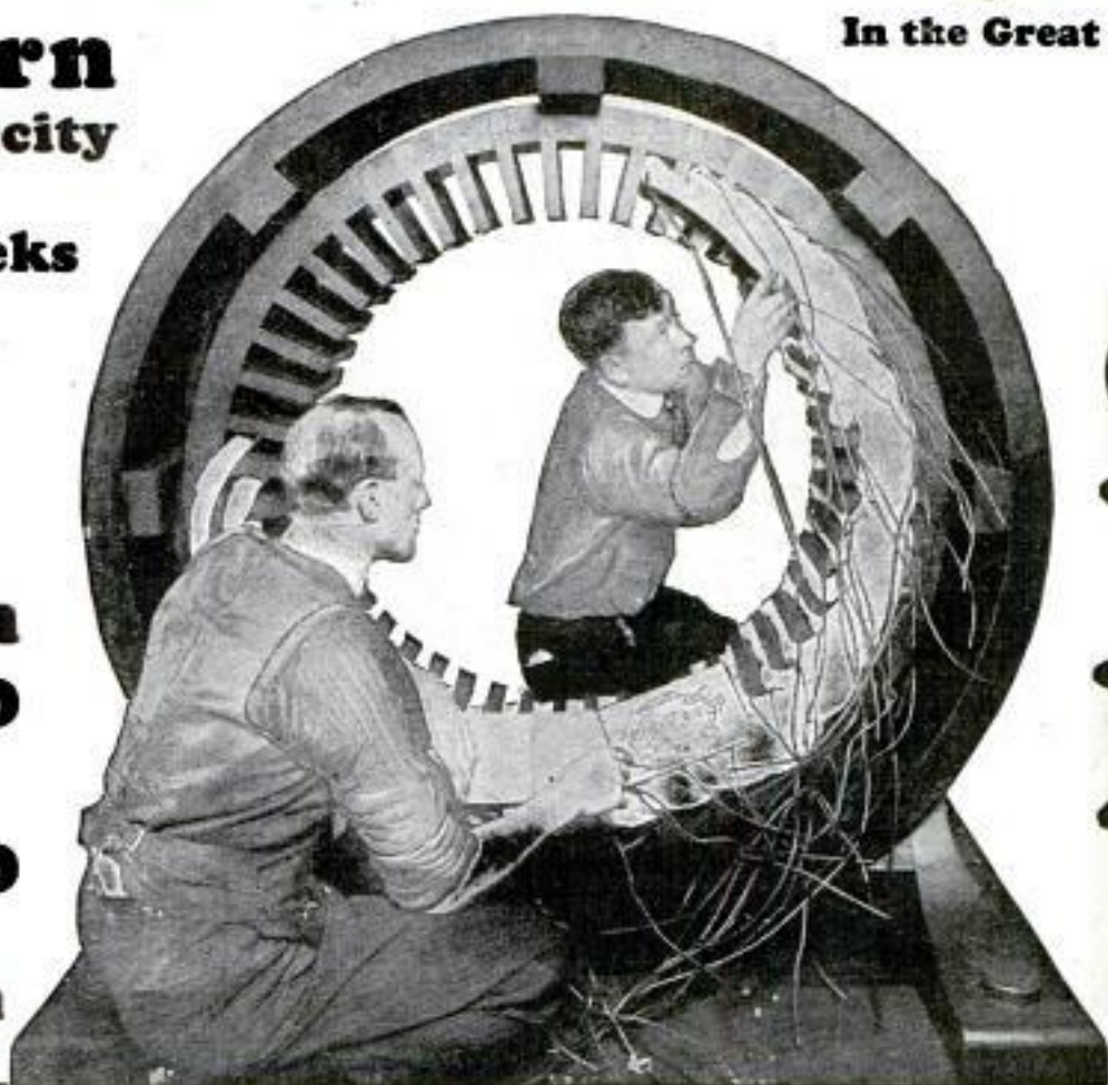
STUDENT WINDING STATOR
