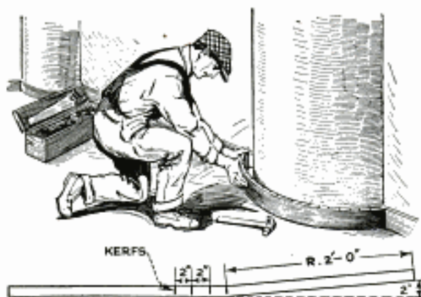
A Simple and Accurate Method of Spacing Kerfs in Work to Be Bent
