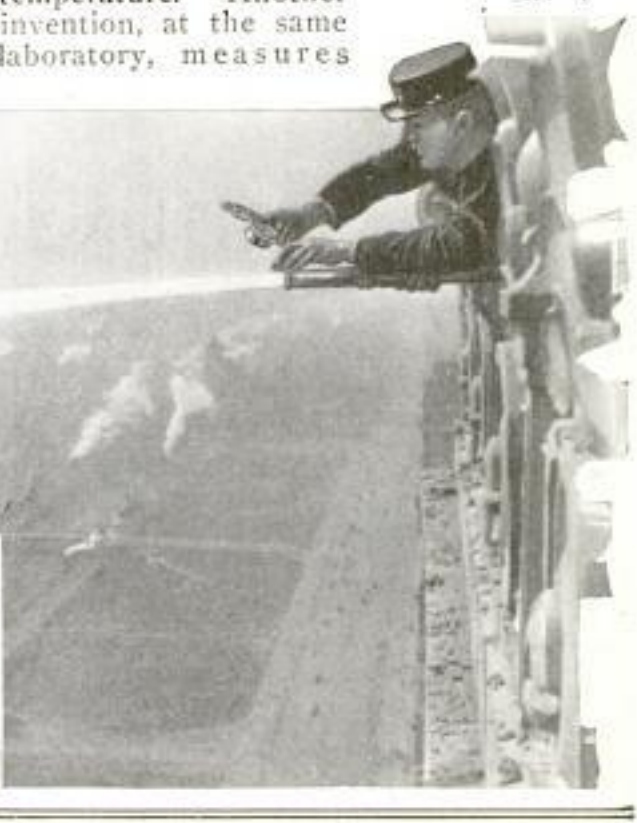
Fireman Measuring Flow of Water from the Nozzle of a Skyscraper's Standpipe System: Left, Arrow Points to Tower Where Hose Outlet Is Installed
