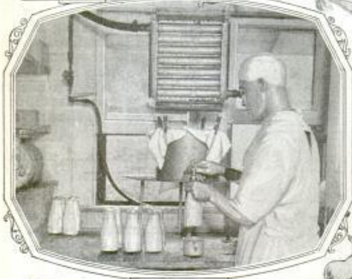
Inside Milk Cooling and Bottling Room Where Pints and Quarts Are Filled for Delivery
