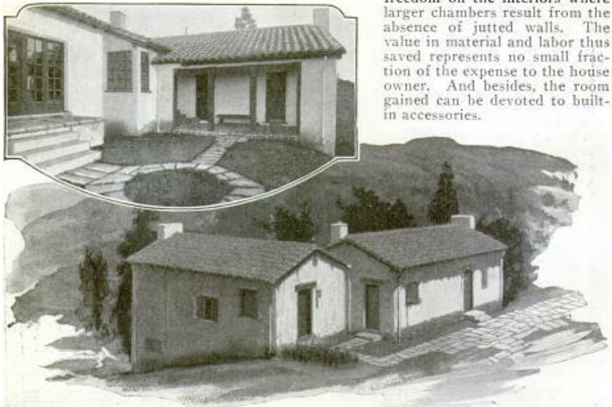
Two Views of a Home of Unusual Mexican Design, Built of Flat, Hollow Tile and Concrete; Resembling Two Buildings, It Has a Large "Patio" and Three Fireplaces
