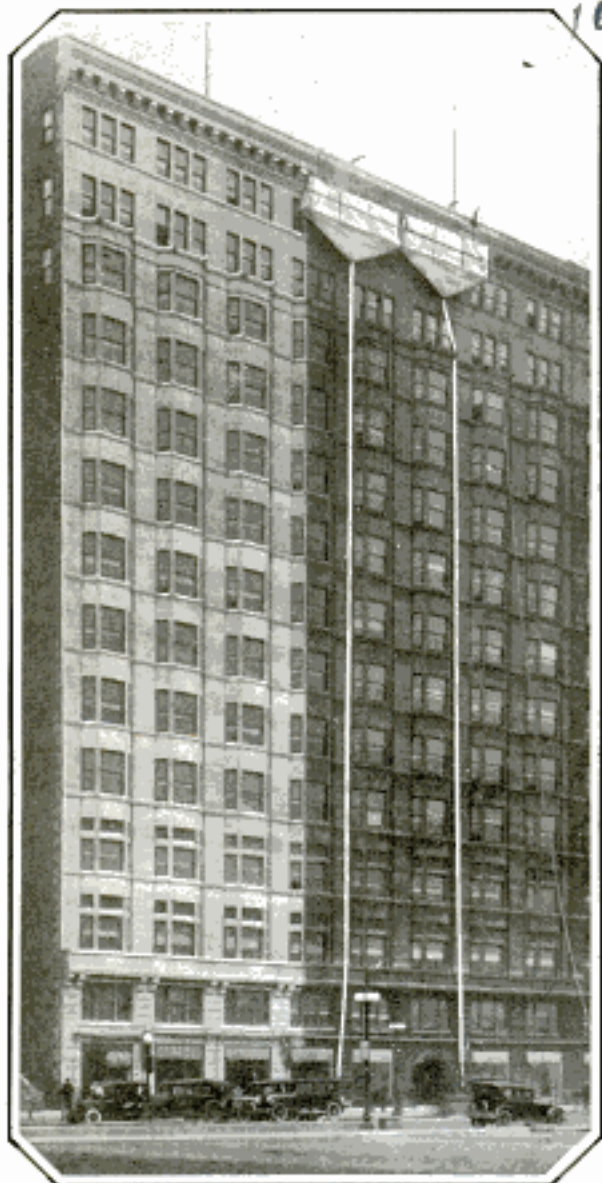
Magic Worked by Sand on Screened Scaffolds: Scoured and Unscoured Sections of Chicago Hotel
