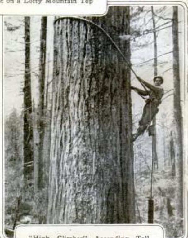
"High Climber" Ascending Tall Spar Tree to Be Trimmed for Support of Aerial Cable
