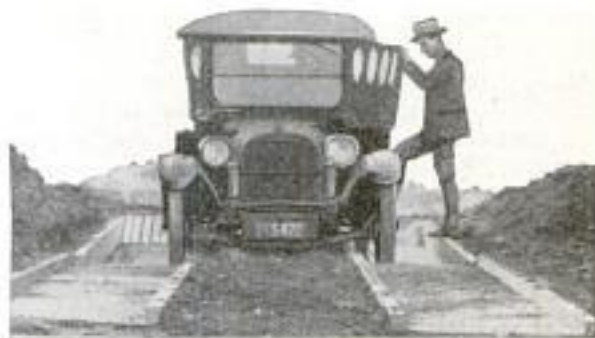
Running a Car through Disinfecting Trough to Kill Germs on Tires and Wheels
