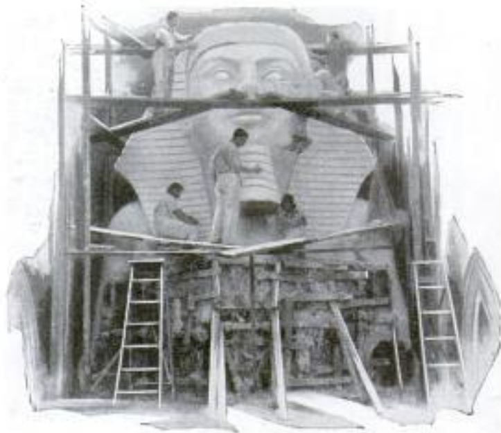
Constructing Huge Plaster Head of Egyptian Statue, Part of Background of Historical Motion-Picture Production
