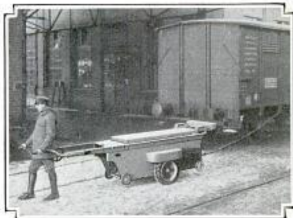
Pulling a Freight Car with Electric Tractor Truck; Spring Bumpers Are for Pushing
