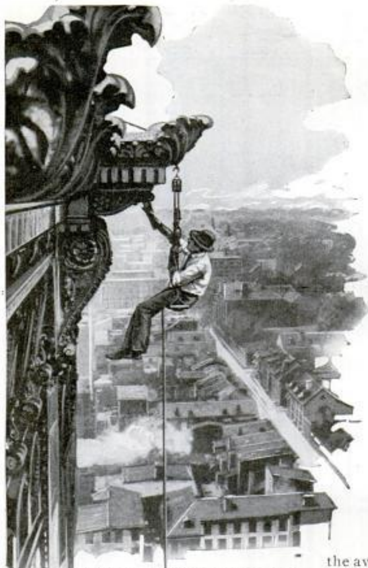
Where the "Bos'n's Chair" Affords Comfortable Support for Dauntless Worker Hung in Midair High over Busy City Streets
