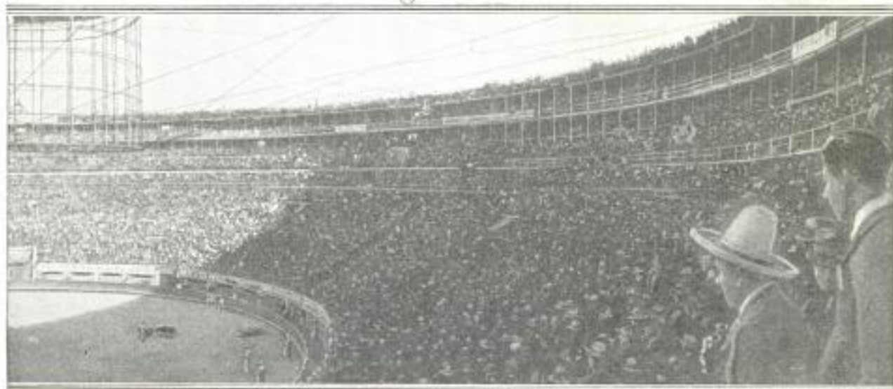
With an Arena 450 Feet in Diameter and Seating Stands of Concrete and Steel, Mexico's Most Prominent Outdoor Amusement Structure Affords Room for 20,000 Spectators
