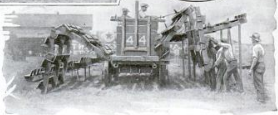
Unloading the Bleachers Takes Crew but a Few Moments and Wagon Remains as Additional Support; Upper Pictures Show Section Extended and Packed
