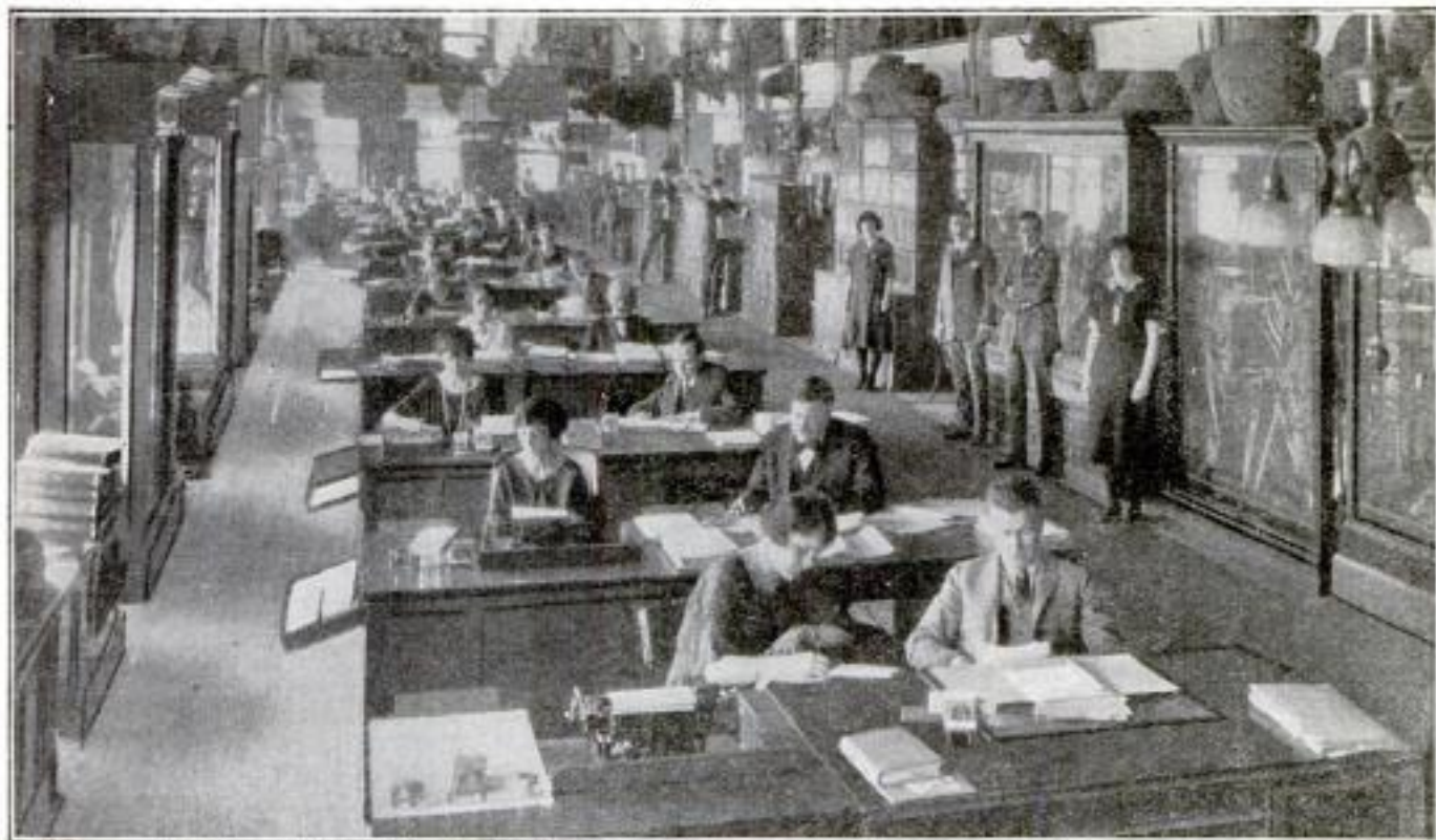
MAIN OFFICE, VICTOR J. EVANS & CO.—VICTOR BUILDING, WASHINGTON, D. C.
