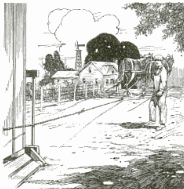
Iron Pipe Arranged Vertically Along Corner of Building Protects It from Hoisting Rope
