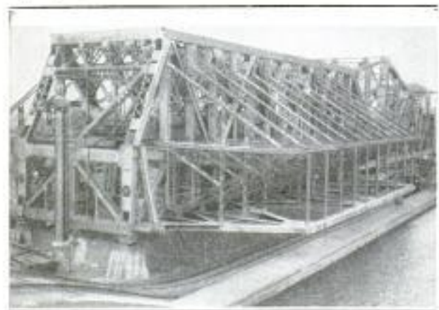
Movable Dam on Panama Canal that Bars Off Channel in Cases of Emergencies
