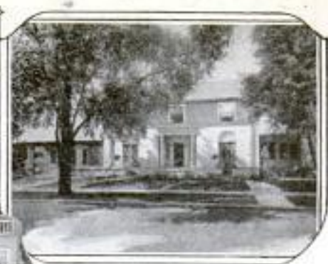
Attractive, but Inexpensive, Home with Double Walls of Concrete Blocks Which Serve to Keep It Cool in Summer and Warm in Winter
