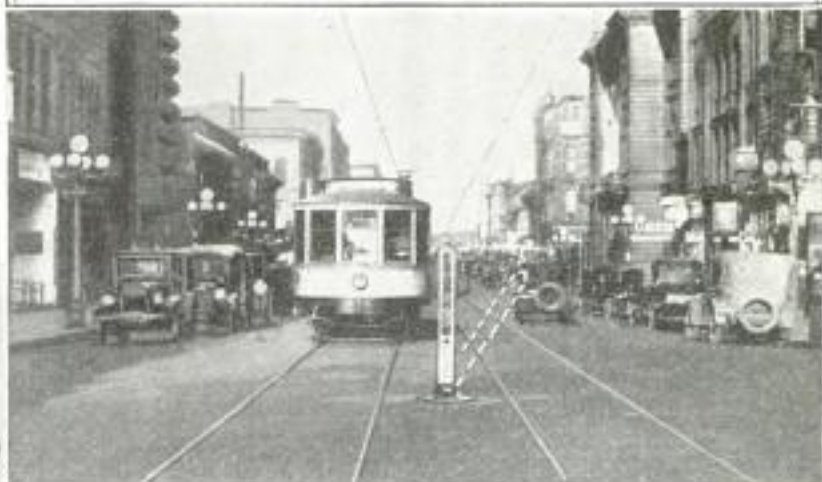
Two Styles of Tilting Traffic Sign Post Resting on Ball Support and One in Position in Street; Dotted Lines Indicate How It Would Swing if Struck
